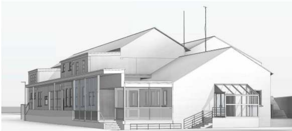
Existing View from South East
