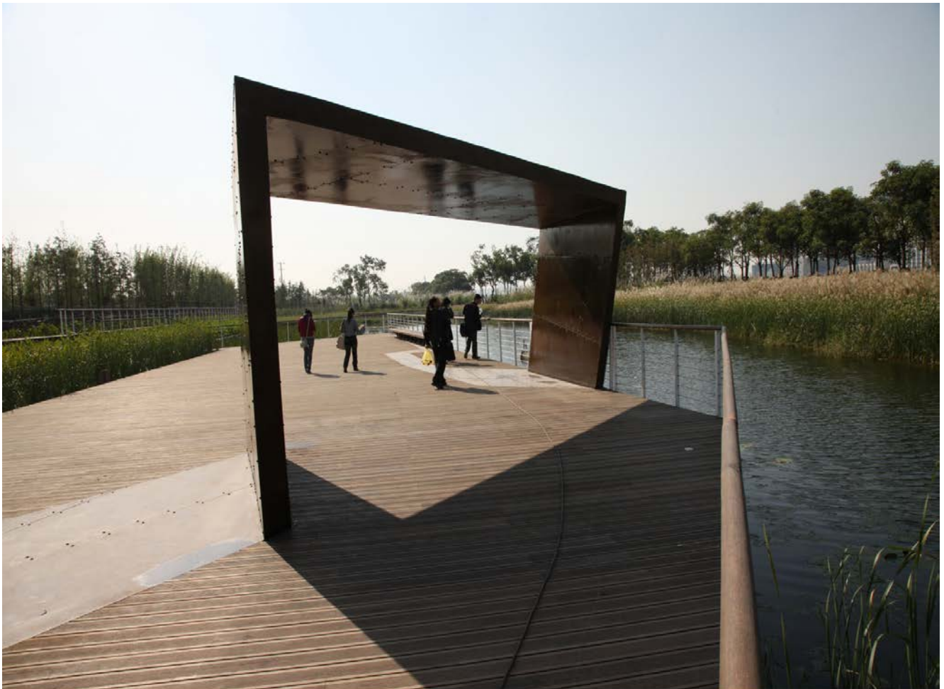
14 The steel arbor in the wetland is composed of recycled steel panels from the site, which provides shade, shelter, frames views, and shapes spaces.
