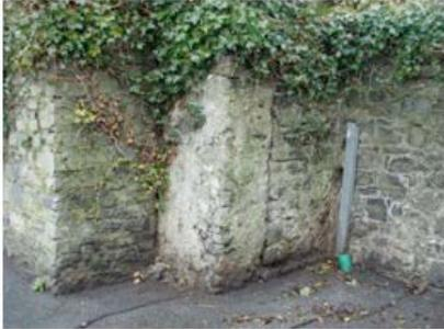
Plate 19. Untied walls at boundary at millrace.
