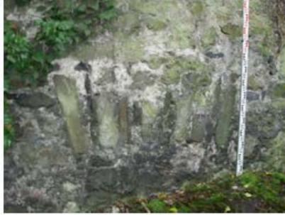
Plate 35. Voussoirs of arch over blocked opening 4.
