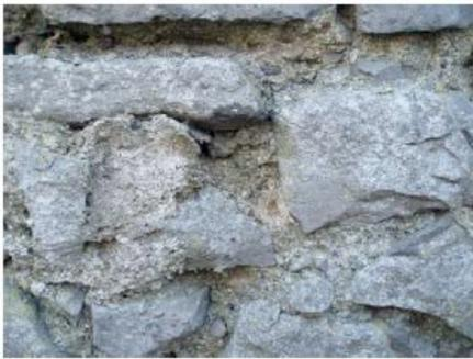
Plate 12. Render of 19th century wall F14 with distinctive pebbles, and later repointing. Many chipped faced stones used.
