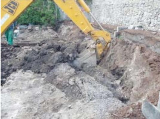
Plate 1. Removal of foundations.
