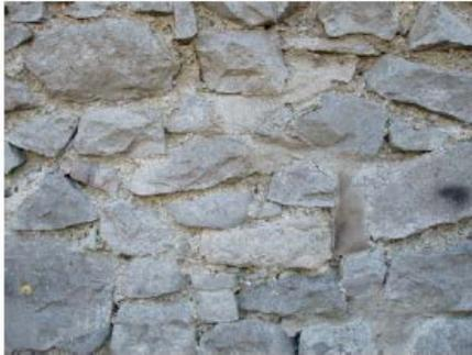
Plate 16. Chipped stone face of 19th century wall.
