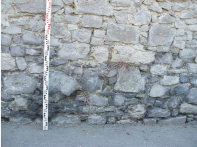
Plate 1. Lower course of wall F12, showing calp masonry.
