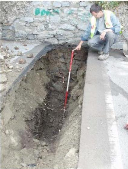
Plate 13. Trial pit 3 in mill race.
