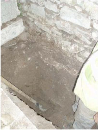
Plate 11. Trial pit 1, shovel at base of wall.
