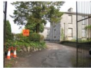
VIEW FROM BARRACK LANE GATES
