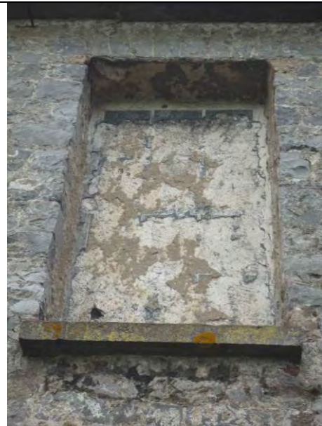
Fig.36: Blind window opening with trace remains of trompe-l'oeil window to first floor (east) of north elevation.
