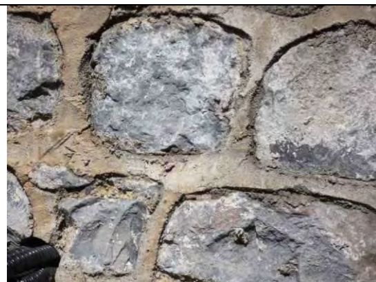
Fig.26: Area of ribbon pointing to the west elevation.
