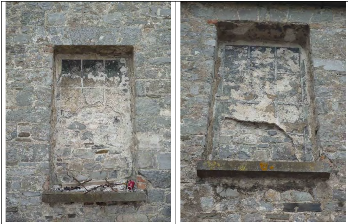
Fig.37: Blind window opening with trace remains of trompe-l'oeil window to ground floor (west) of north elevation.
