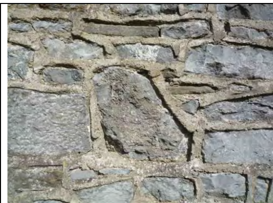
Fig.25: Cementitious strap pointing to the south elevation of the south wing.
