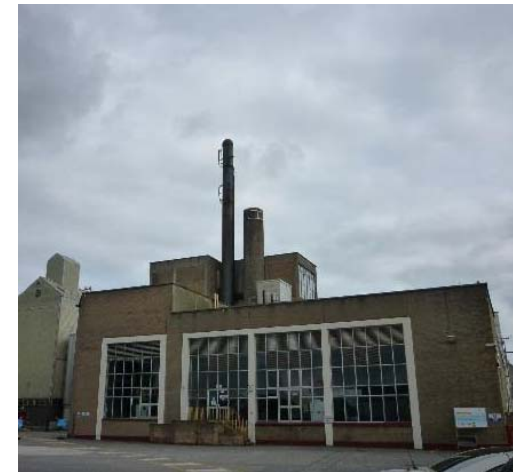
Existing – The Brewhouse
