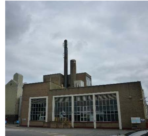
Existing – The Brewhouse
