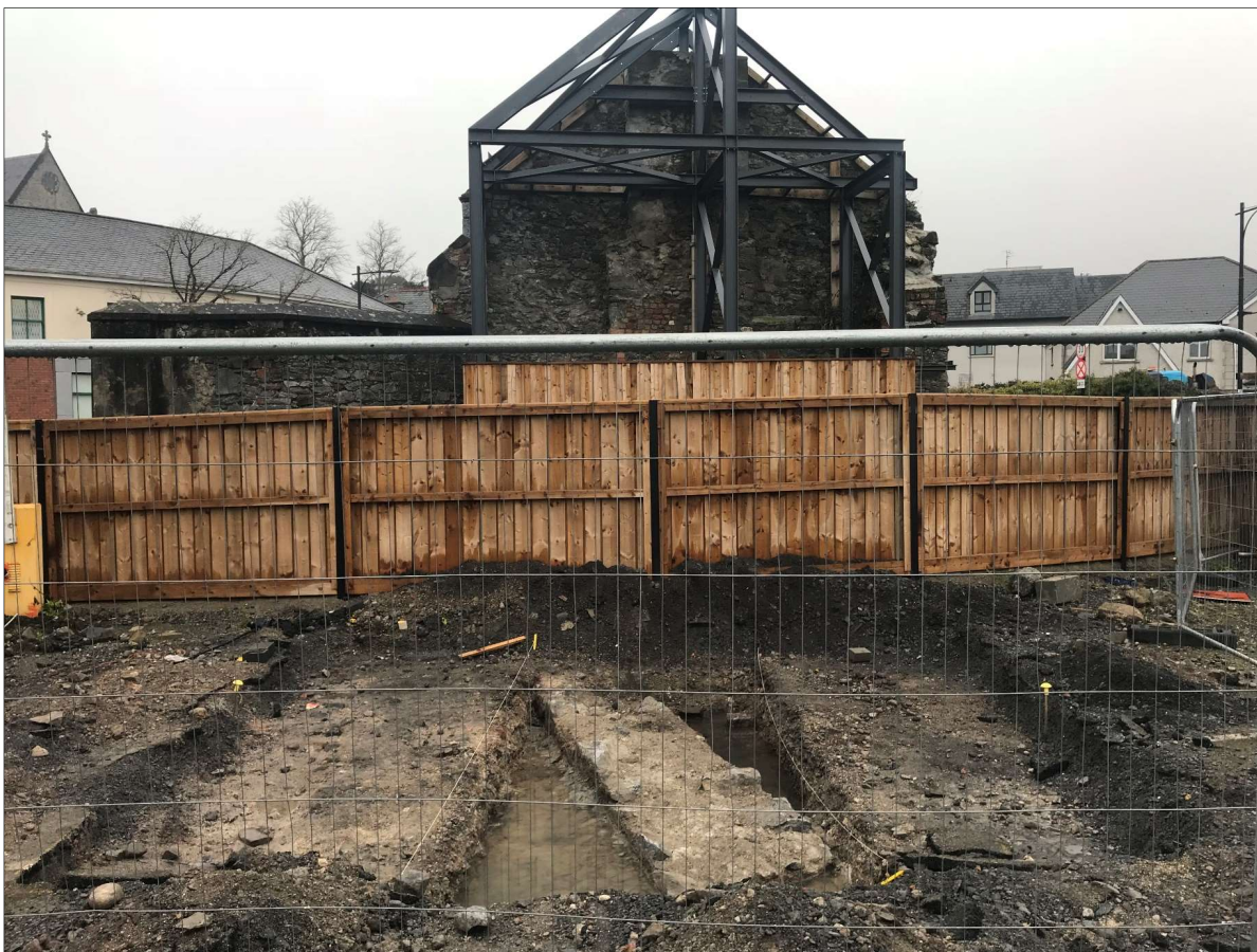
Plate 4: Masonry walls in Test Trench 1, Urban Block 12, with the preserved gable of No. 22 Vicar Street in the background.
