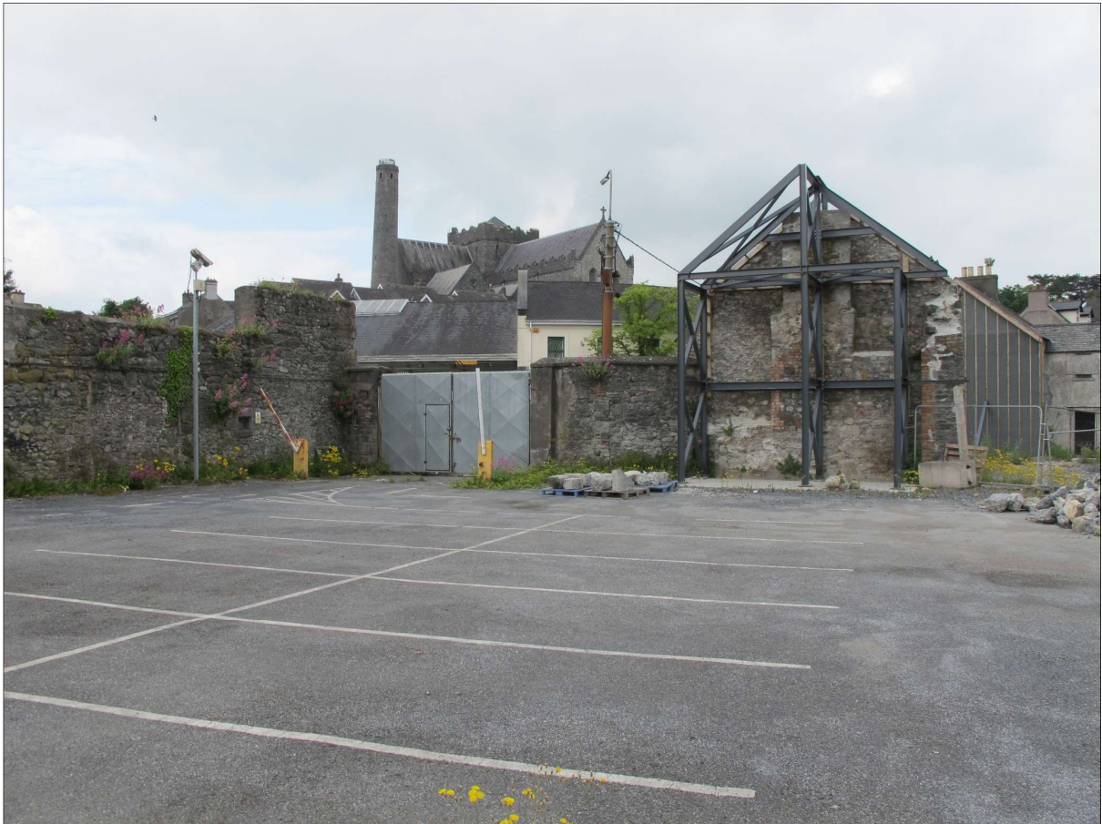
Plate 3: North end of the Bull Inn and the preserved gable of No. 22 Vicar Street
