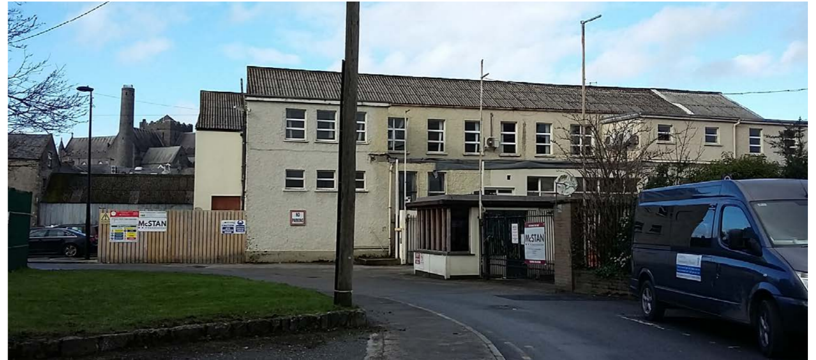
View of South Facade from Horse Barrack Lane
