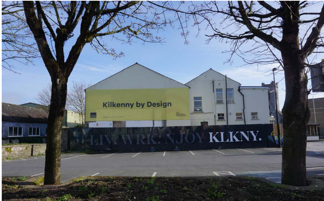
View of West Facade facing Irishtown
