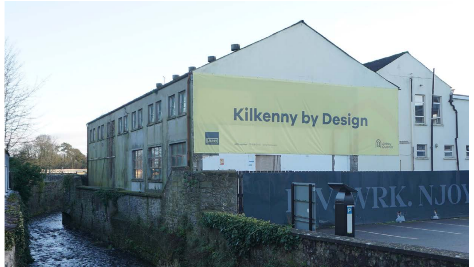
View of the North Facade from the bridge at Irishtown
