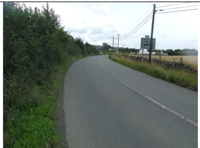
Plate 8: Showing existing R699 in Kiltorcan townland, facing south.
