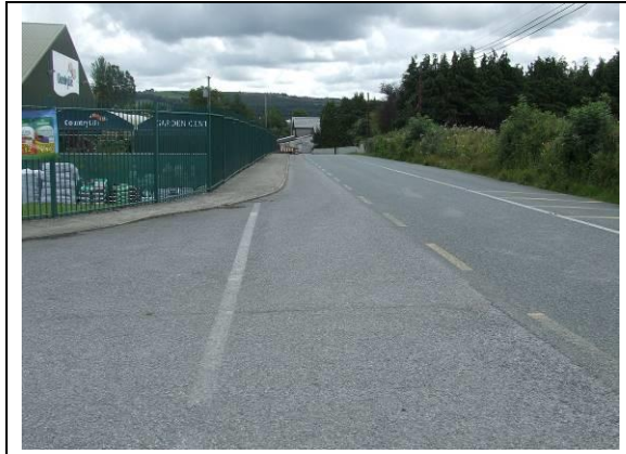
Plate 1 Existing R699 at Knocktopher Manor, outside Glanbia at northern end of project, facing southeast.
