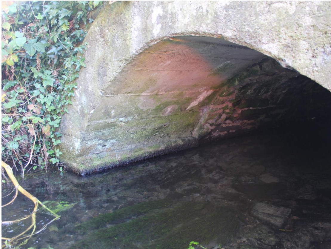
Figure 20: Barrel arch of bridge showing the changing building materials and profile
