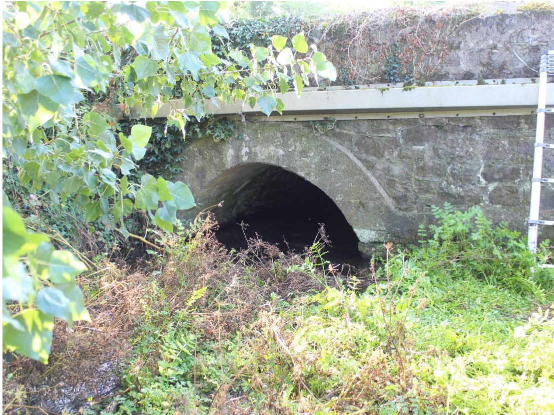
Figure 18: Northern elevation of bridge (eastern arch)
