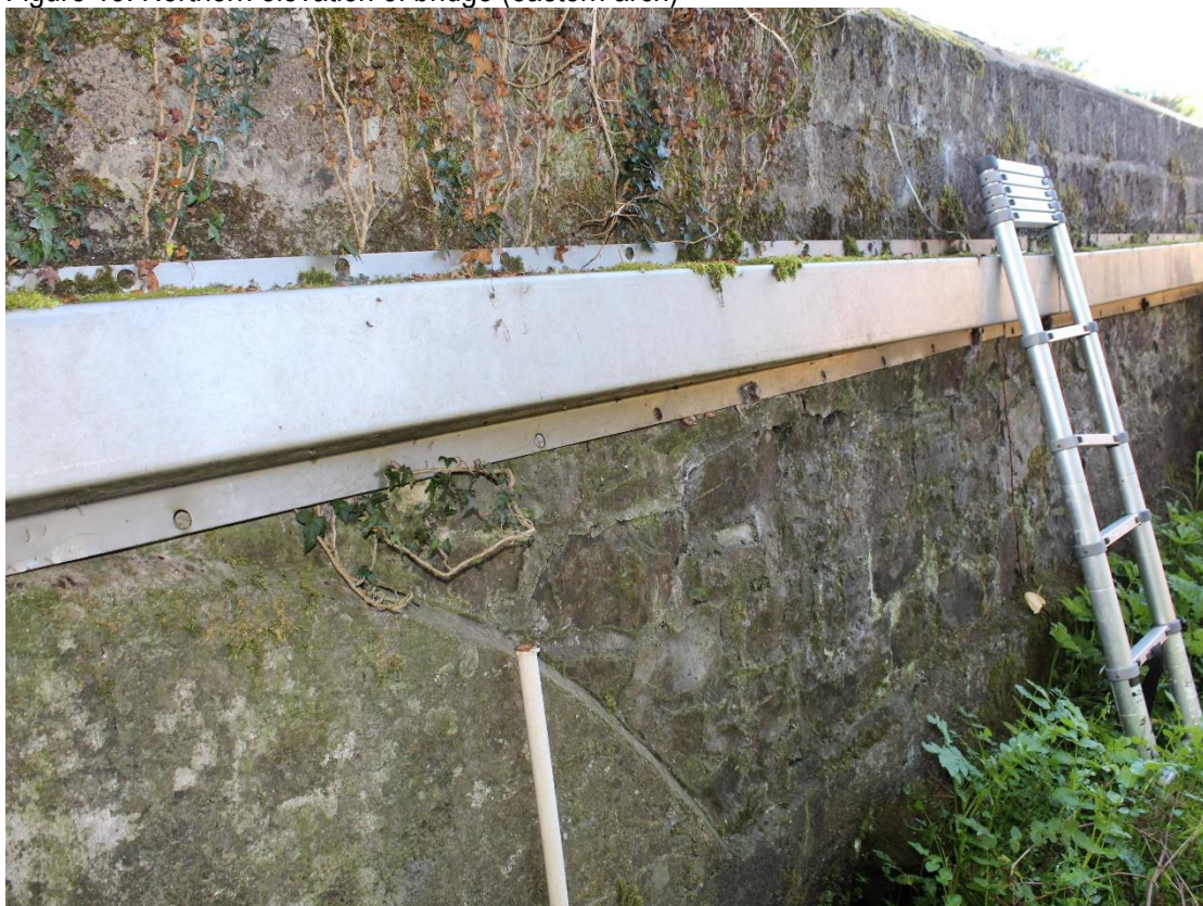
Figure 19: Stonework along northern elevation
