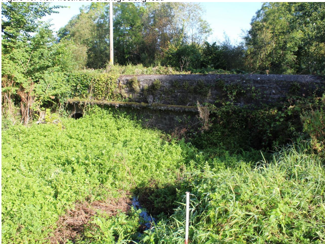
Figure 17: Southern elevation of bridge
