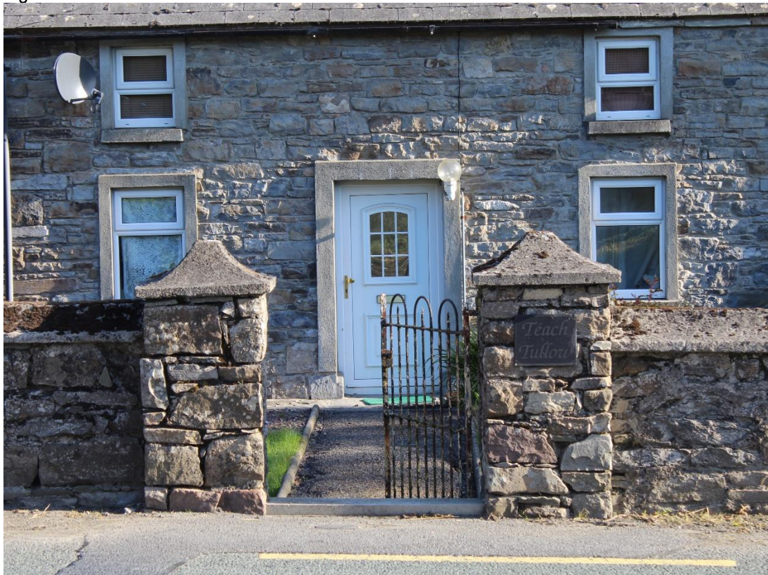
Figure 11: Gate piers and gate
