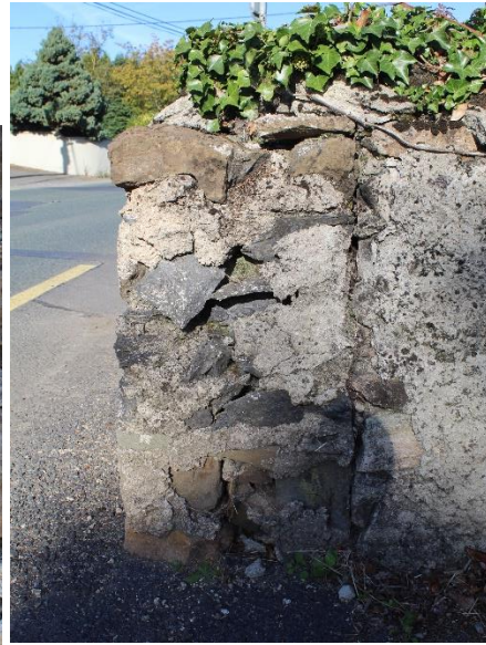
Figure 12: Detail of rubble stone and mortar construction and Figure 13: Cross section of wall
