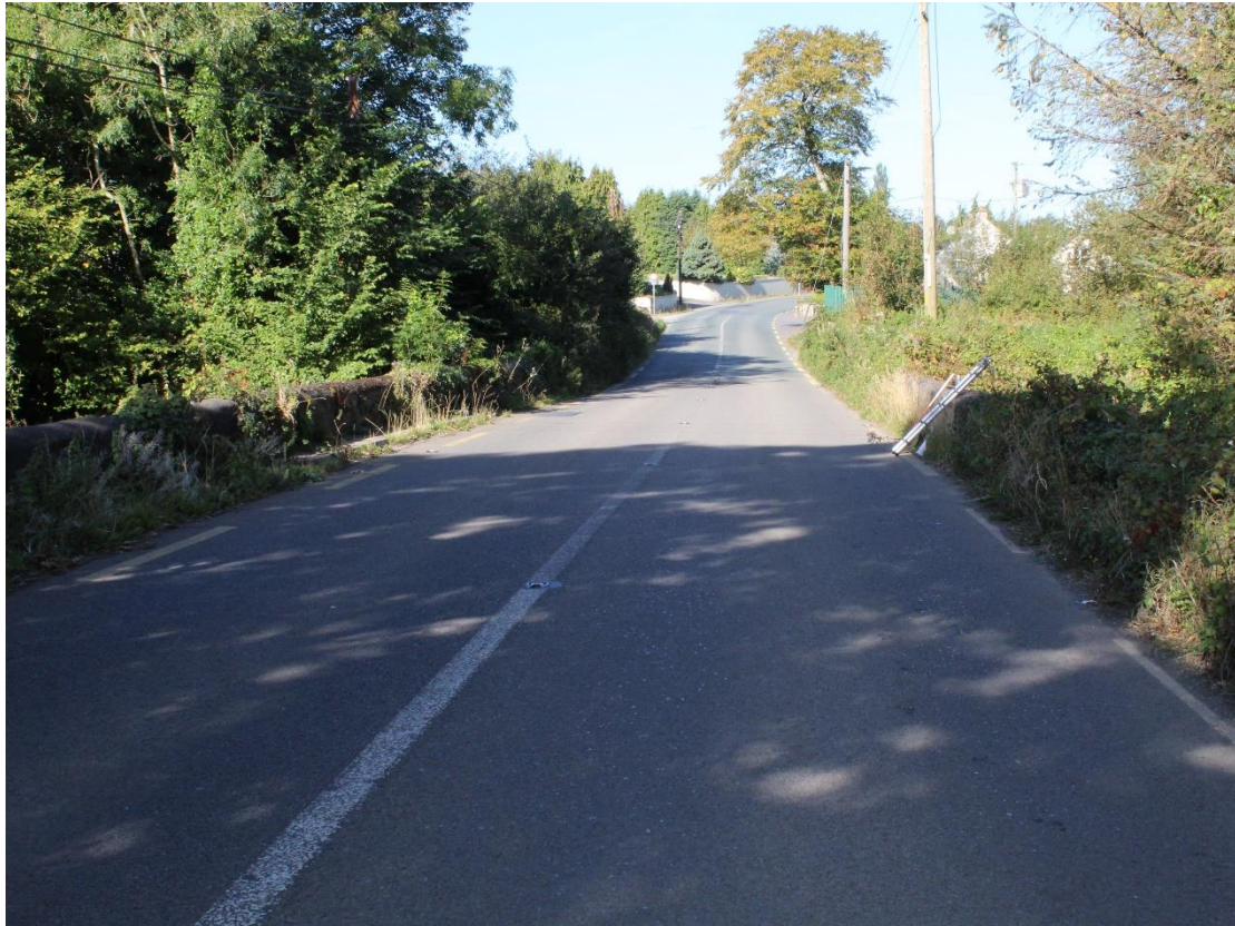
Figure 16: View westwards of bridge along road
