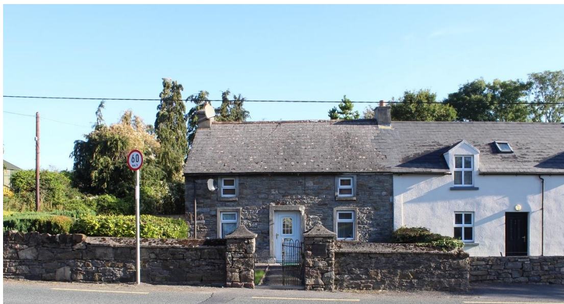
Figure 7: Front elevation of nineteenth century house and boundary wall
