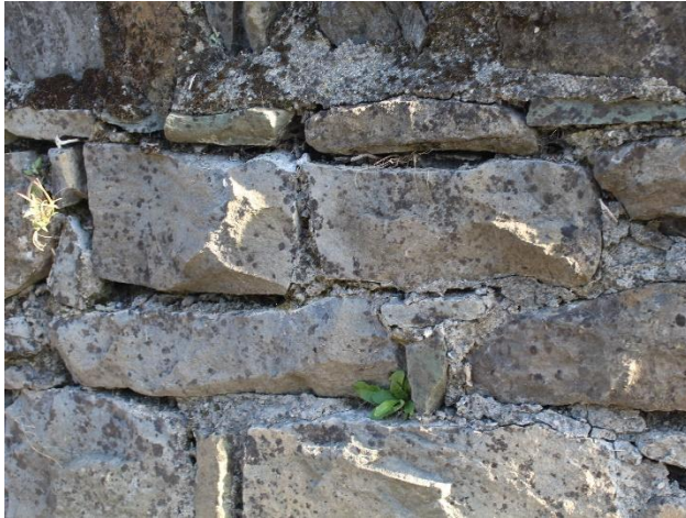
Figure 12: Detail of rubble stone and mortar construction and Figure 13: Cross section of wall
