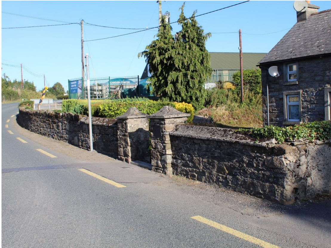
Figure 10: View of house and wall from east
