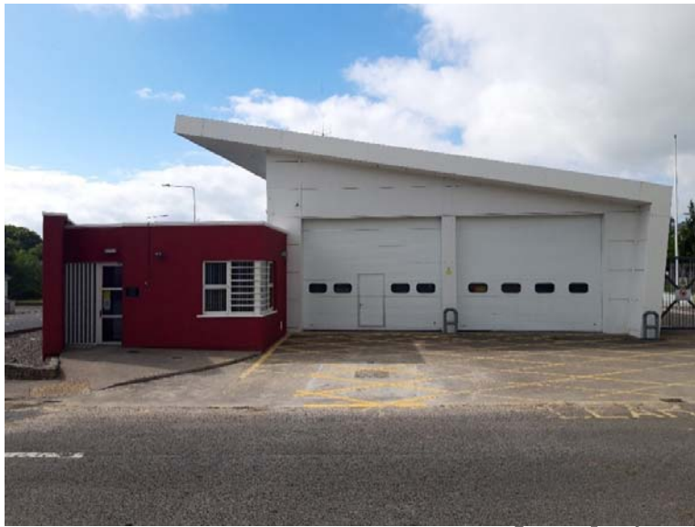
Figure 4:4: Castlecomer Fire Station
