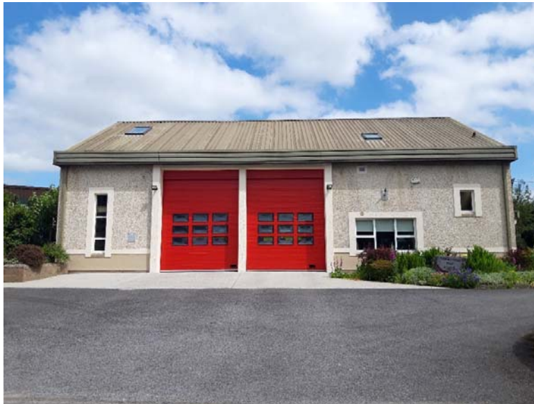
Figure 4:10: Thomastown Fire Station
