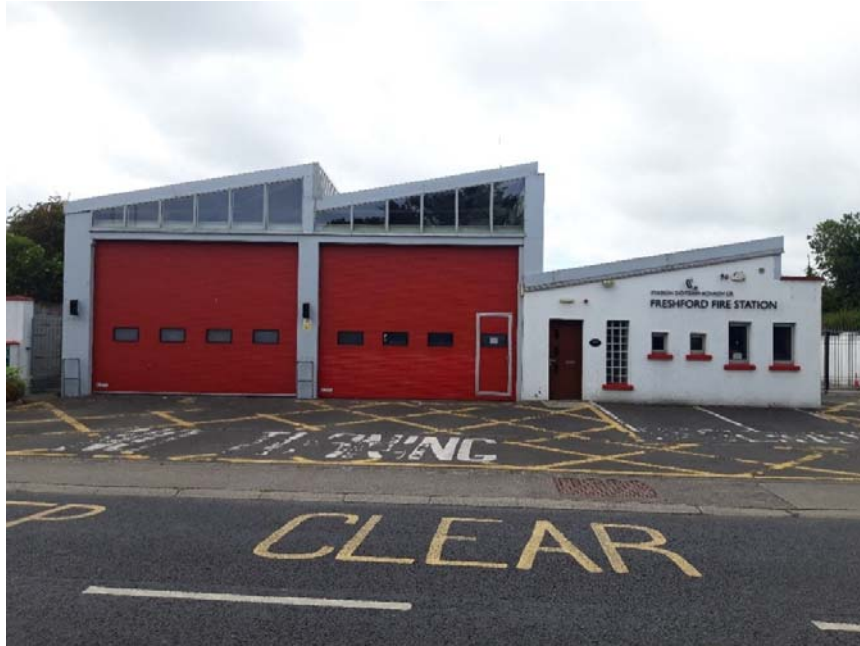
Figure 4:6: Freshford Fire Station
