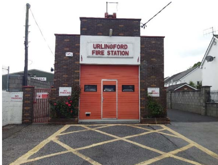
Figure 4:8: Urlingford Fire Station
