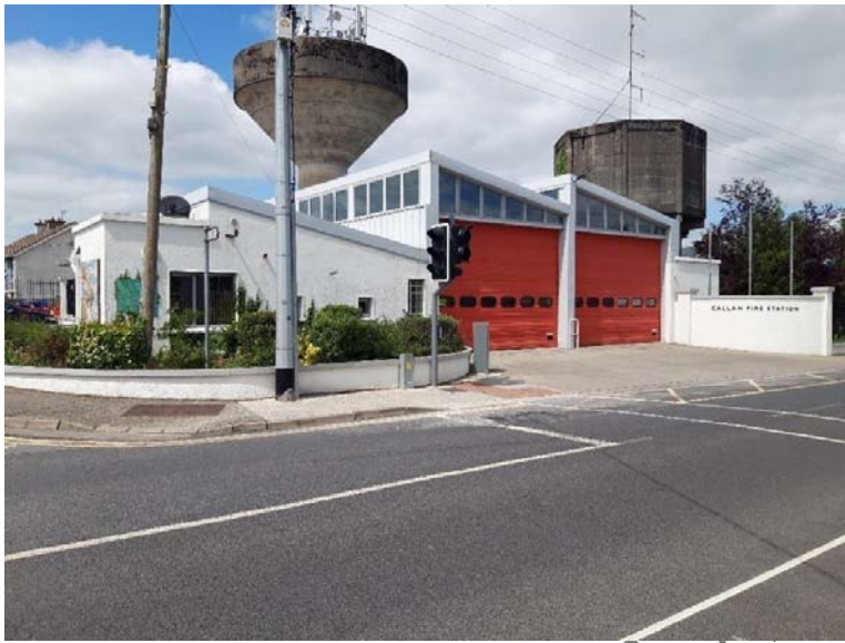
Figure 4:12: Callan Fire Station
