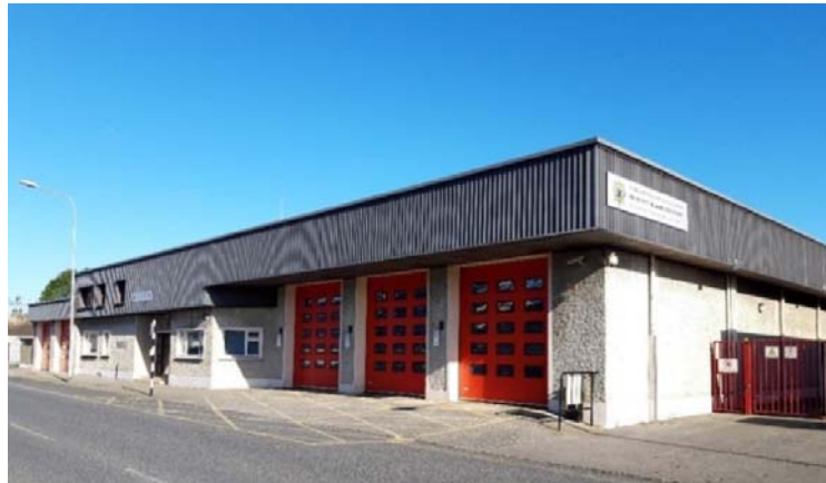
Figure 4:2: Kilkenny City Fire Station
