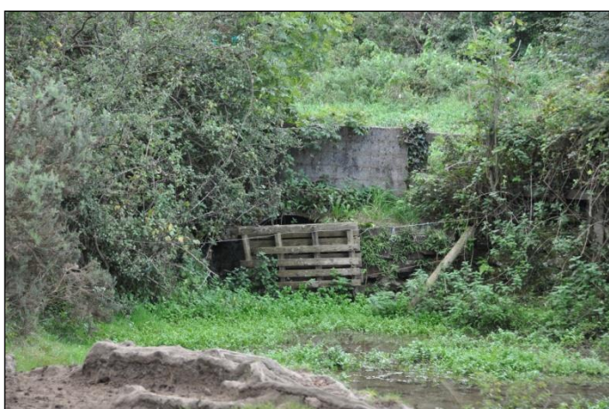
Plate 5 The bridge over Skelpstown stream is low, overgrown with bramble and passage underneath is blocked with a wooden palette.
