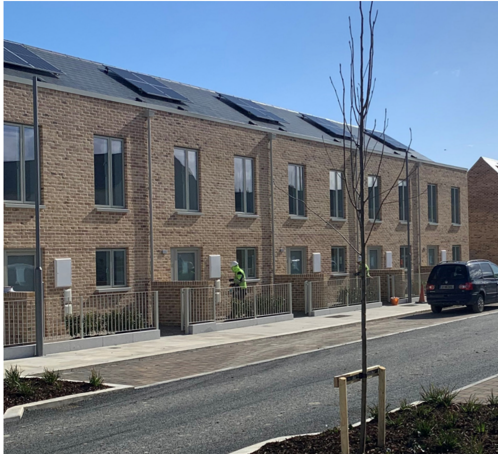
Ballyogan, Dún Laoghaire–Rathdown - van Dijk Architects Metal railing to defensible spaces at the front of the houses
