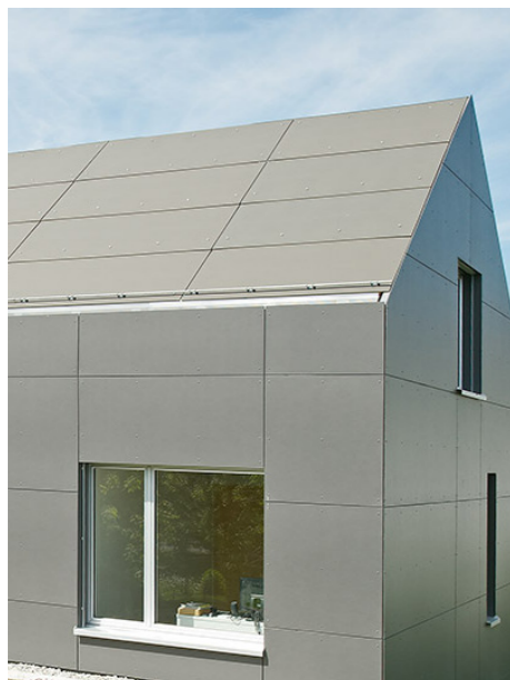
Fibre cement cladding Feature cladding to blocks 3 and 7
