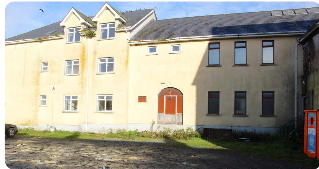
Figure 3.13: Vacant Buildings with residential potential.
