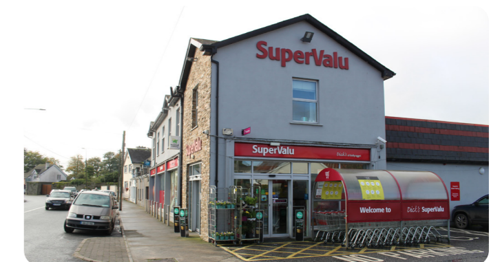
Figure 3.31: Supervalu Supermarket in Ballyragget
