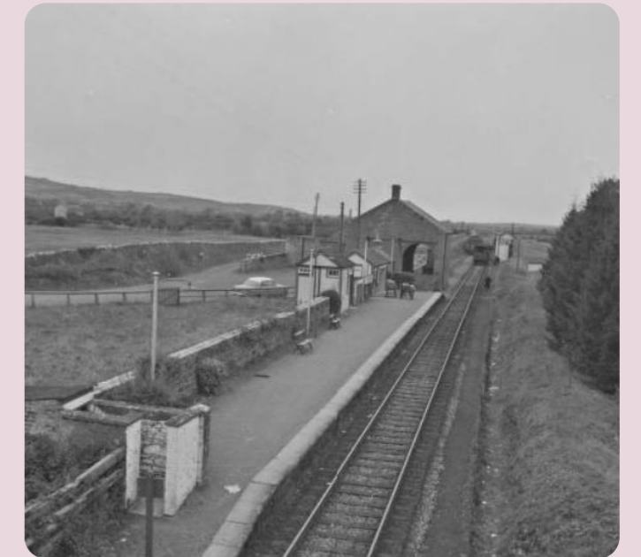
Railway Station in 1960s before track lifted Source: National Library of Ireland.
