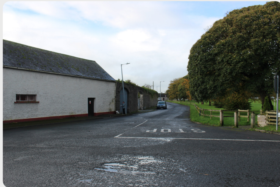
Figure 3.54: Road south of Fair Green without Pavements.
