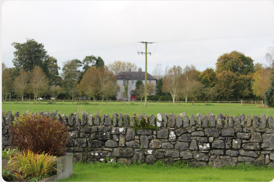
Figure 3.21: Ballyragget Lodge (Formerly Ballyragget Convent of Mercy).
