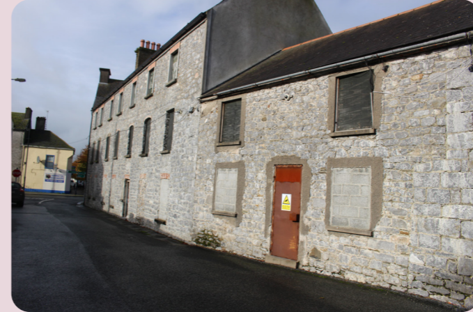
Butler's House from the rear
