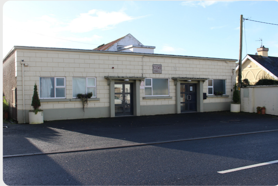
Figure 3.34: CYMS Hall Ballyragget or the Ballyragget Community Hall.
