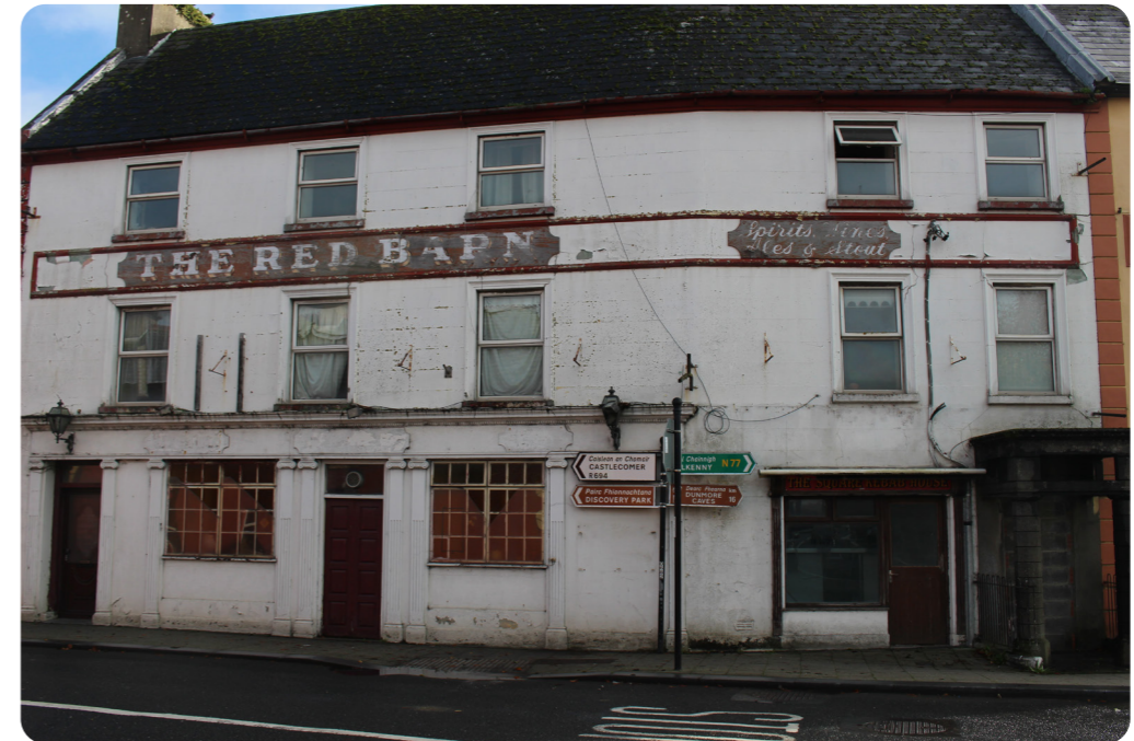
Vacant and derelict Red Barn Building facing onto the Square.
