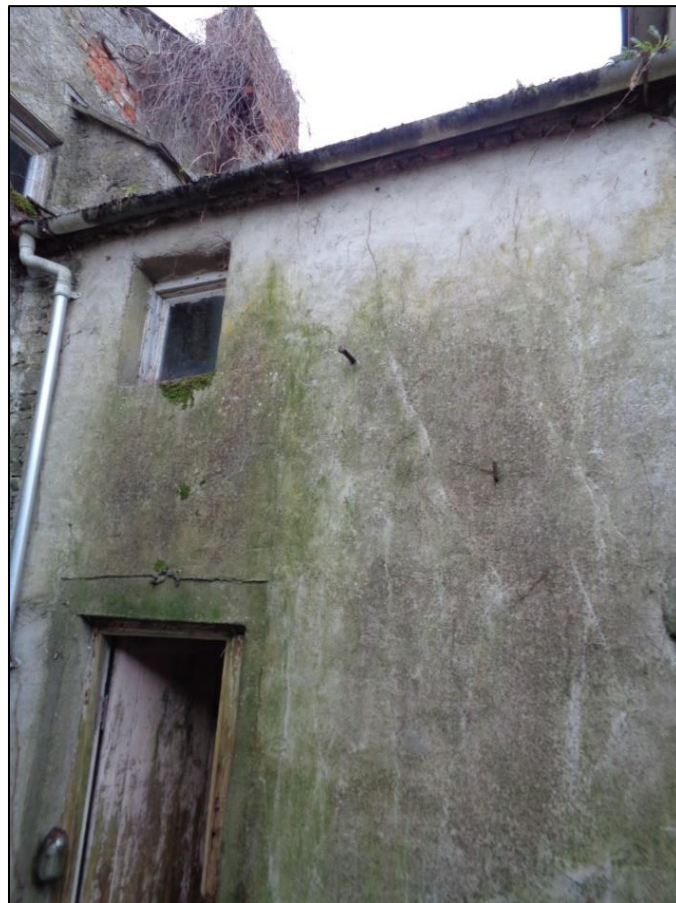
Pl.17. Rear Wall of No.8.
