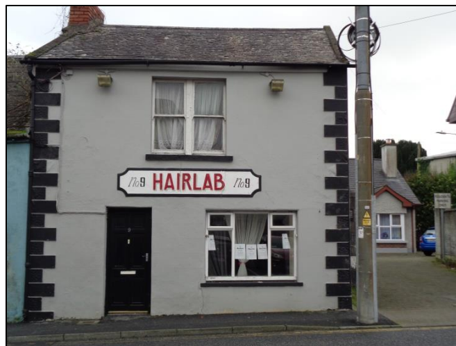
Pl.20. Front Façade of No.9.
