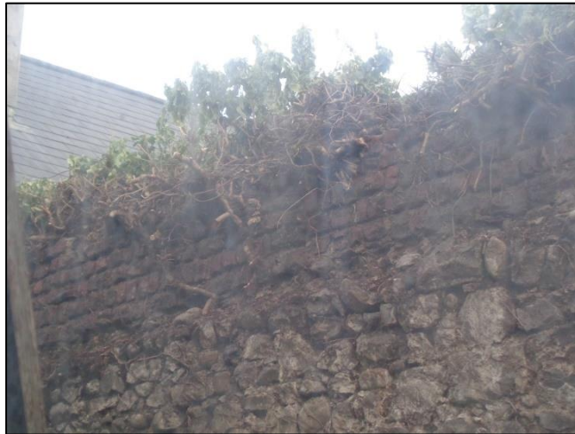
Pl.13. Red Brick in Rear Wall of Nos. 6 & 7.
