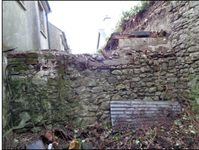
Pl.18. North Boundary Wall of Yard to No.8.
