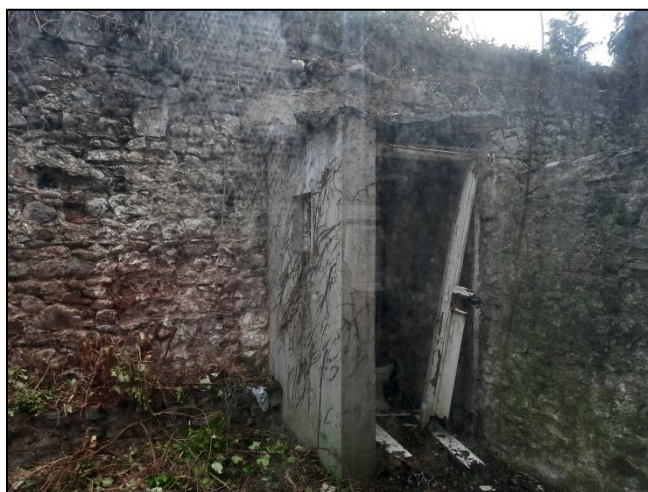
Pl.11. Rear Boundary Wall and Outdoor Toilet.
