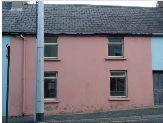
Pl.6. Front Façade of No. 7 Upper Patrick St.
