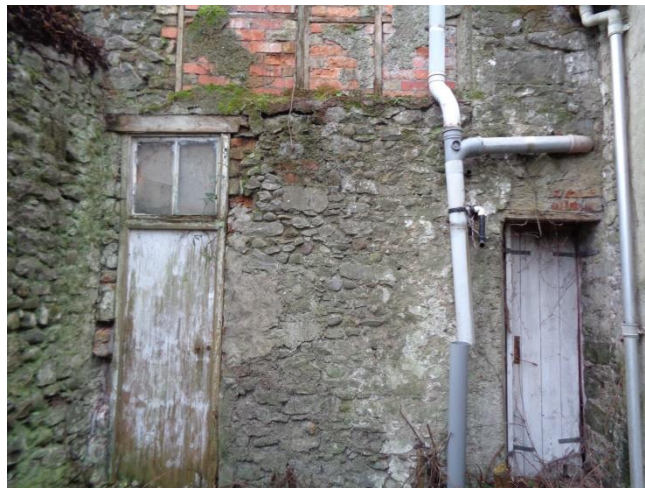
Pl.19. South Boundary Wall of Yard to No.8 (Extension Building to No.9).
