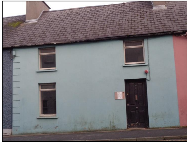
Pl.2. Front Façade of No. 6 Upper Patrick St.
