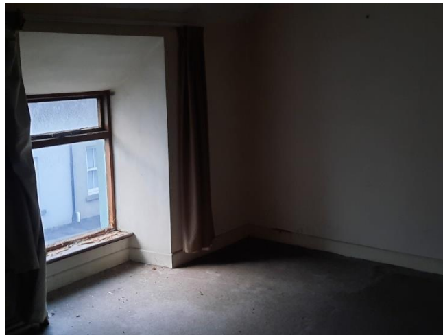
Pl. 5. First Floor Room in No.6.
