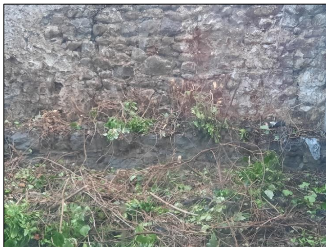
Pl. 14. Plinth at Base of Boundary Wall at No. 7.
