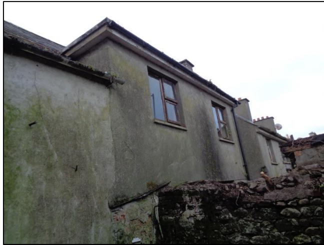
Pl.8. Rear Wall of No. 7.
