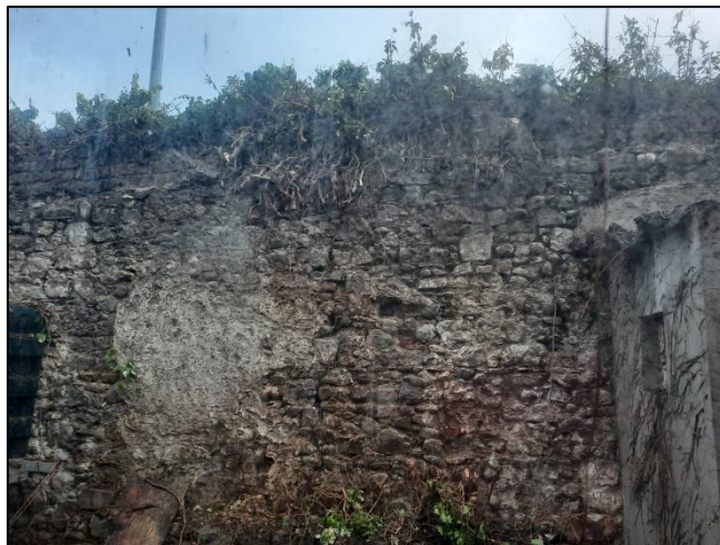
Pl.10. Rear Site Boundary Wall to Nos. 6 & 7.
