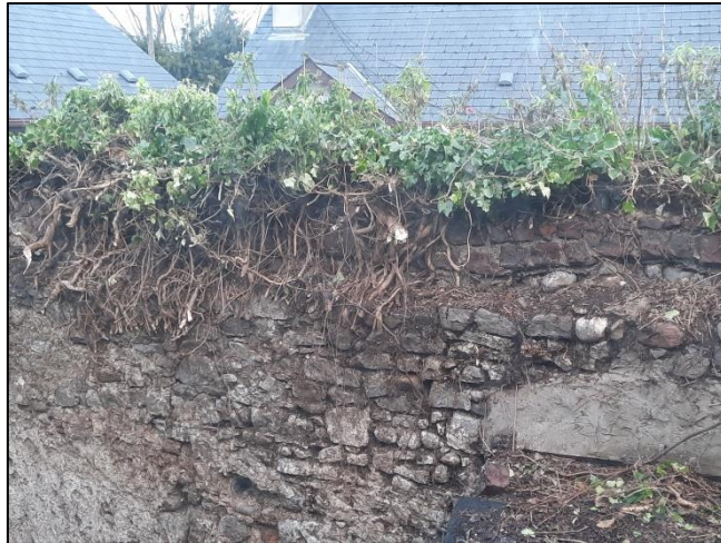
Pl.12. Upper Section of Rear Wall and Remains of Blocked up Ope.
