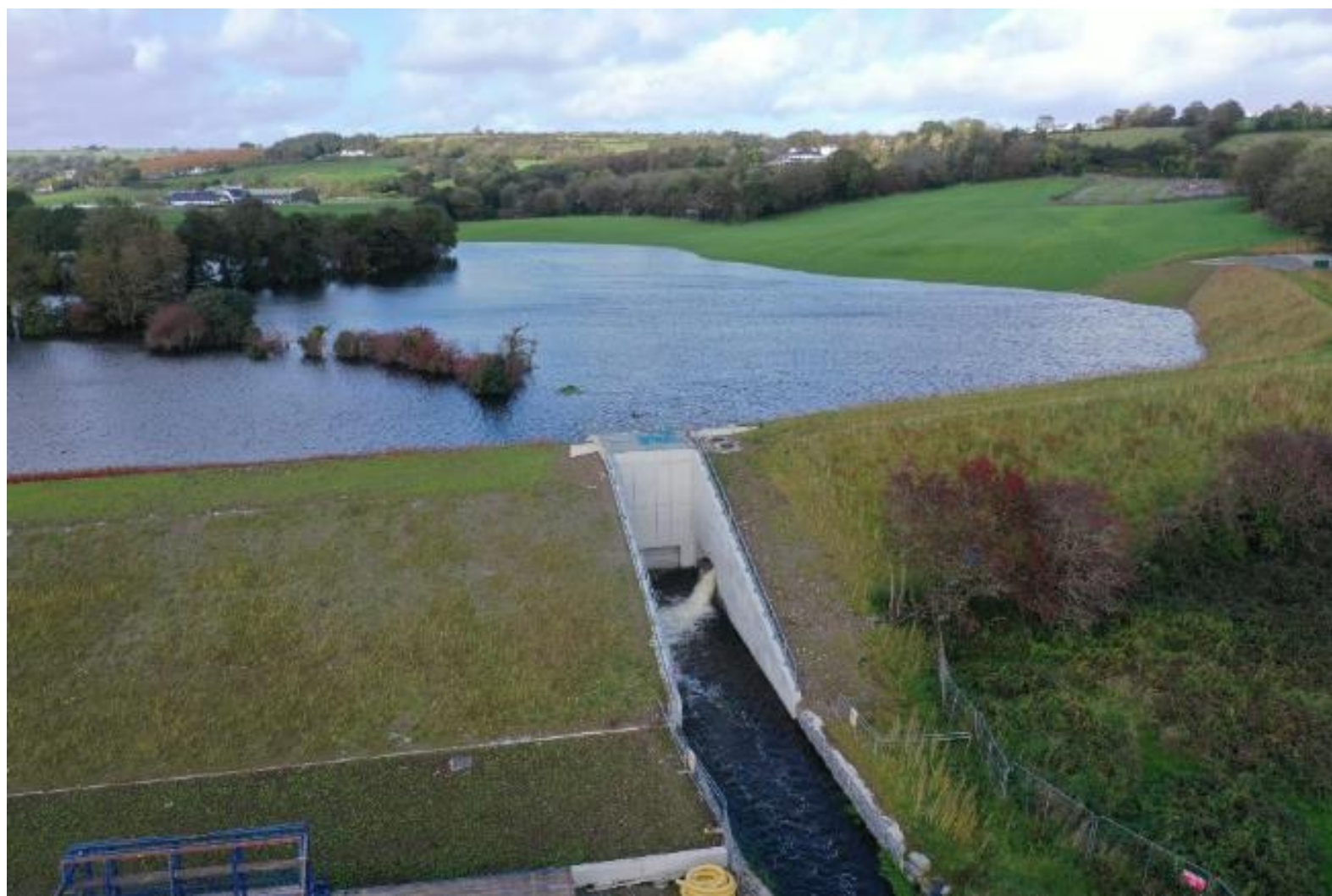
Example of storage area with flow control (River Feagle, Clonakilty)
