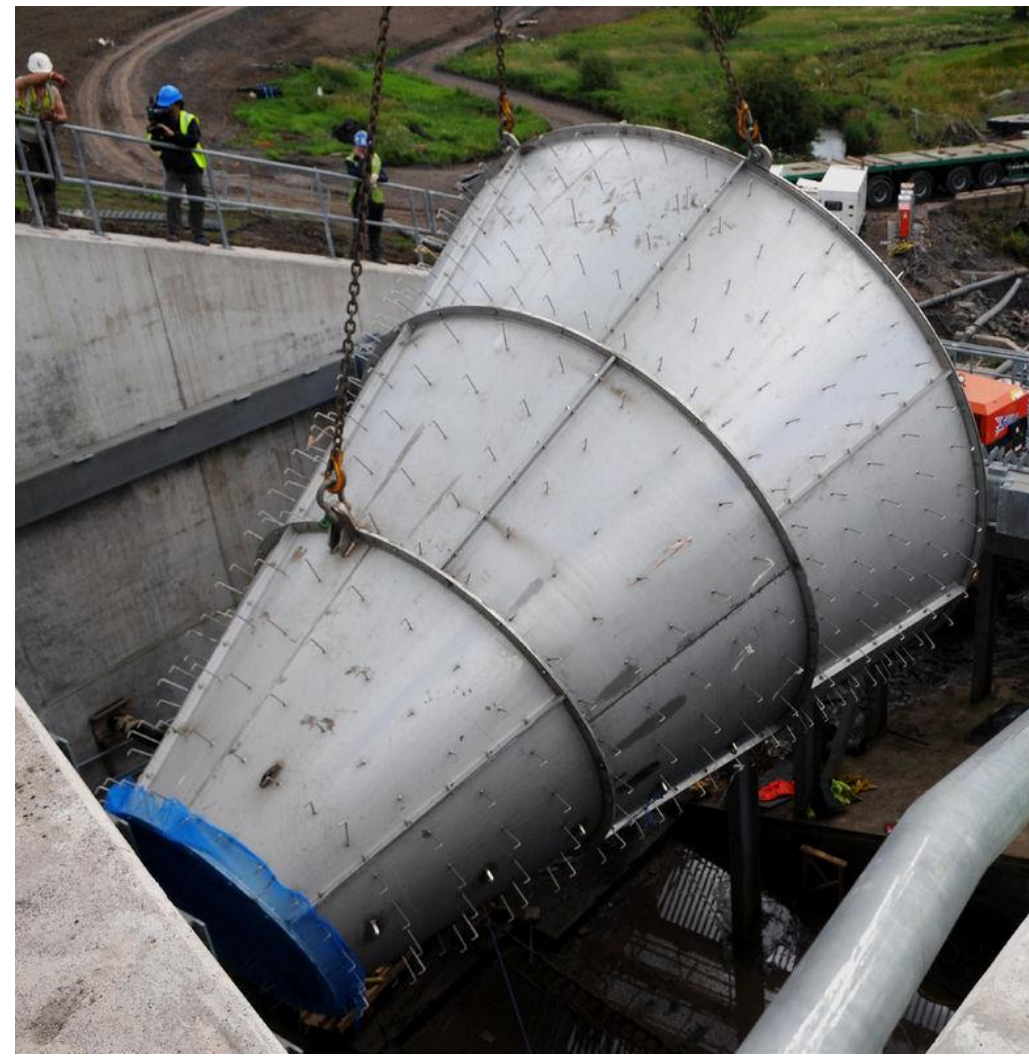
Hydro-Brake Flood flow control for flood prevention
