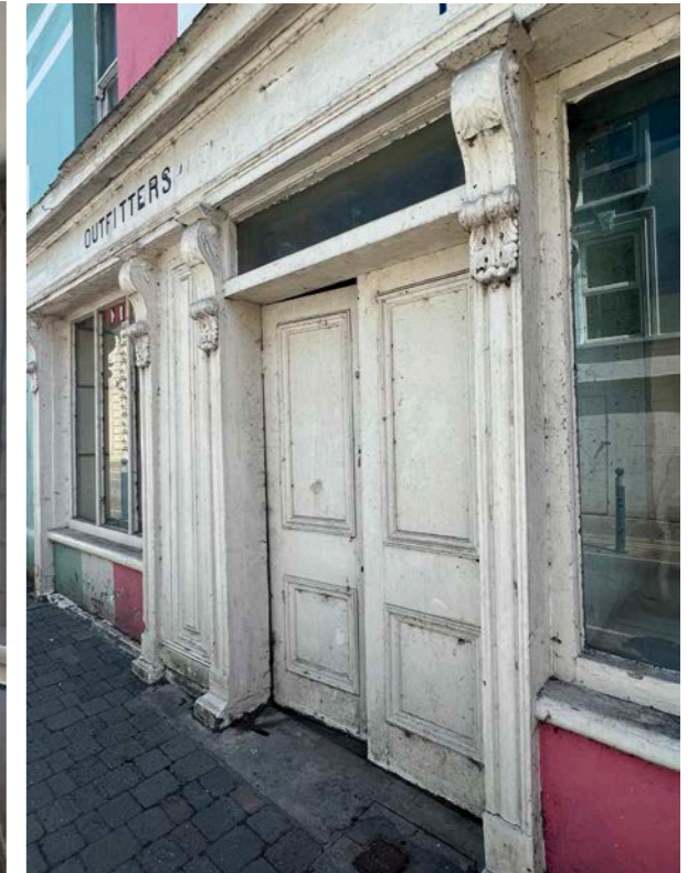
18 - SHOP FRONT AND MAIN FRONT DOOR
