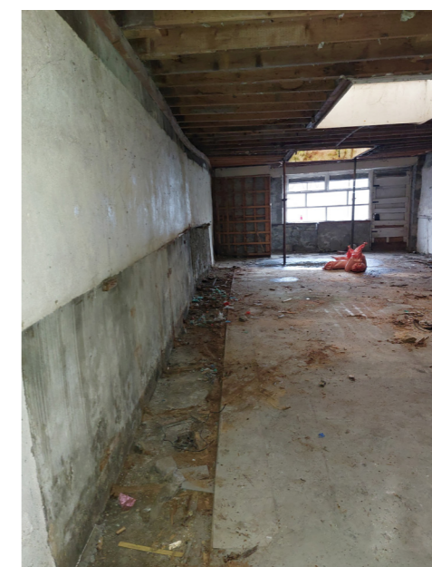
VIEW OF LOUNGE, SINGLE STOREY EXTENSION
