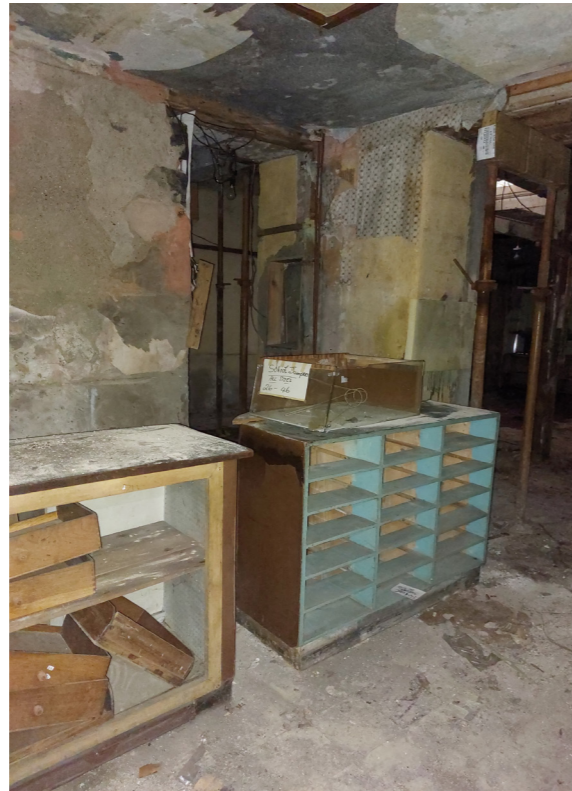
18 - VIEW IN ORIGINAL CARRIAGEWAY
