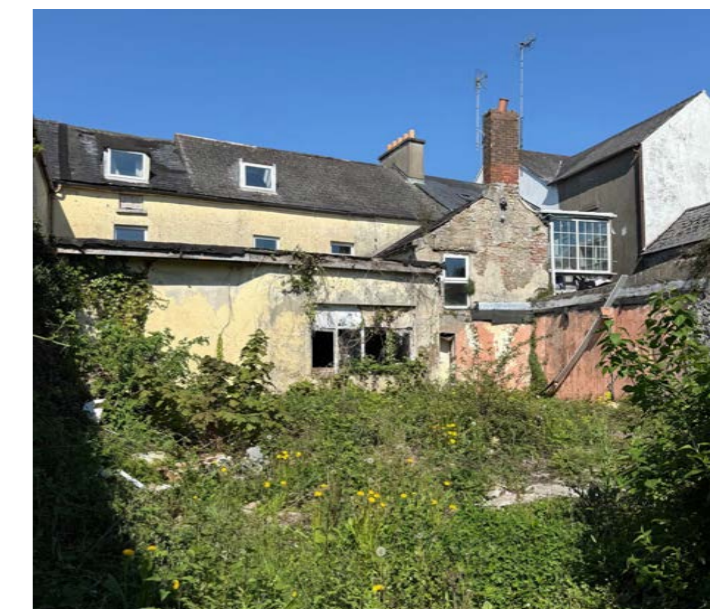
Rear of 18 Powers
