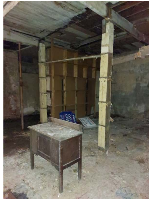
18 - REAR EXTENSION TO BE DEMOLISHED
