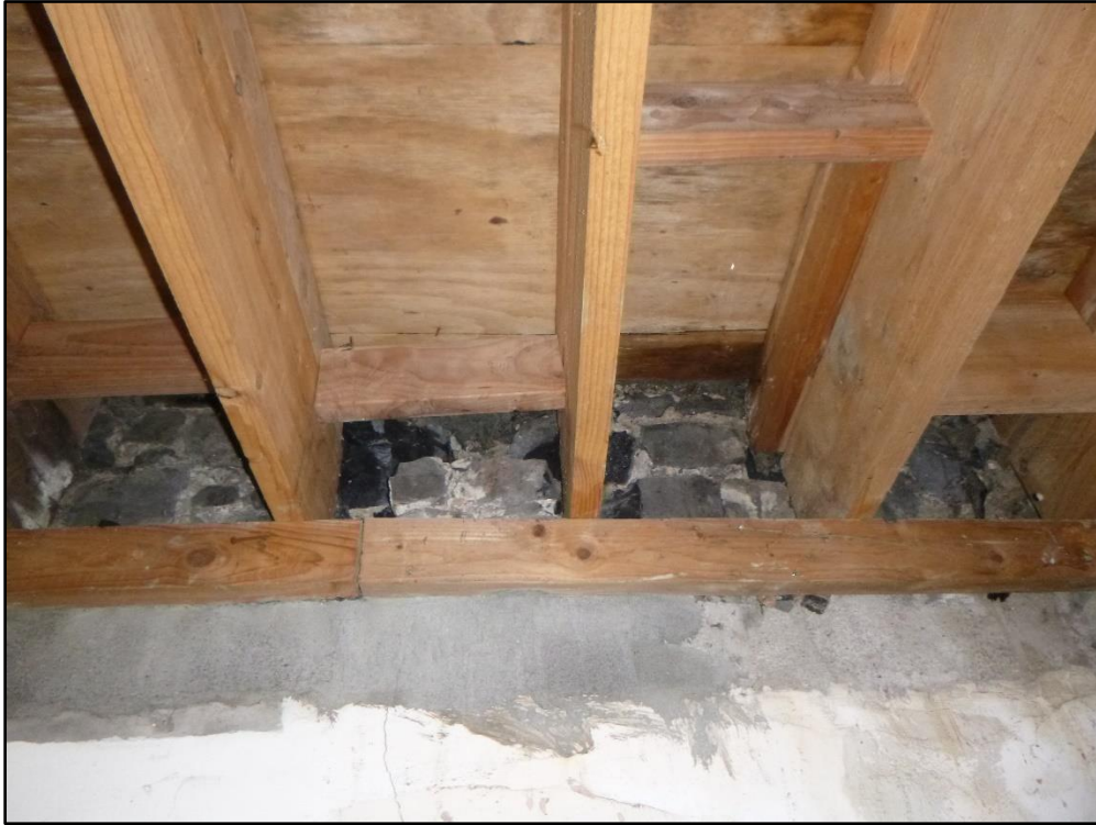
Plate 11 Roof detail of rear lounge to No. 20 set in stonework of rear S boundary wall (Source: Shanarc Archaeology Ltd. 10.04.2024).
