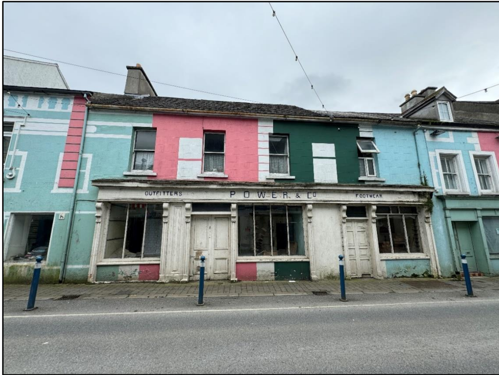
Plate 2 No. 18 Upper Bridge Street frontage (Source: Shanarc Archaeology Ltd. 21.03.2024).
