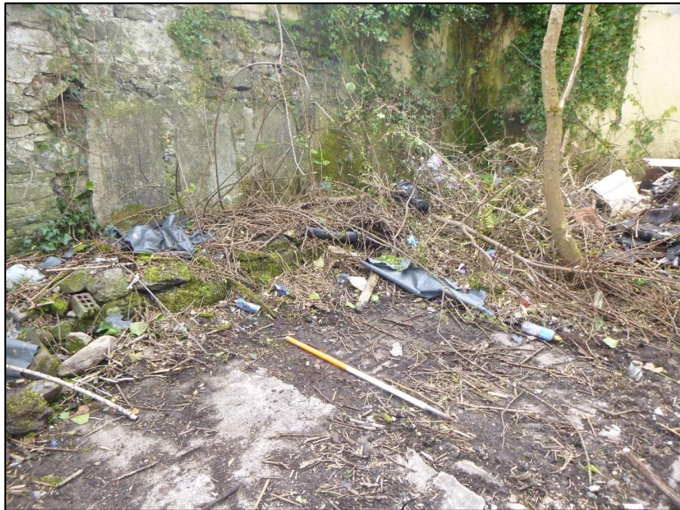
Plate 3 Location of former structure to rear of No. 18, evident in party wall (S side) and on ground surface; drystone retaining to base of party wall (Source: Shanarc Archaeology Ltd. 10.04.2024).
