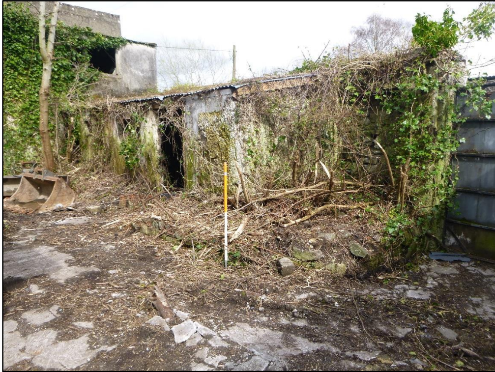
Plate 4 Stone outbuilding abutting Clodeen Lane; built on platform formed to S side by drystone retaining (Source: Shanarc Archaeology Ltd. 10.04.2024).
