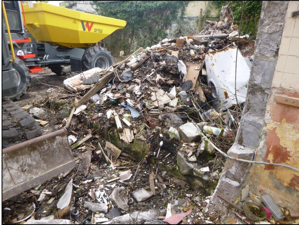
Plate 6 Low remains of mortared stone wall abutting rear of present rear extension to No. 18 (Source: Shanarc Archaeology Ltd. 10.04.2024).
