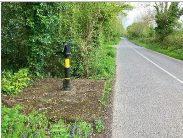
Pump on concrete platform
