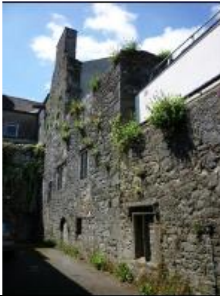
Plate 10 Rear of No 40 Parliament St (along Horse Barrack Lane), the location of the Red Lion Inn, showing 16-18 th century mullioned windows, facing west.
