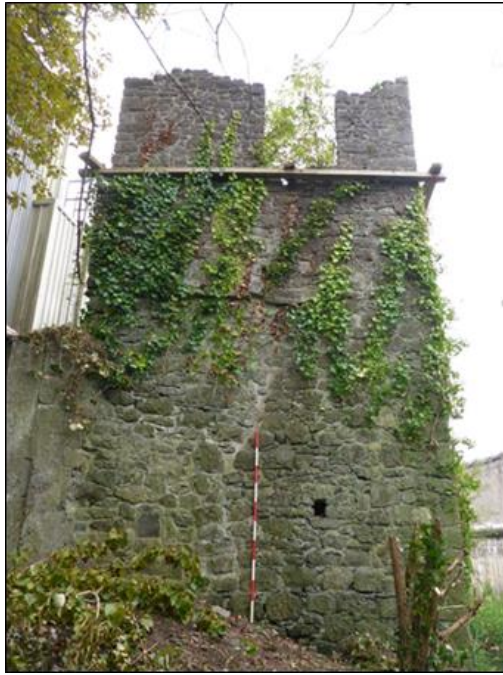
Plate 16 East elevation showing the repair work
