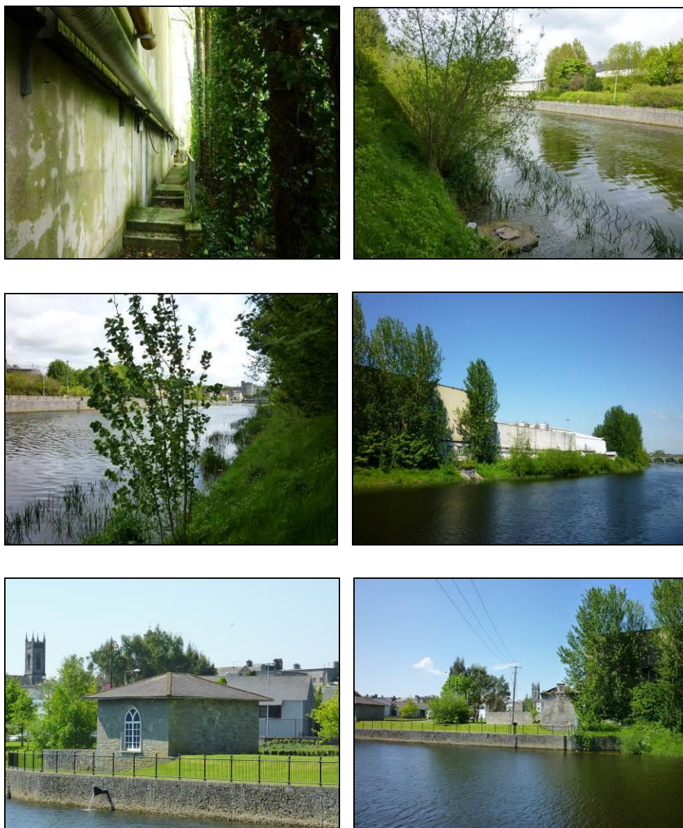
Plates 9-14 show various views of the riverside along the existing Diageo complex.
