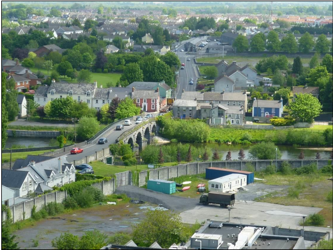
Plate 25 Green's Bridge, view from west to east (NIAH 12004007)
