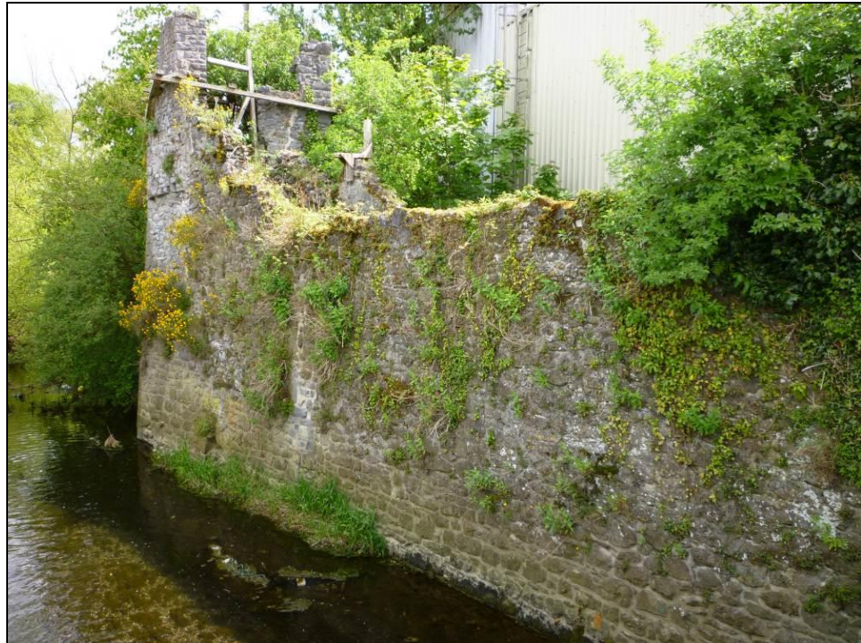
Plate 20 Evan's Tower and wall walk prior to stabilisation works May 2013
