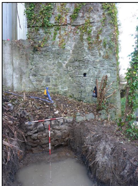
Plate 4 Revetment wall at Evan's Tower
