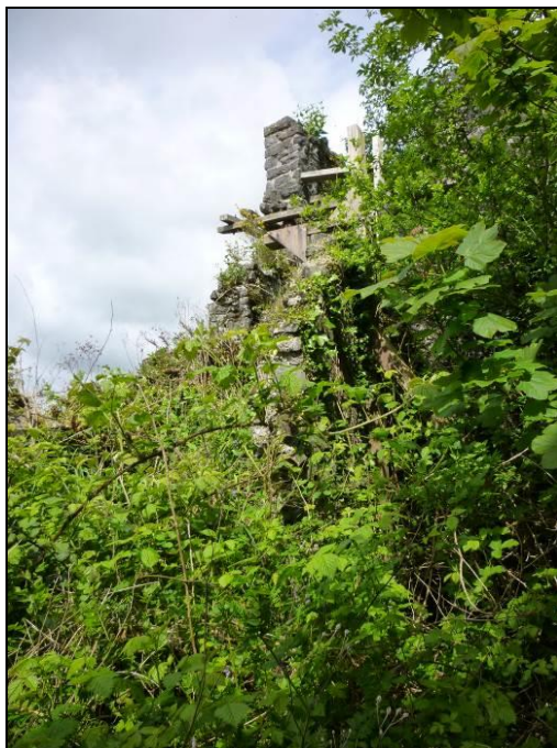
Plate 18 Wall walk 2013 prior to clearance
