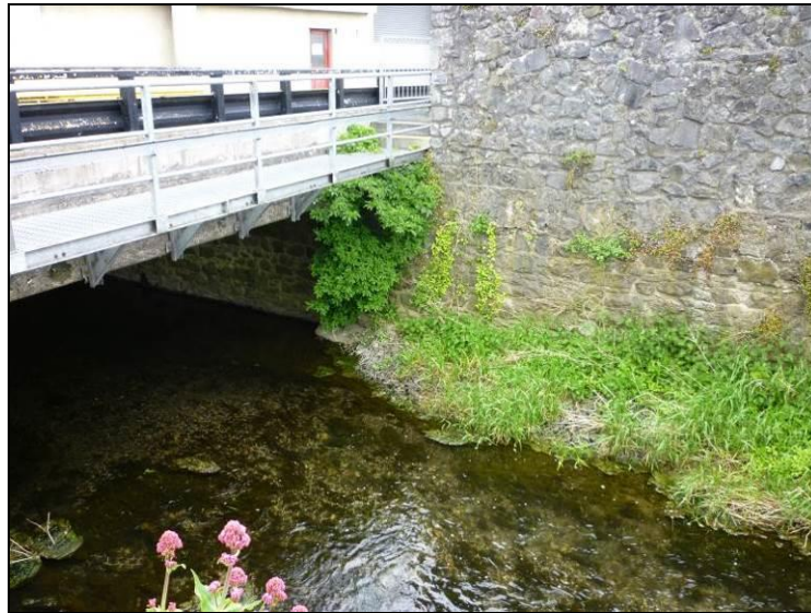
Plate 22 The existing bridge over the River Breagagh
