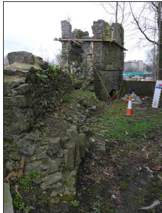
Plate 19 Wall walk after clearance 2015 prior to bracing
