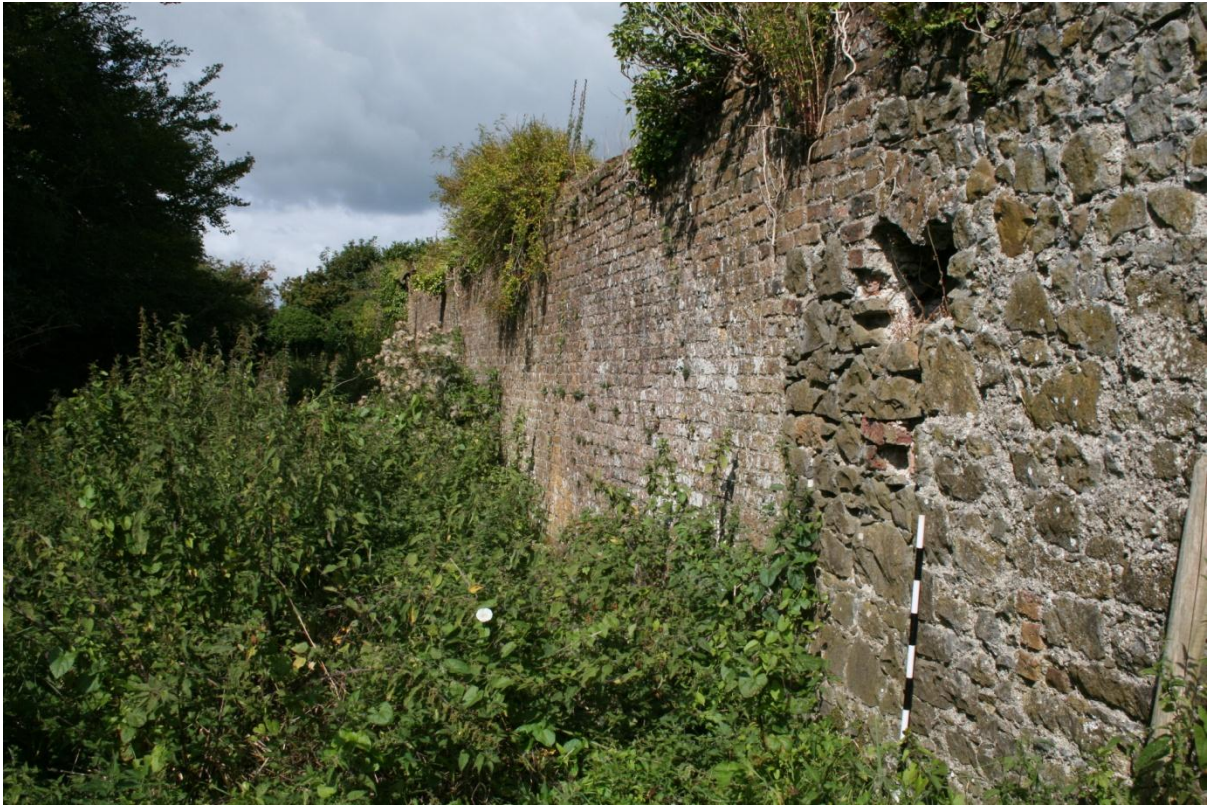
Figure 33: South wall exterior, west end.
