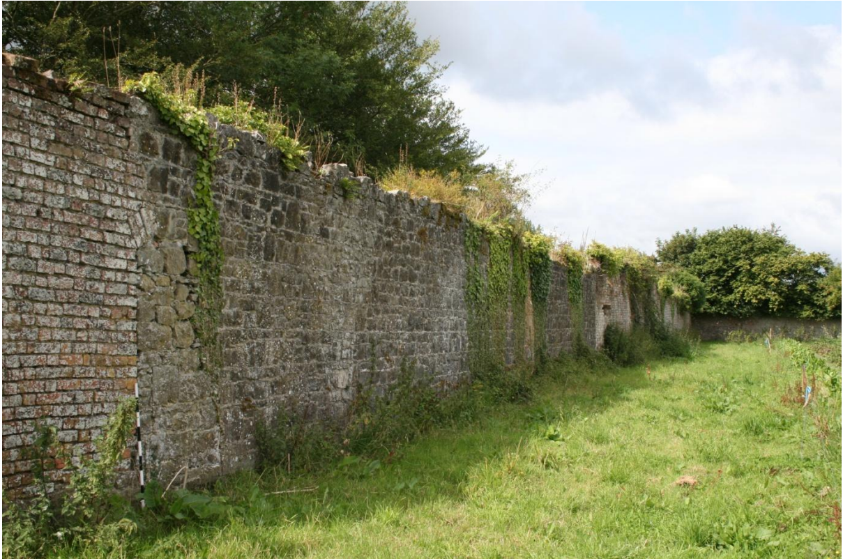
Figure 38: South wall, interior.
