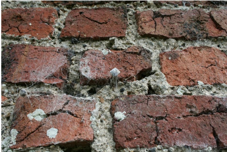
Figure 46: Planting nails on interior of south wall.
