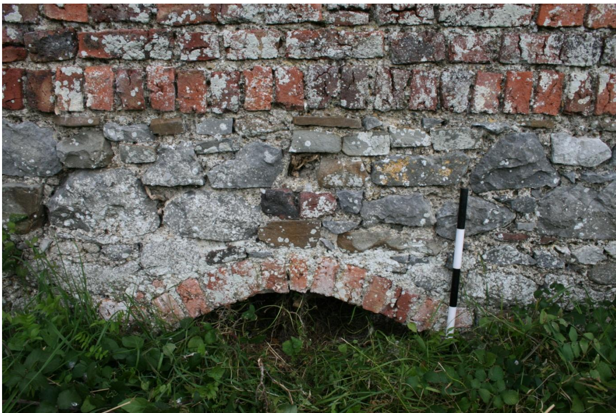
Figure 48: Frost arch in south wall interior, note root from later planting.
