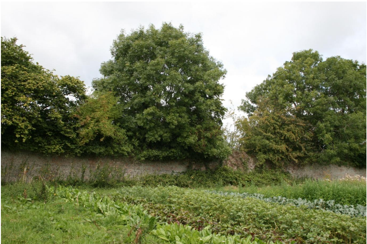
Figure 41: West wall interior, from east.
