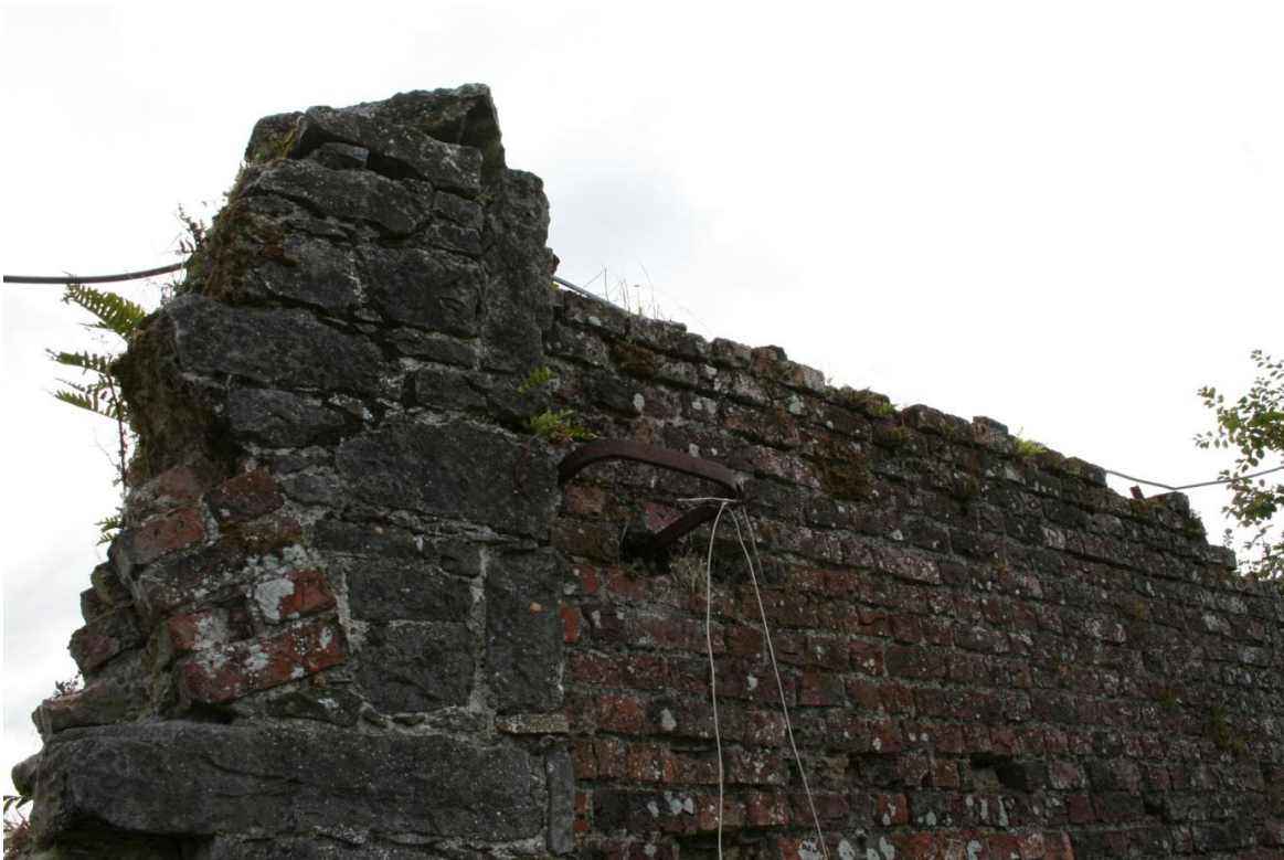
Figure 22: Lamp hanger beside cart entrance, east wall interior.
