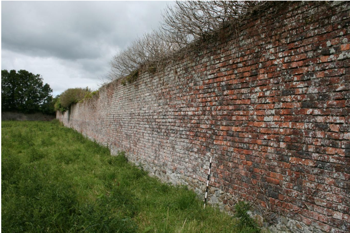
Figure 50: South wall interior, west side..
