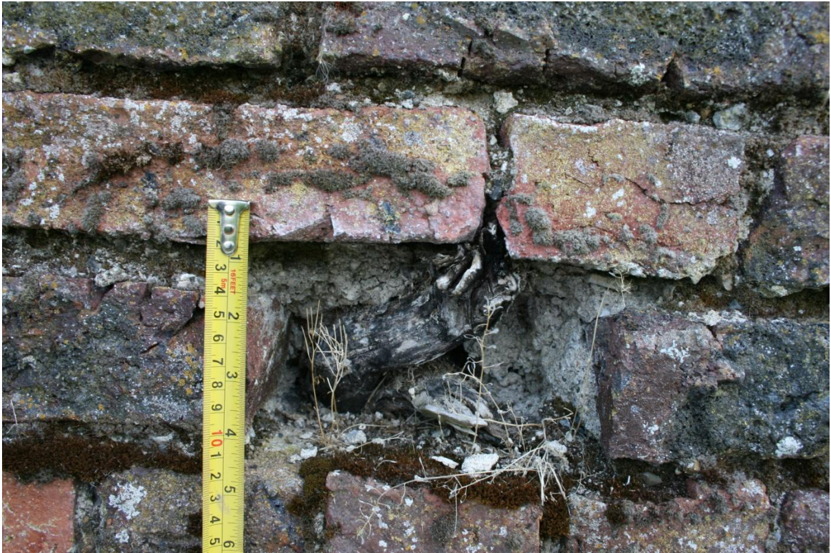
Figure 27: Planting within the brick wall east wall interior.
