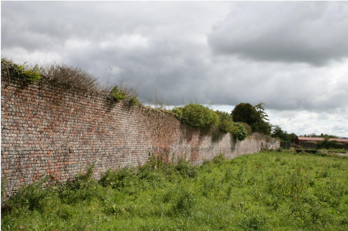
Figure 44: North wall interior from south-west.
