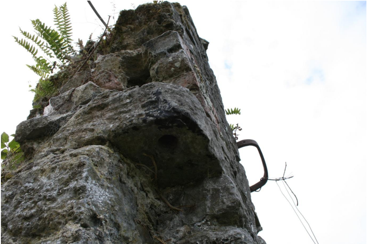
Figure 21: Spud stone for gate to cart entrance
