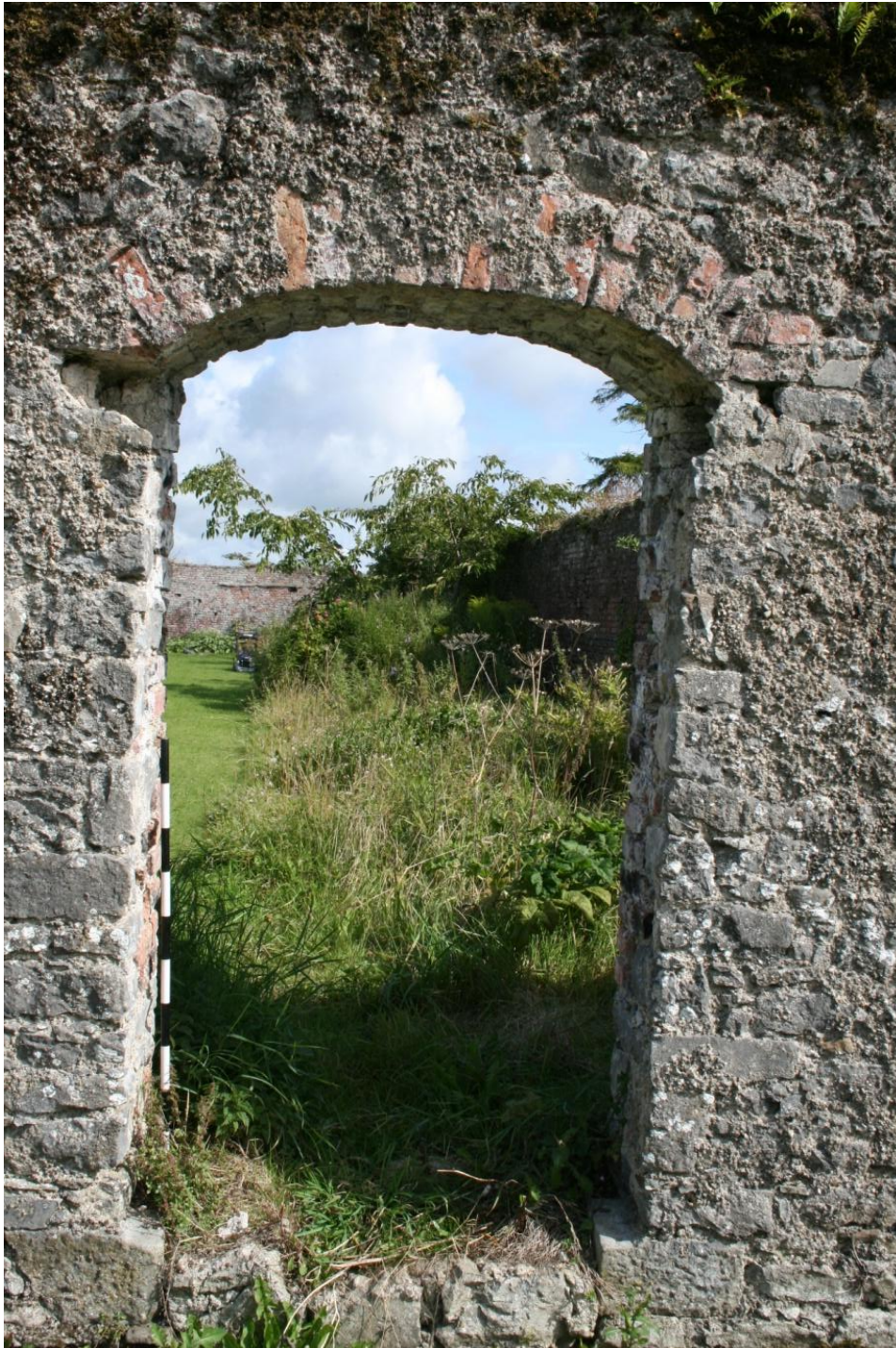
Figure 29: Pedestrian entrance through south wall, at east side.
