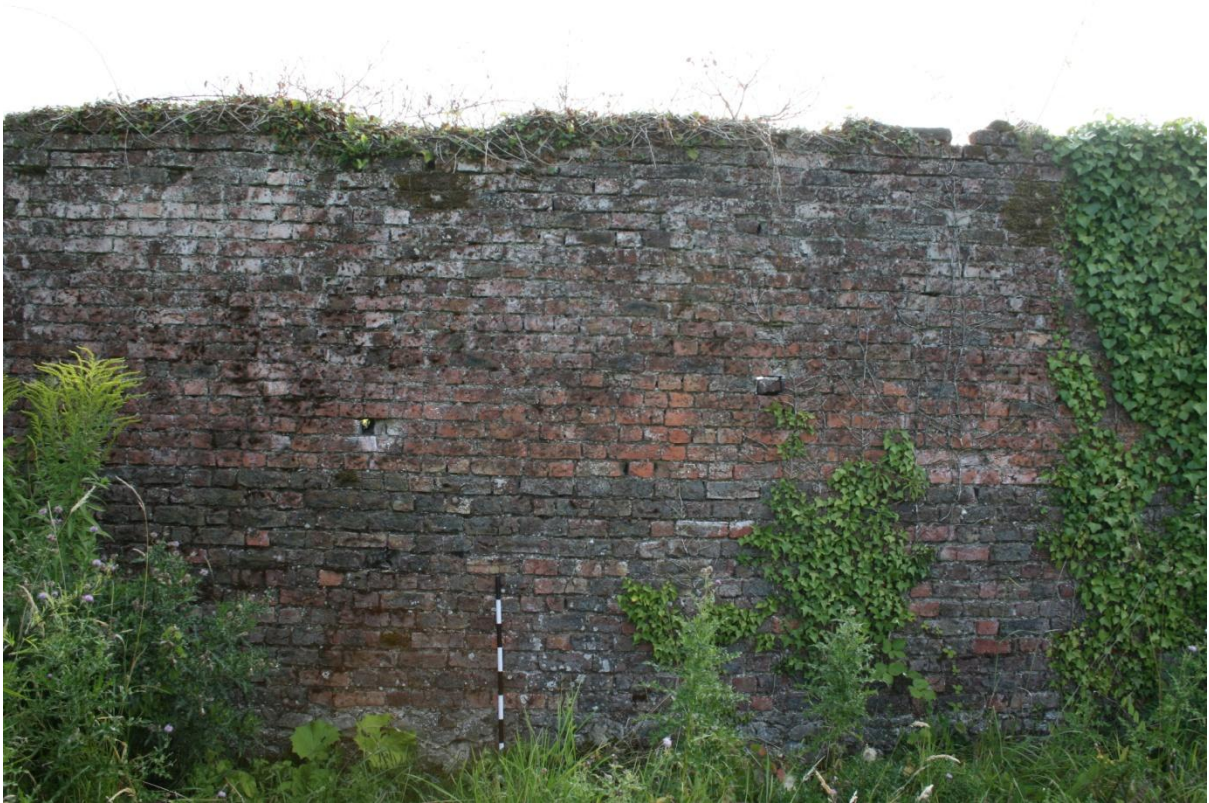
Figure 25: Brick lining above stone courses at base, east wall interior.
