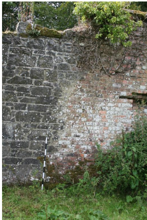
Figure 39: Joint between stone repair and summer house wall, south wall interior.
