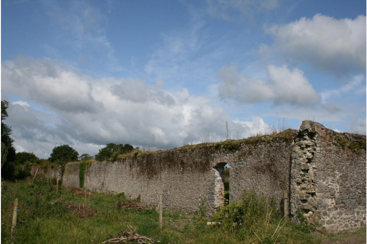
Figure 30: South wall exterior, from south-east.
