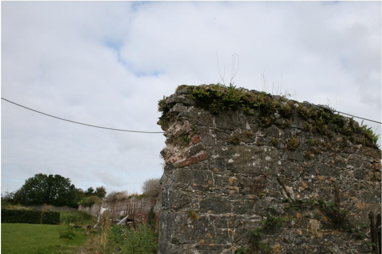
Figure 17: Remains of brick arch to cart entrance
