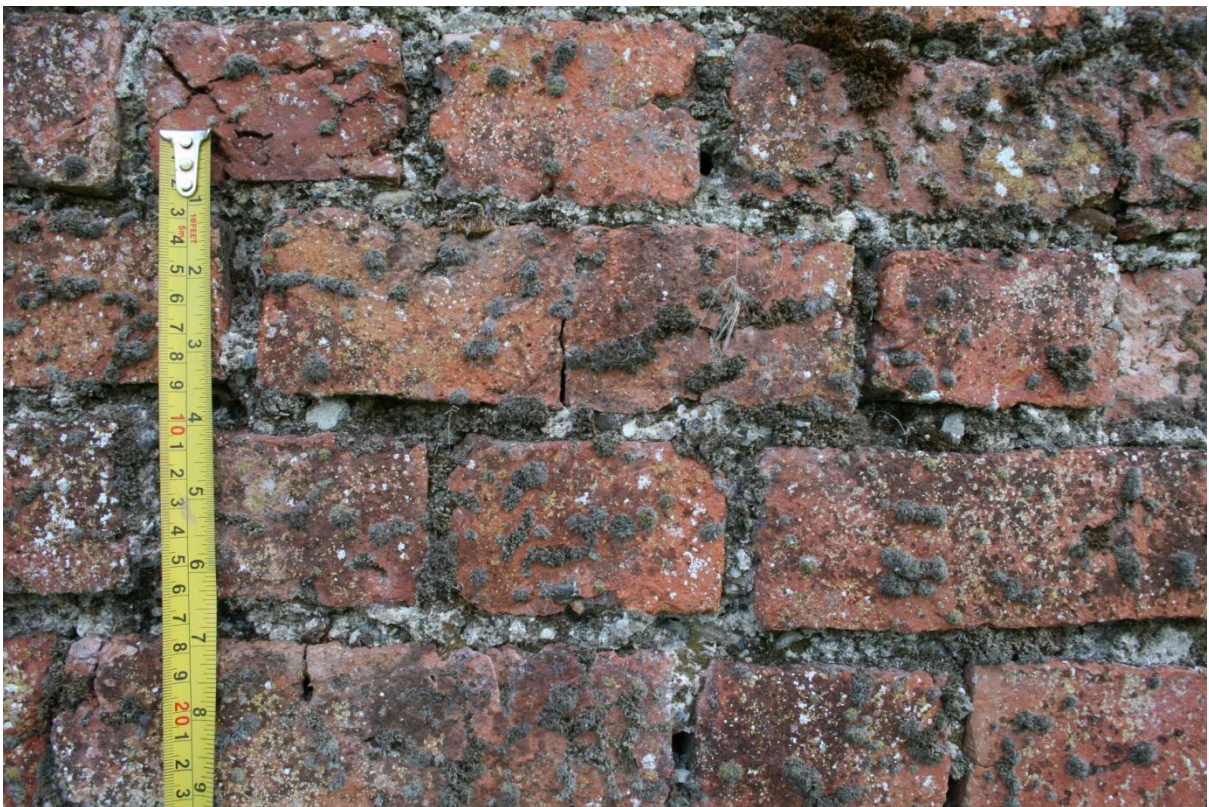
Figure 26: All of the brick is 8 inch x 2.5 inch hand-built, almost certainly of late 18th century date.
