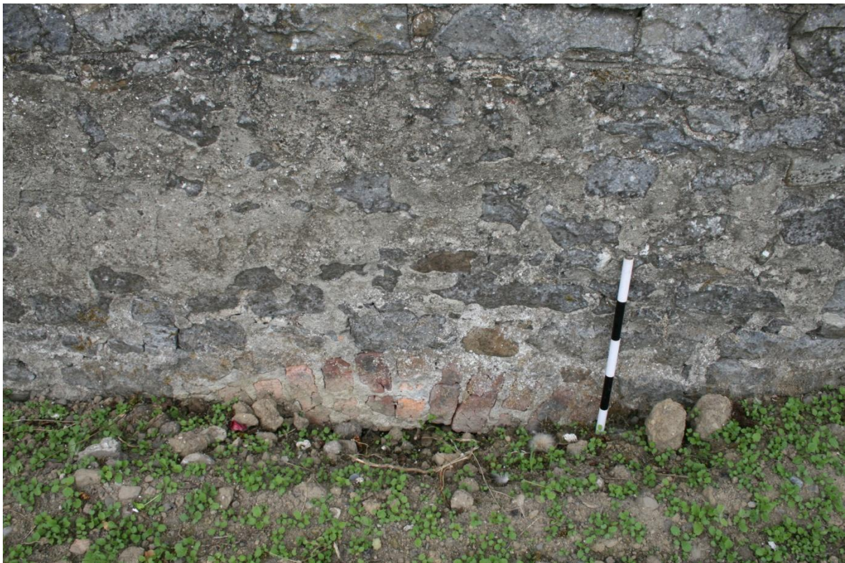
Figure 14: Frost arch at the base of the east wall exterior.
