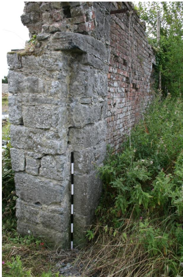
Figure 20: Off-set and spud stone for timber gate at main cart entrance
