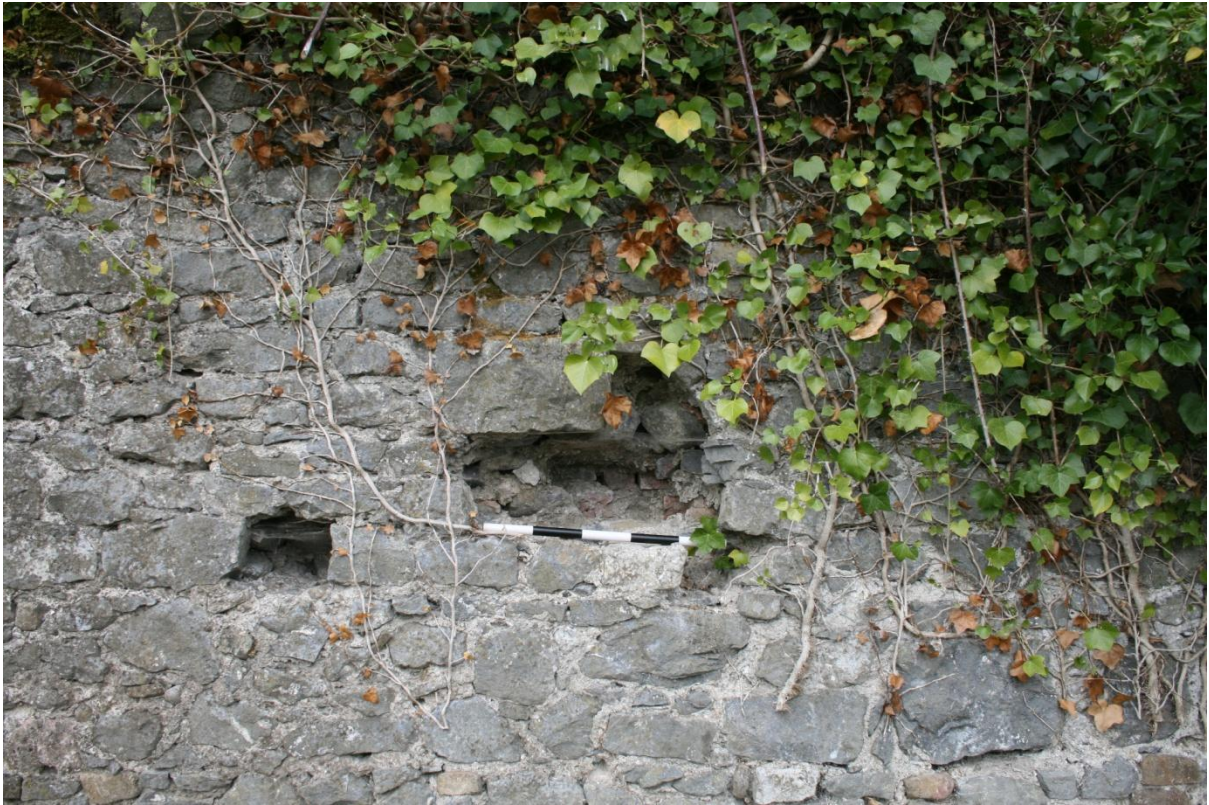
Figure 15: Modern joist holes in the east garden wall exterior.
