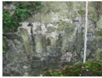
Plate 35. Voussoirs of arch over blocked ope 4.
