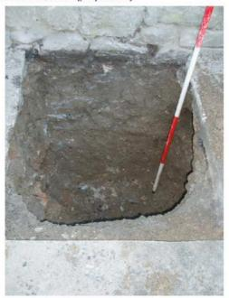
Plate 2. Lower courses of wall F12 in testpit, base of ranging rod sits on earlier masonry.
