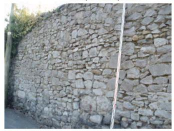
Plate 10. Boundary wall showing at least three phases of building. Upper and middle build are 19th century, lower wall F12 is probably 18th century in date.
