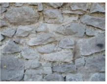
Plate 16. Chipped stone face of 19th century wall.
