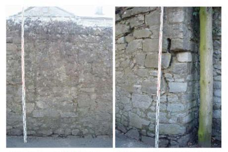
Plate 8. infilled ope in gable wall of barracks.
