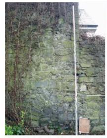
Plate 31. Blocked arch, cut /abutted by later wall.
