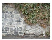
Plate 18. Wall along millrace, showing join of two builds.
