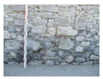
Plate 1. Lower course of wall F12, showing calp masonry.
