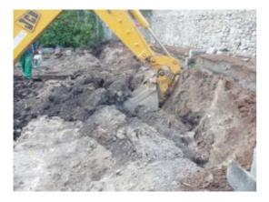
Plate 1. Removal of foundations.
