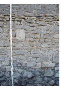
Plate 13. Levels of rebuilding, with reused stone from abbey.
