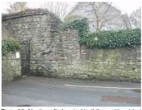
Plate 22. North wall claustral building, with added masonry to west, with brick dressed window.
