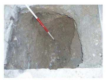
Plate 3. Wall F12 sits on earlier masonry which projects from the base of the wall. Depth 1.32m below street level. Red brick rubble abuts lower face of wall F12.
