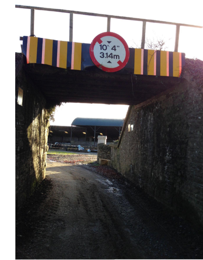
IRISH RAIL OVERBRIDGE WITH STEEL DECK
