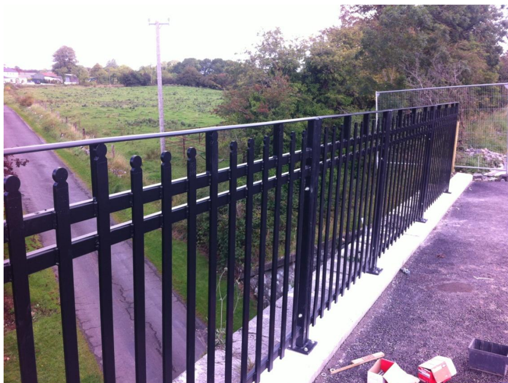
Photo 3.5: New parapet railing provided where there was no existing masonry parapet
