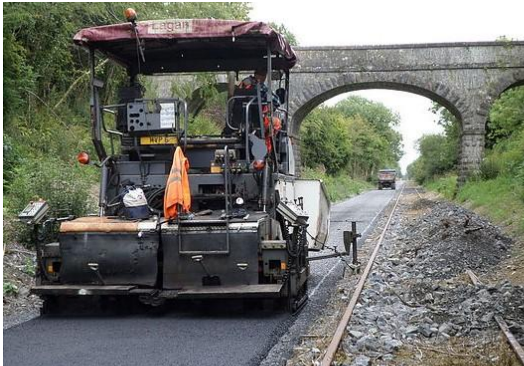
Photo 3.2: Bituminous layer placed using a paver
