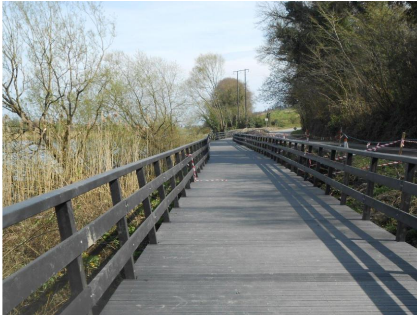
Photo 3.9: Example of a light weight boardwalk/structure (recycled plastic)
