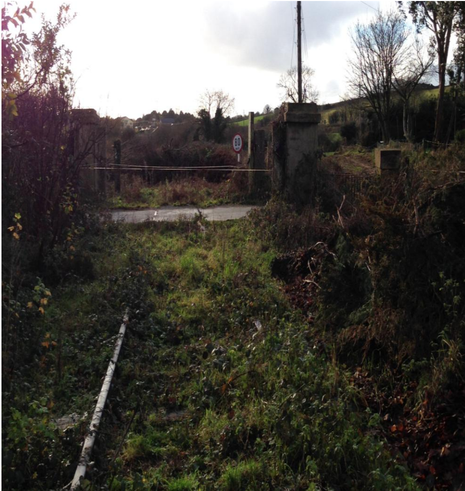
Photo 4.7 Looking south towards level crossing at Ch. 6+610
