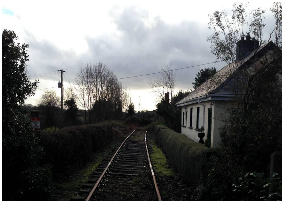
Photo 4.5: Gate house at Level Crossing at Ch. 5+000
