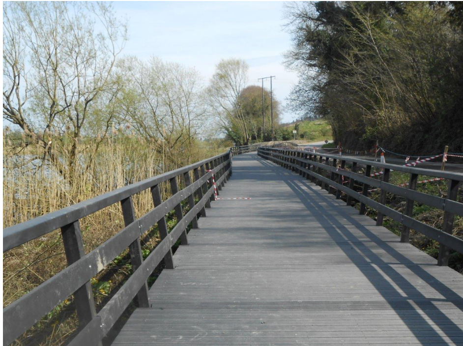
Photo 7.8: Light-weight reinforced plastic board walk on the Boyne Greenway
