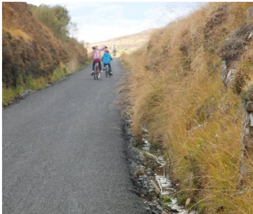
Photo 7.9 - Example of cutting drainage on the Great Western Greenway in Mayo
