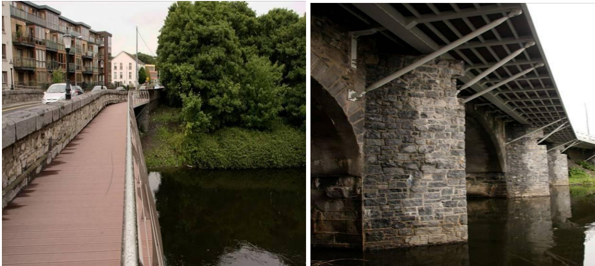
Photo 5.4 & 5.5: Footbridge fixed to existing bridge crossing of the River Liffey in Chapelizod, Dublin
