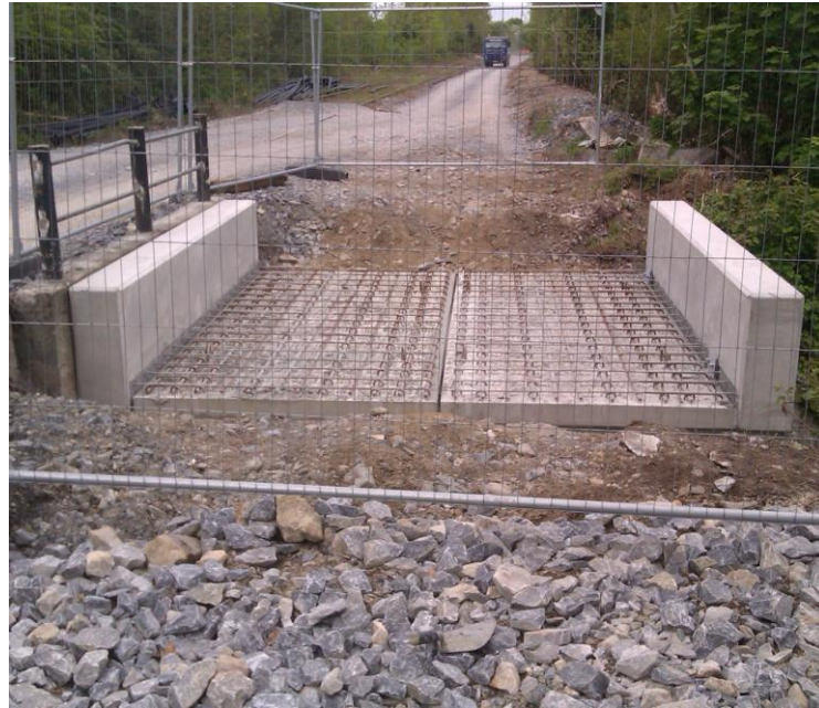
Photo 7.6: Structure UBJ 443 at Ch. 11+760
