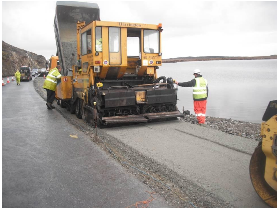
Photo 7.2 - Cycleway Sub-base laid with a paving machine at Derrylea, Co. Galway
