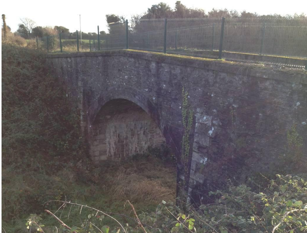
Photo 4.15: Masonry Under-bridge UBJ 437 (Ch. 15+960)
