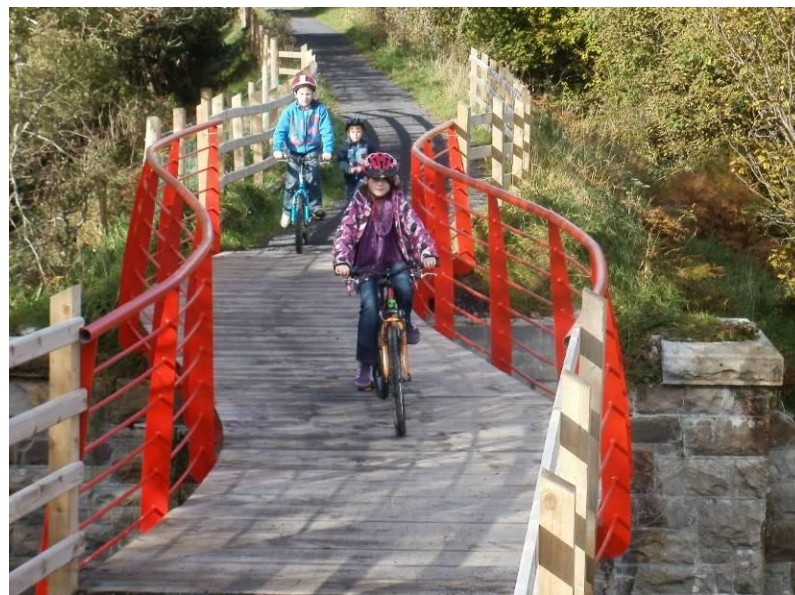
Photo 7.7: Light-weight Bridge Deck on the Great Western Greenway in Mayo
