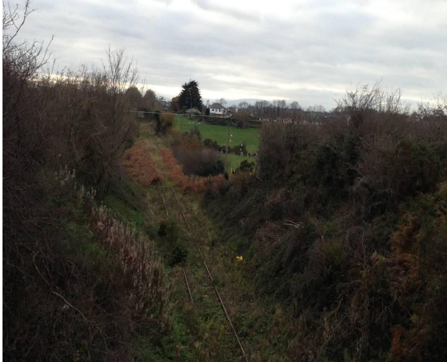
Photo 4.4: Looking south from bridge IR REF: UBJ 460 towards Waterford (Ch. 4+300)
