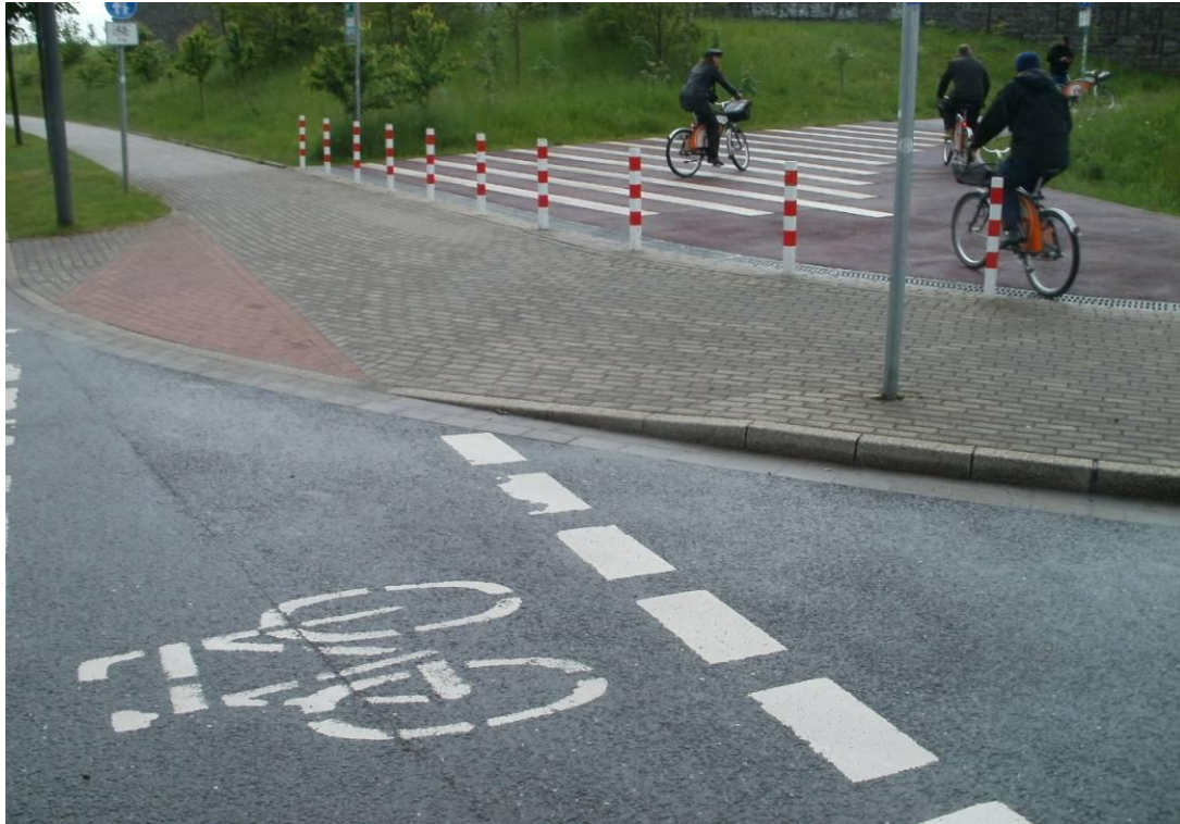
Photo B1: Example of simple Access Control using bollards (Essen, Germany)
