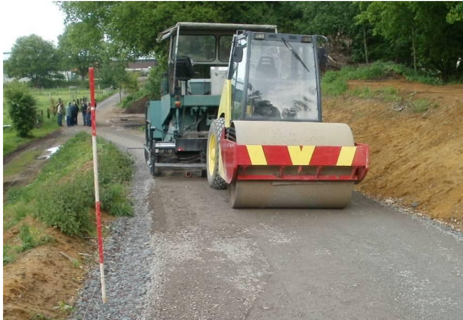
Photo 7.3 - Cycleway Sub-base laid with a paving machine in Germany
