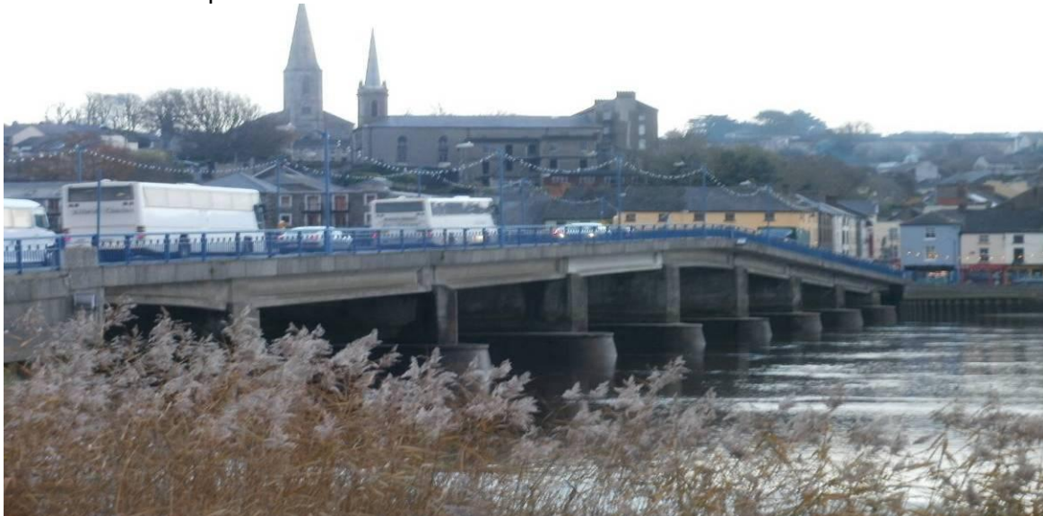
Photo 5.3: O'Hanrahan Bridge crossing into New Ross
