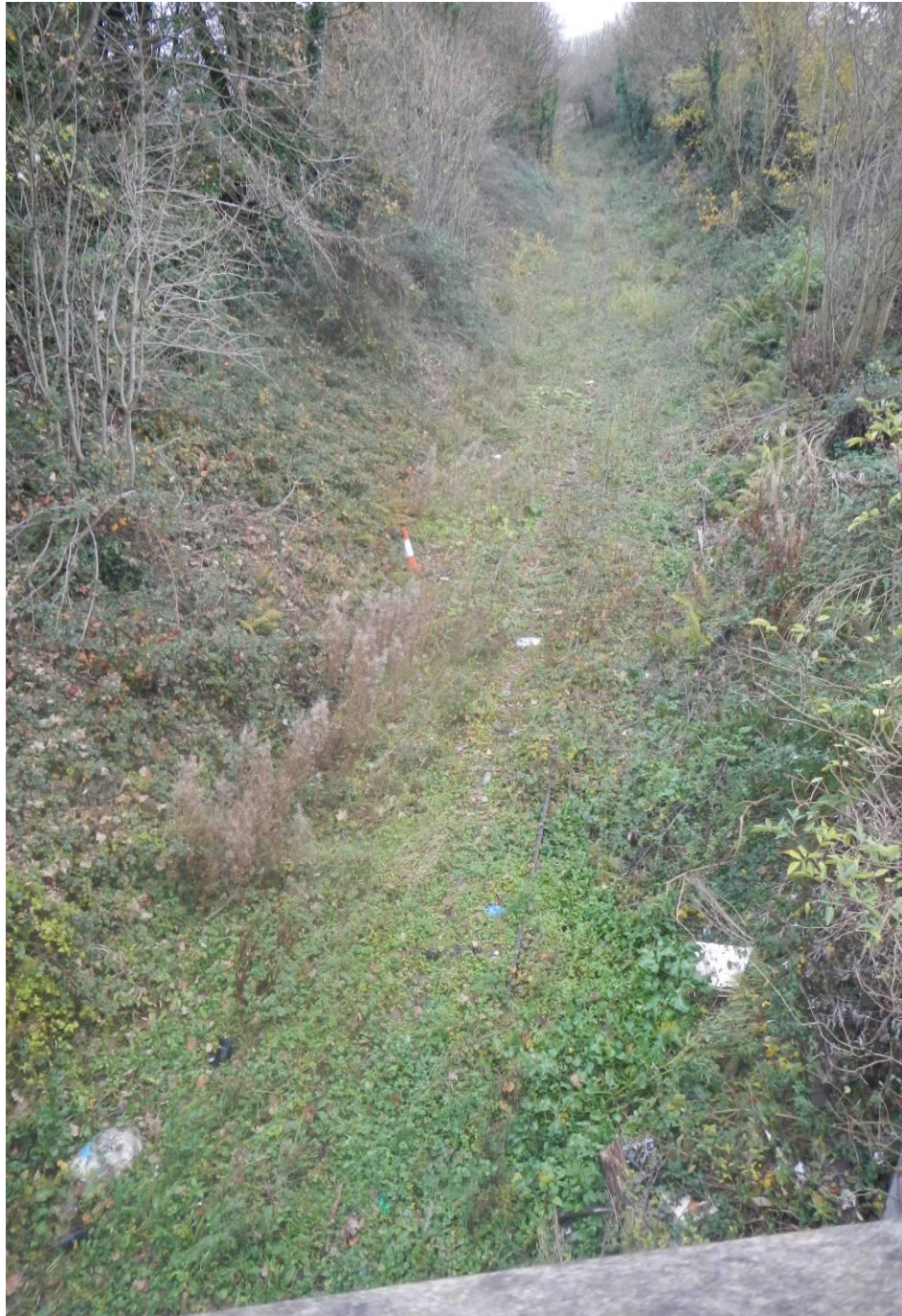
Photo 4.1: Looking north from bridge OBJ 470 in Ferrybank (Ch. 0+000). Adjoining houses screened by vegetation.
