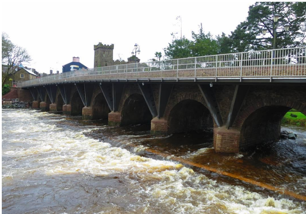
Photo 5.6: Footbridge fixed to existing bridge crossing of the River Sullane in Macroom, Co. Cork
