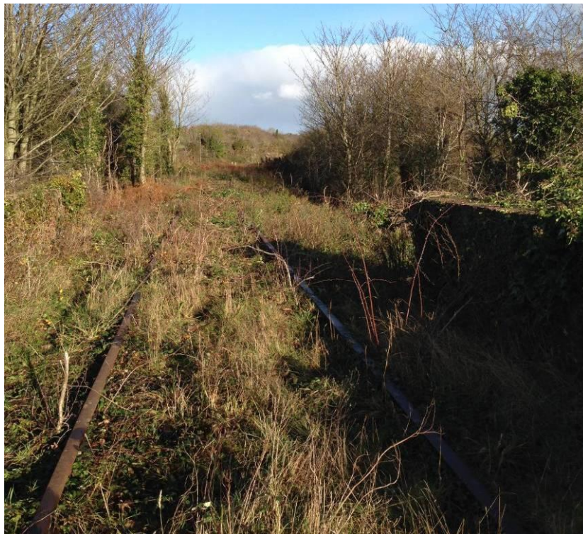
Photo 4.11: View from bridge deck at Ch. 11+230 (IR REF UBJ 444)
