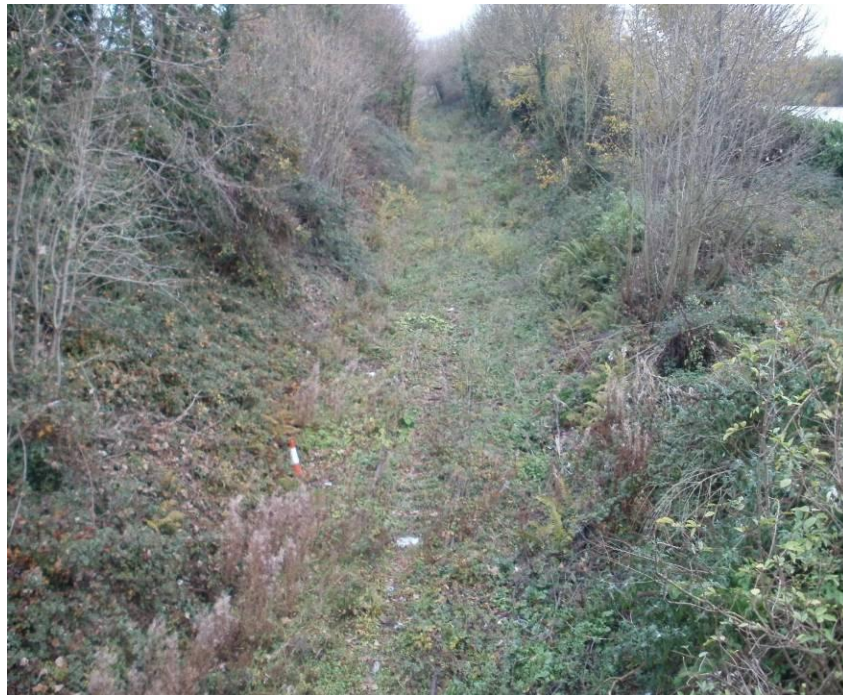
Photo 5.2: Looking north from OBJ 470 towards possible location of ramp
