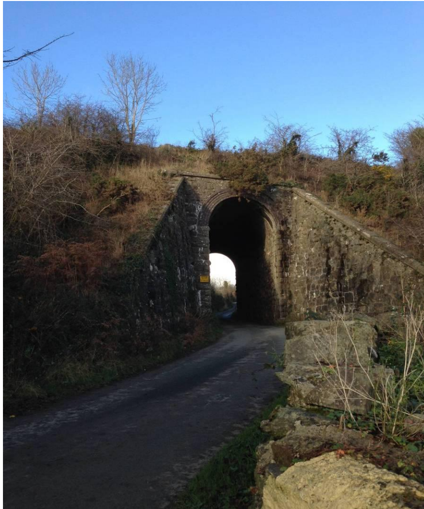
Photo 4.10: Railway Corridor on embankment at Ch.10+380 (IR REF UBJ 447)
