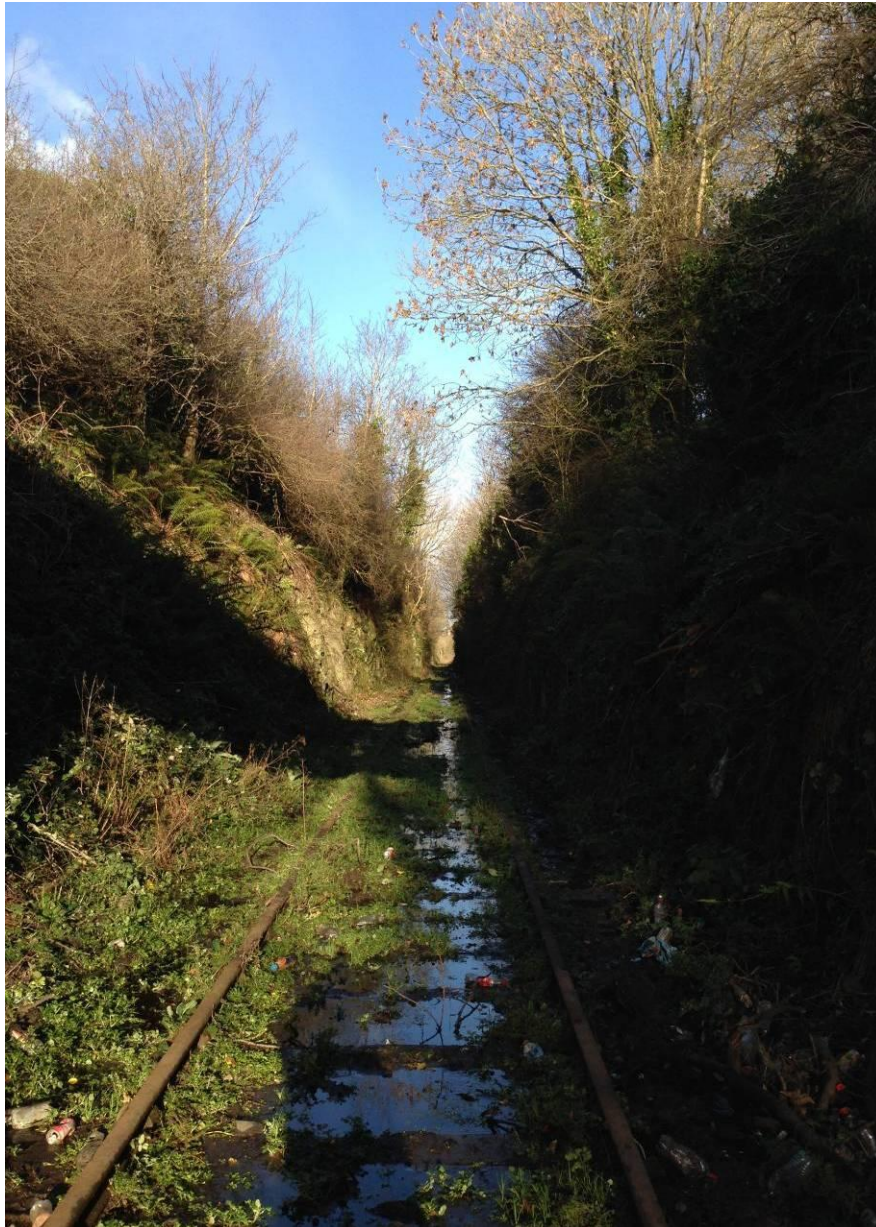
Photo 4.9: Area of rock cutting at Ch. 7+600
