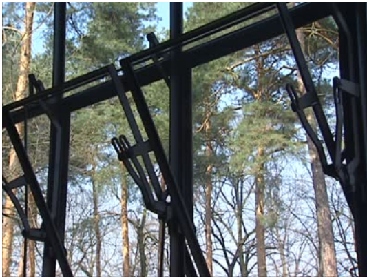
Feininger House, Dessau Germany Walter Gropius mechanically open and close steel windows
