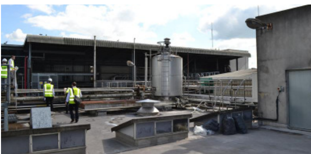
EXISTING BREWHOUSE ROOF SCAPE
