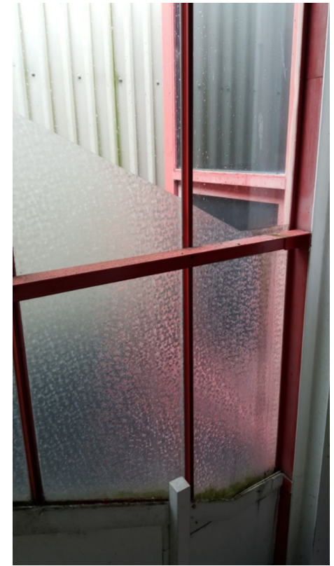
The original window frame: Note the celebration of the joint and the exaggerated shadow gap
