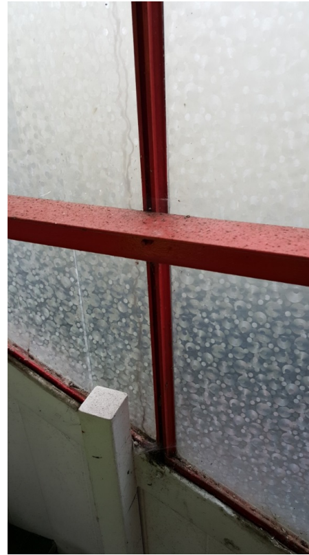
The original window frame: Note the celebration of the joint and the exaggerated shadow gap
