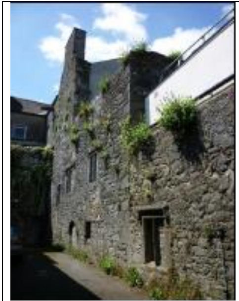
Plate 10 Rear of No 40 Parliament St (along Horse Barrack Lane), the location of the Red Lion Inn, showing 16-18 th century mullioned windows, facing west.
