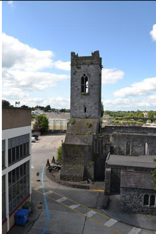
Plate 8 St. Francis Abbey and north-eastern end of Brewhouse building, facing north
