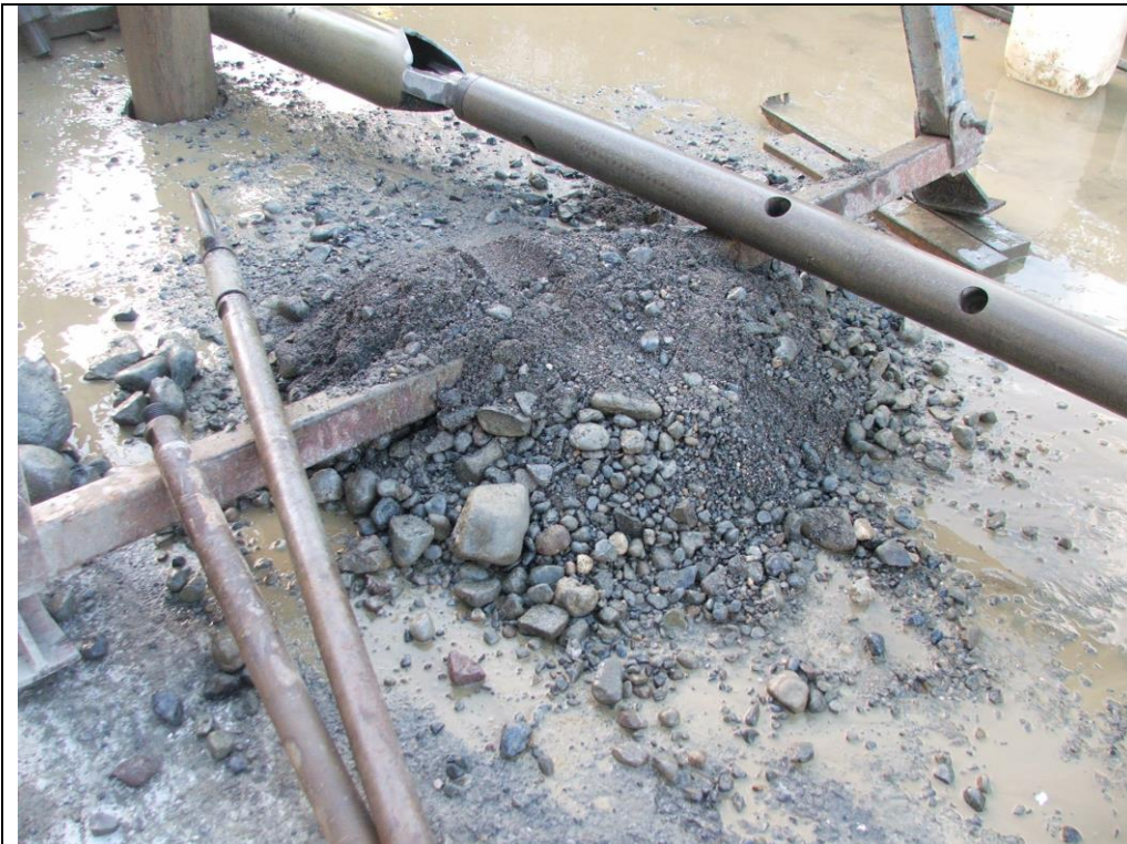
Plate 14 Showing grading soils and stone hardcore from geotechnical sampling in yard to west of Brewhouse building.
