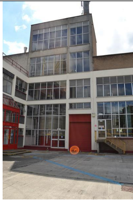
Plate 6 South end of Existing Brewhouse building, facing east
