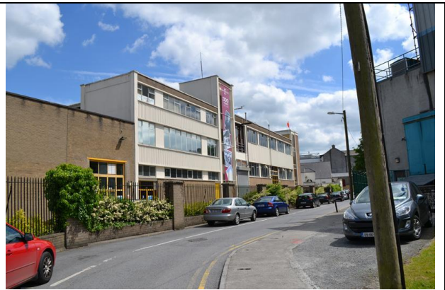
Plate 2 Western side of Existing Brewhouse building from Horse Barrack Lane, facing southeast
