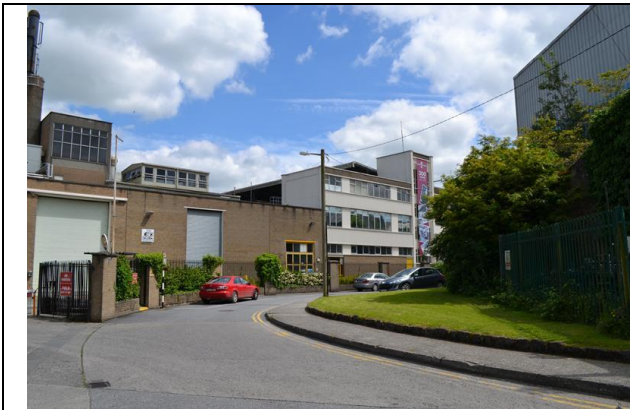
Plate 1 Existing Brewhouse building from Horse Barrack Lane, facing southeast
