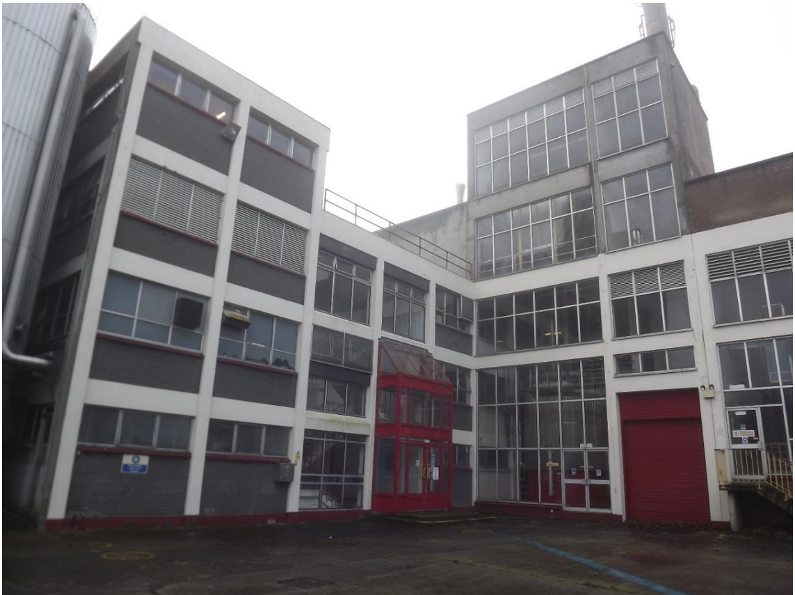
The regular structural grid of the concrete frame
