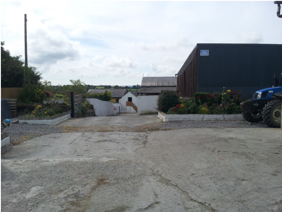
Image 1 – Location of crossing at chainage 12+080
