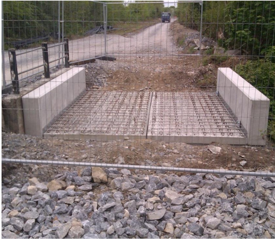
Photo 3.3: Example of new bridge deck placed over existing bridge abutments
