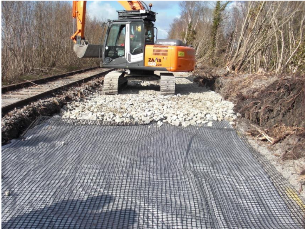
Photo 3.1: Geotextile laid under the Greenway foundation
