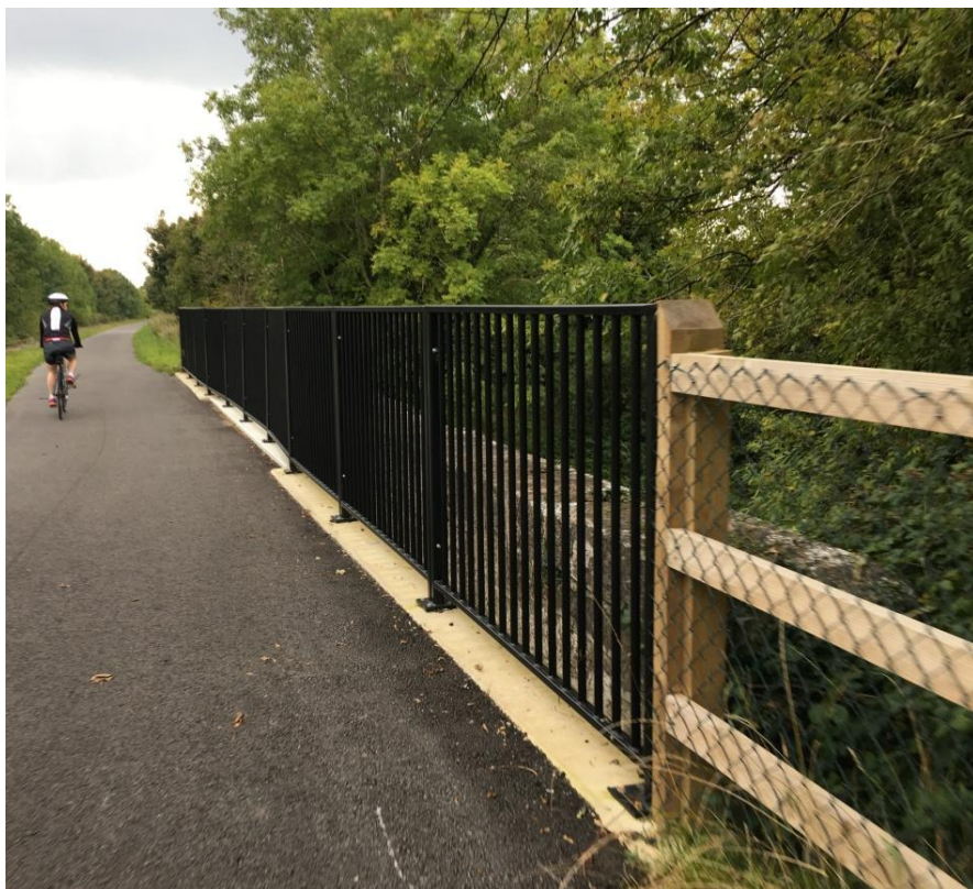
Photo 3.4: New parapet railing placed in front of low bridge parapet
