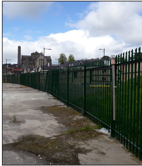
Figure 10 Existing Palisade fence, with timber fence in the background, along boundary with the Central Access Scheme / St Francis Bridge
