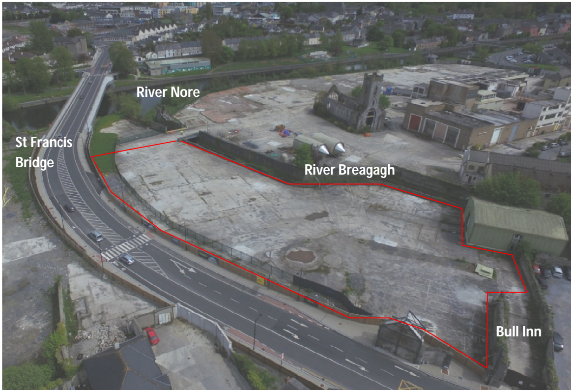
Figure 5 Current Aerial View of the site of the proposed development
