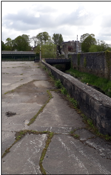
Figure 9 Low level boundary wall along the River Breaghagh
