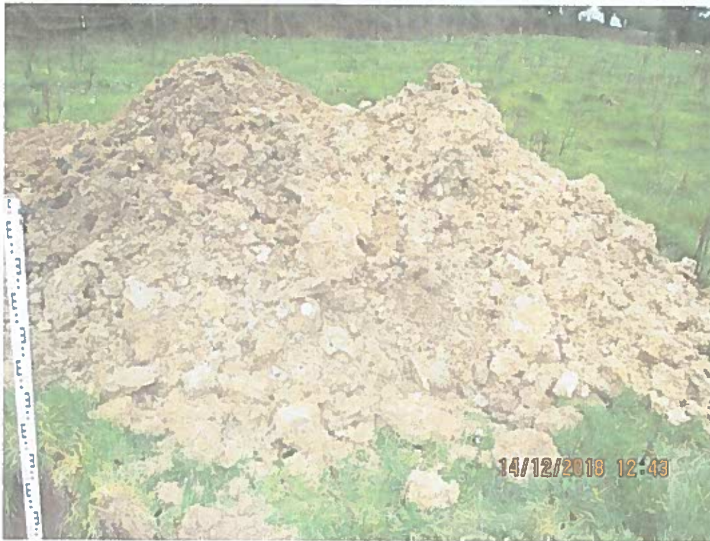
SOIL/SUBSOIL FROM EXCAVATED TRIAL HOLE
