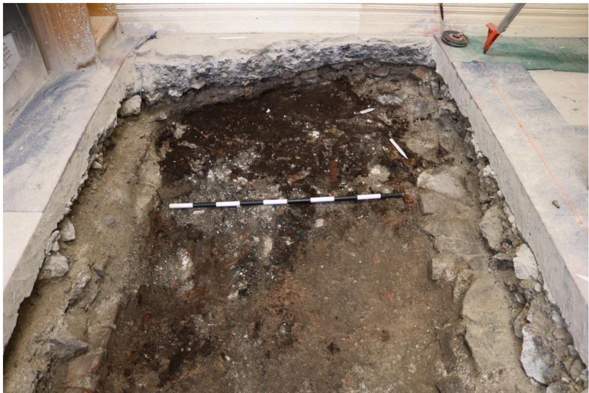
Figure 47: The remains of the mid 20th century fuel store 096, from the east
