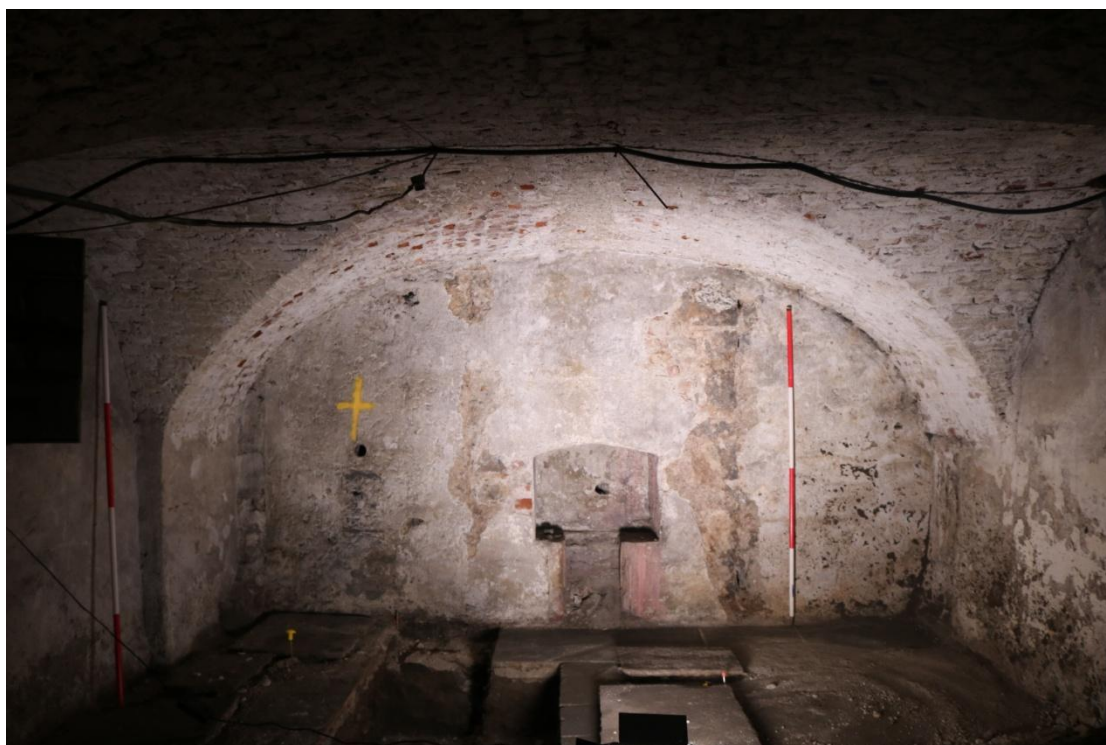
Figure 71: West facing elevation of east basement wall, southernmost bay
