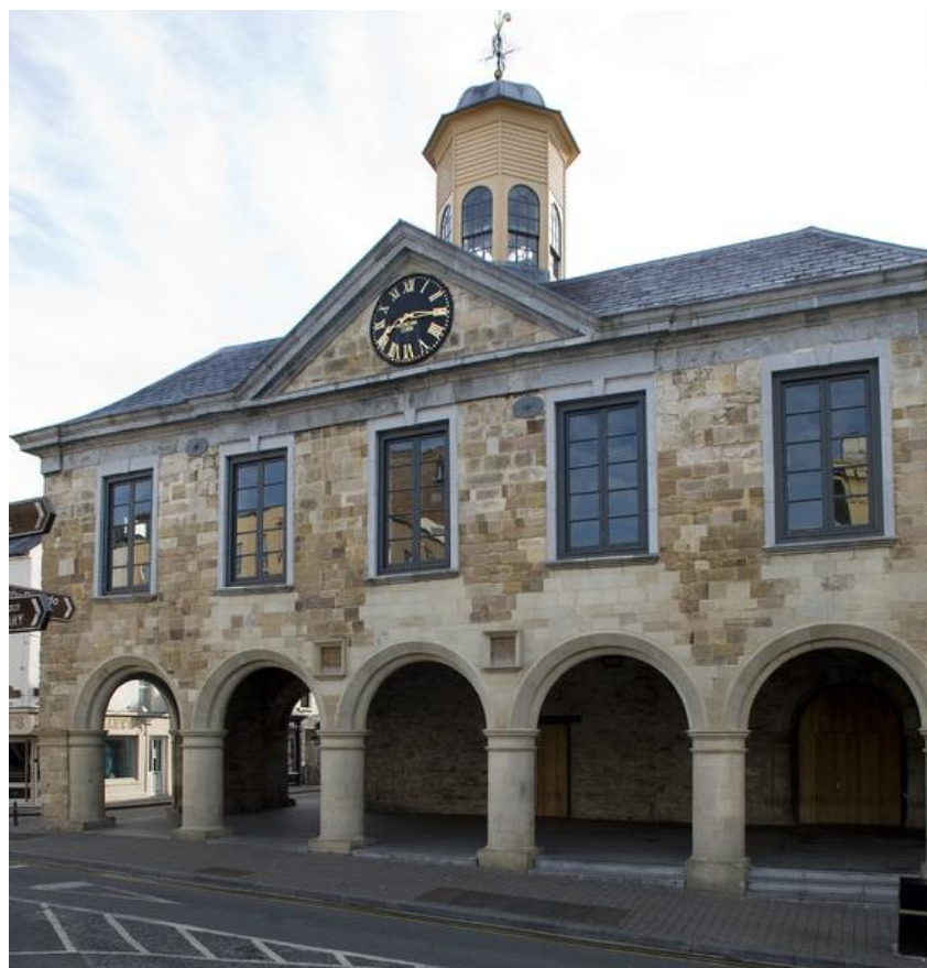
Figure 76: Main Guard, Clonmel, built 1675
