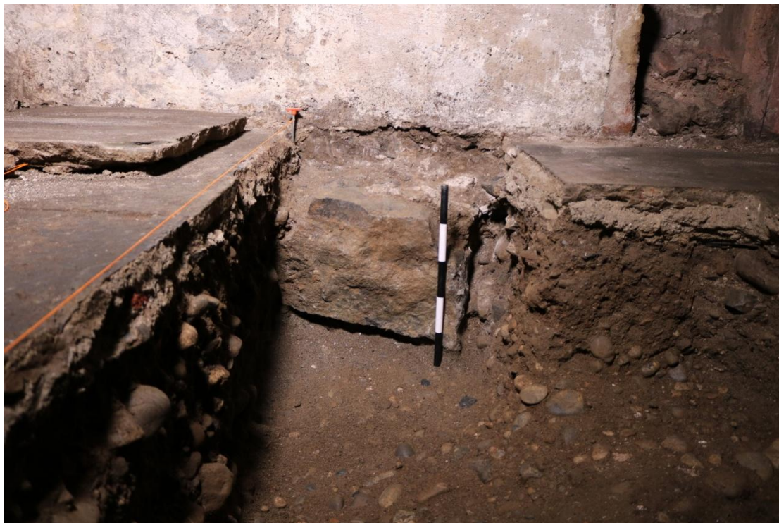
Figure 65: Medieval wall foundation 024 below wall 047 and resting directly on the natural 018, from the west
