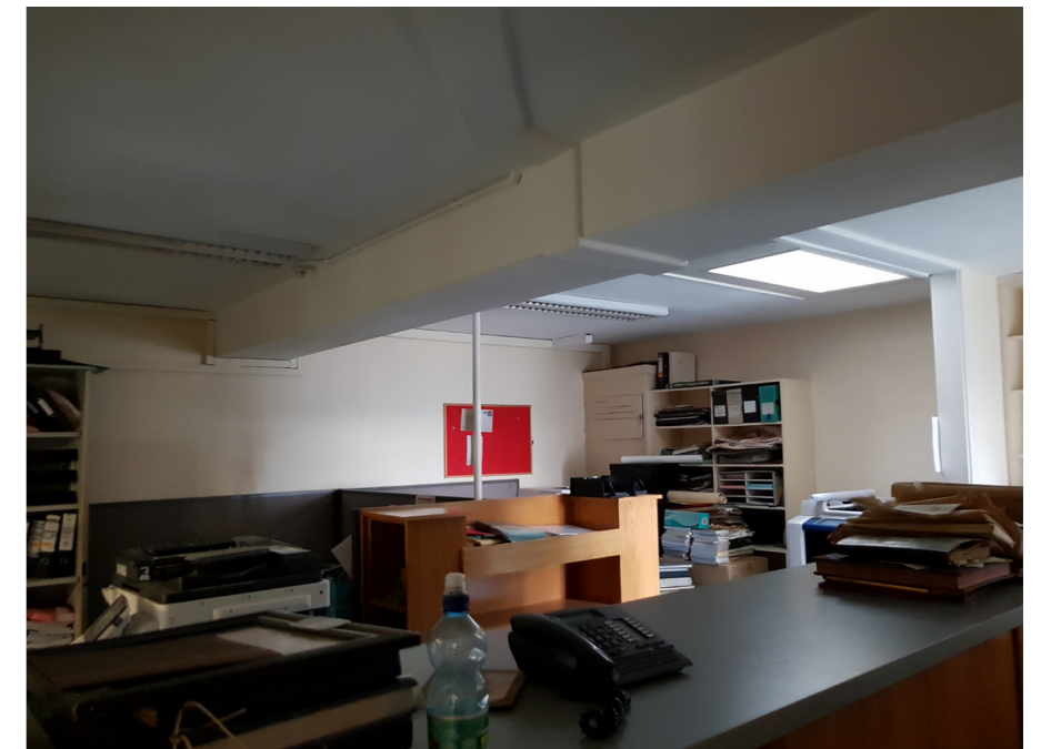
Third floor mezzanine: Office
