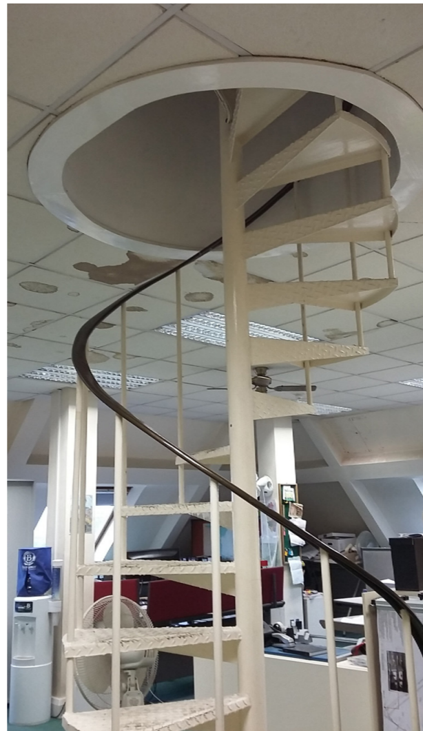
Fourth floor: Spiral stair to Cupola
