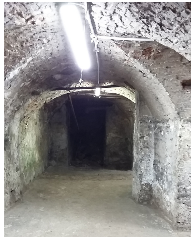
Basement: Brick vaults looking South
