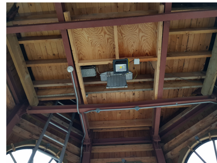
Cupola: Looking up towards bell chamber
