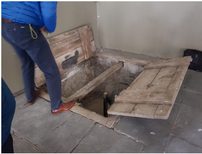
Current trapdoor access to basement from arcades
