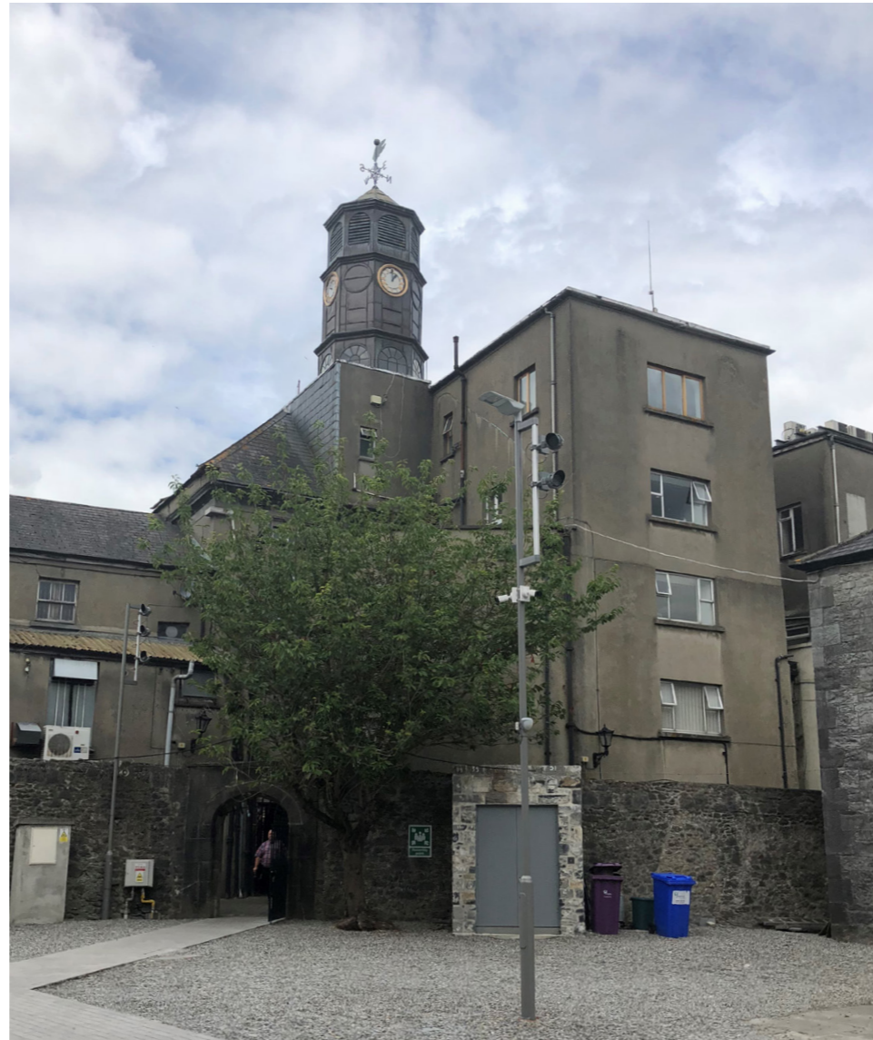
Existing building photographed in 2018
