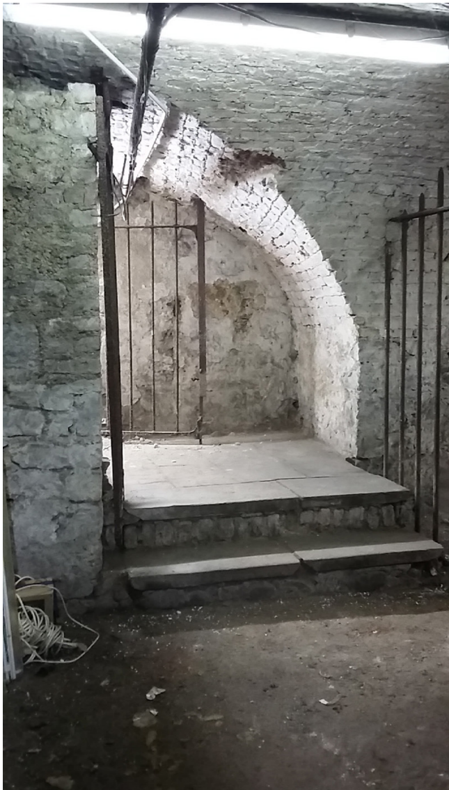
Basement: Steps to trapdoor
