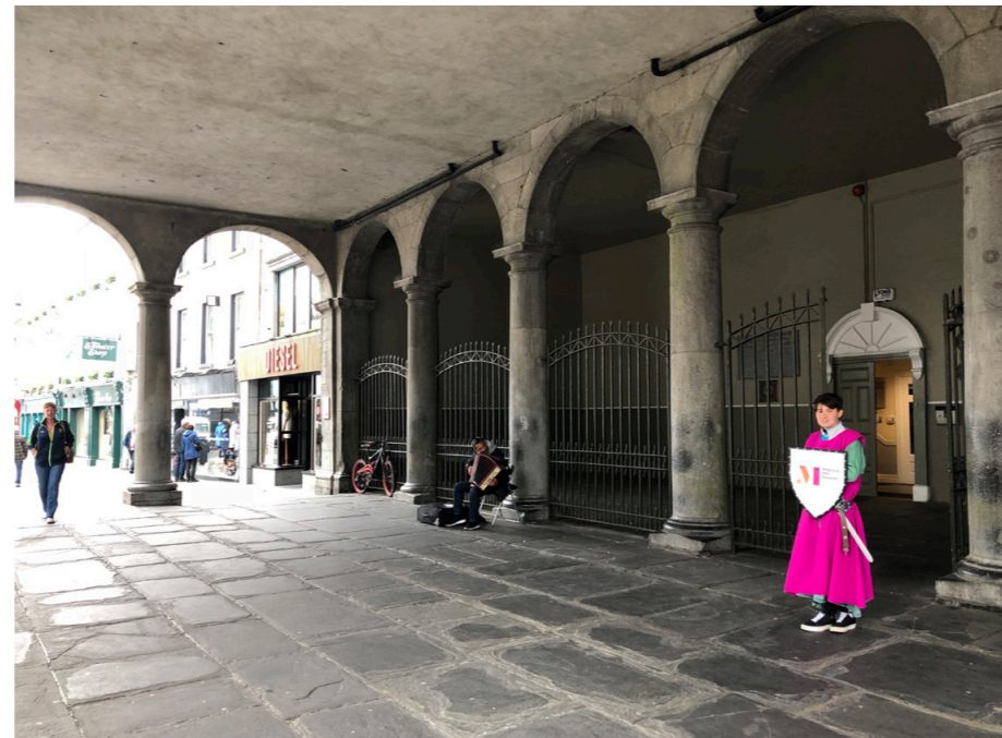
View of arcades and railings
