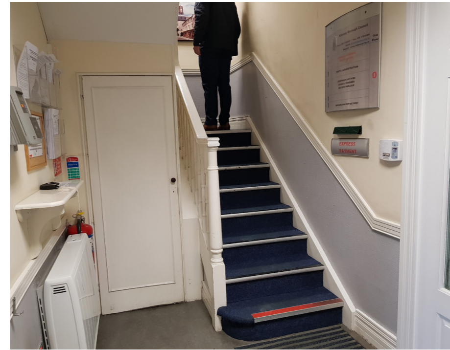
Staircase in ground floor return
