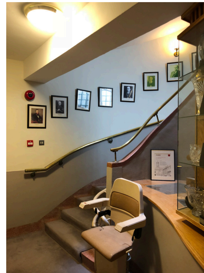
Ground floor: Ceremonial Staircase
