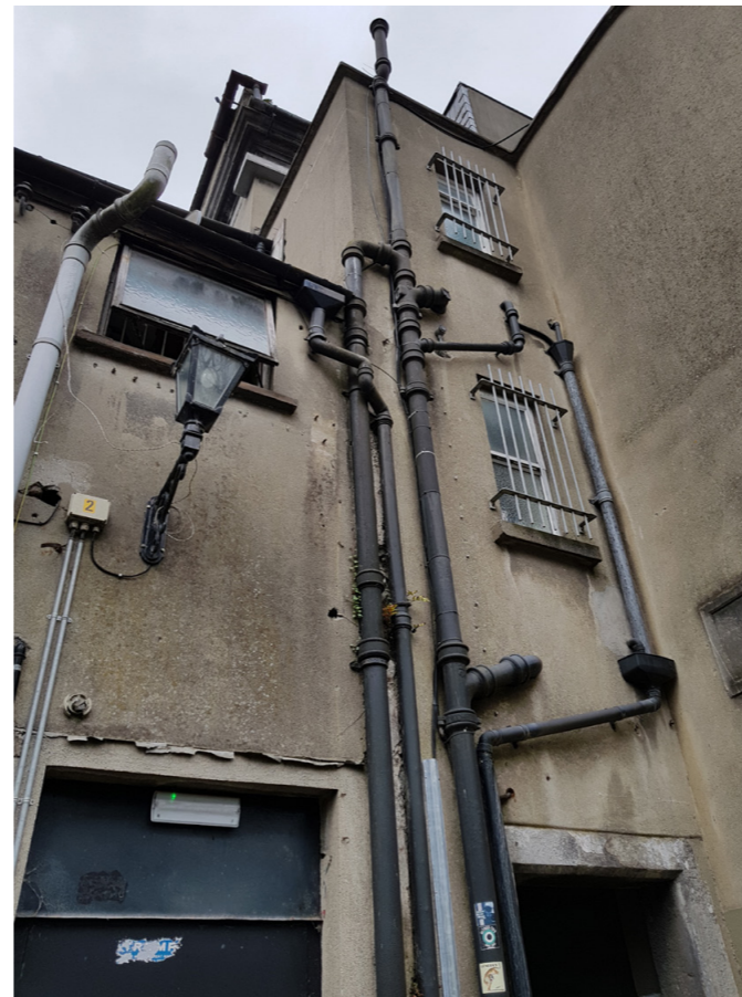
Part of rear facade from St. Mary's Lane
