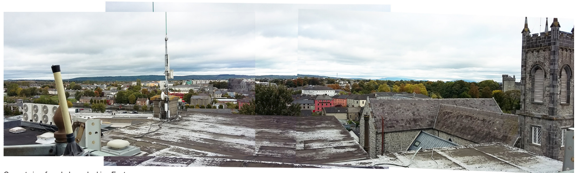
Current view from balcony looking East
