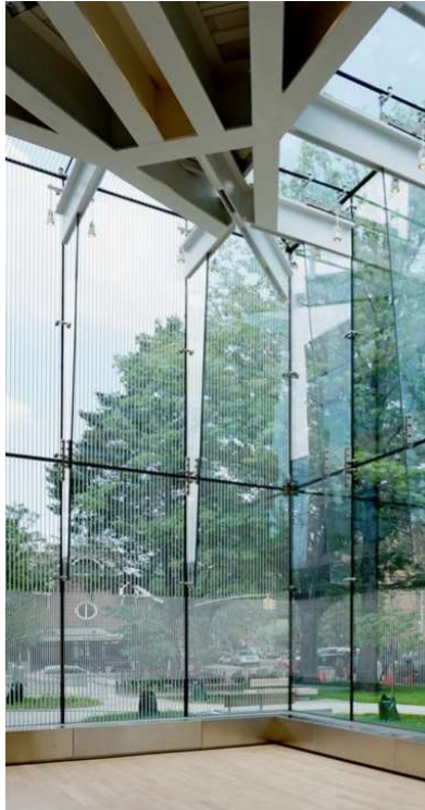
Figure 2. Discreet Lighting within a glazed structure
