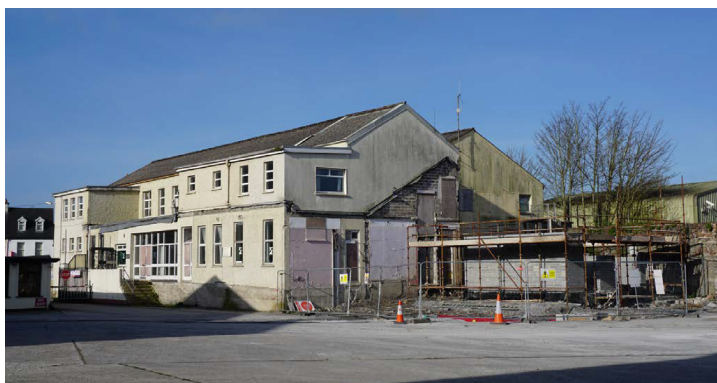
Figure 9: View of Existing Building from St. Francis Abbey (East)
