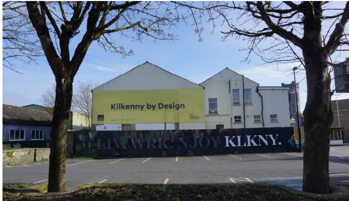
Figure 7: View of Existing Building from Parliament Street (West)
