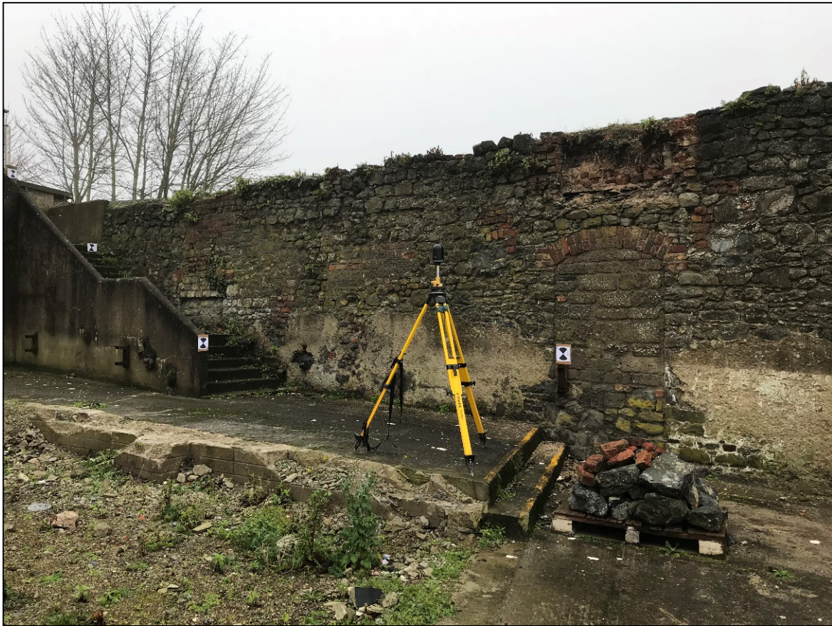
Plate 9 Laser scan of the city wall in progress
