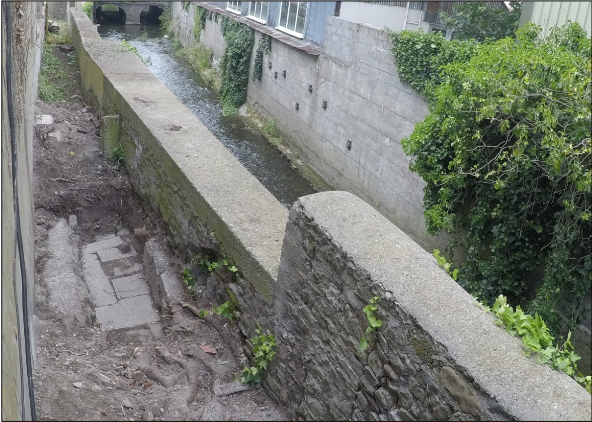
Plate 6: ACSU Test Trench 10:2, looking west, along the narrow space between the Mayfair Building and the city wall National Monument
