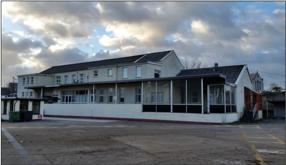
Plate 1: Mayfair Building in 2017, looking north before demolition works
