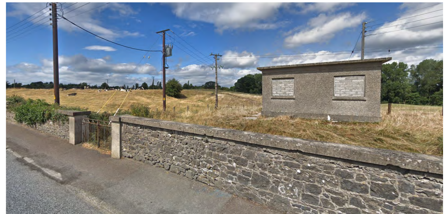
View looking North across site from Kennyswell Road
