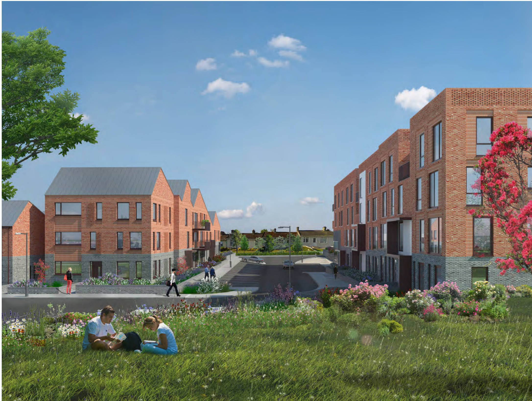
View looking South towards Kennyswell Road from the Public Open Space
