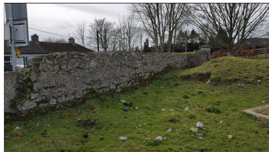
Plate 8: Intact section of wall (opp. nos 13, 14 and 15 Circular Rd)
