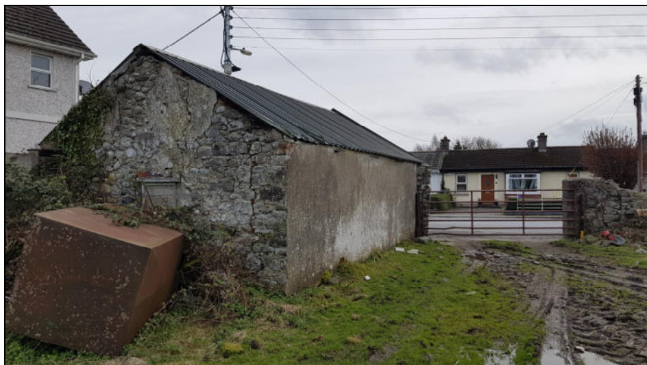
Plate 5: Shed in SE corner of site along Circular Rd
