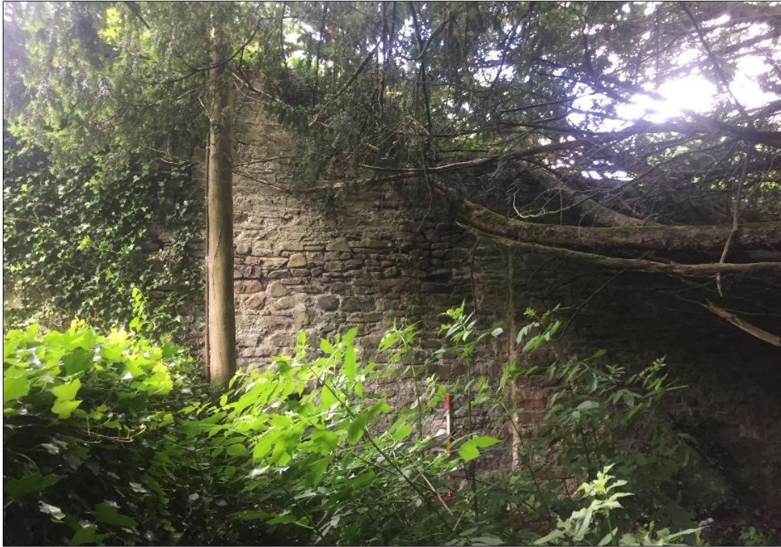
Plate 29: North elevation of west abutment with small step visible in wall just right of ranging rod. ESB pole left of centre is at corner where the river-bank wall abuts wing wall of bridge. No evidence of a structure having existed was uncovered during the inspection
