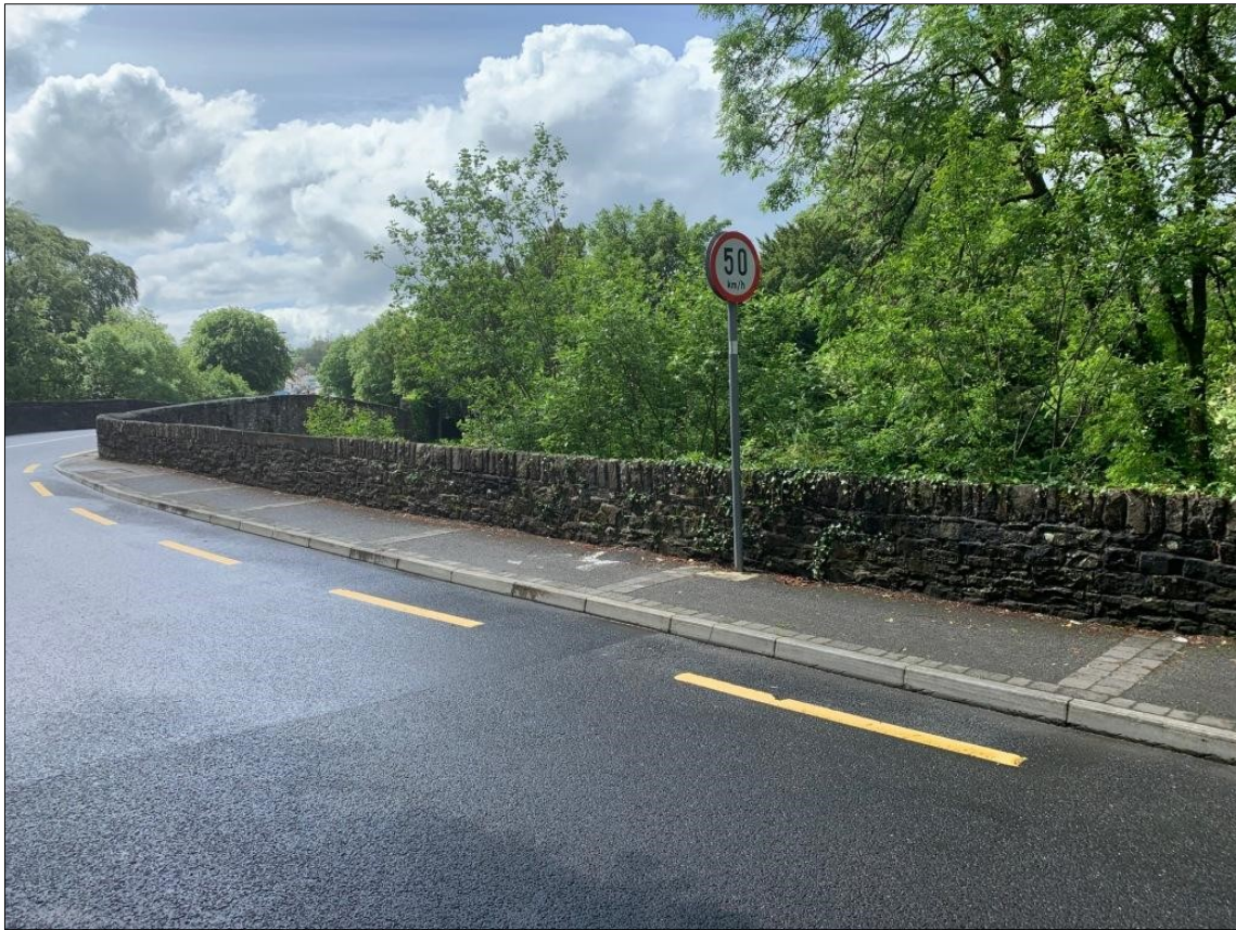
Plate 39: View from east of the roadside wall on the north-east approach to bridge. A new opening is proposed to provide the eastern approach footpath to the new footbridge. This wall appears to have been consolidated with concrete in recent years and the vertical coping stones which only face onto the roadside place at the same time.
