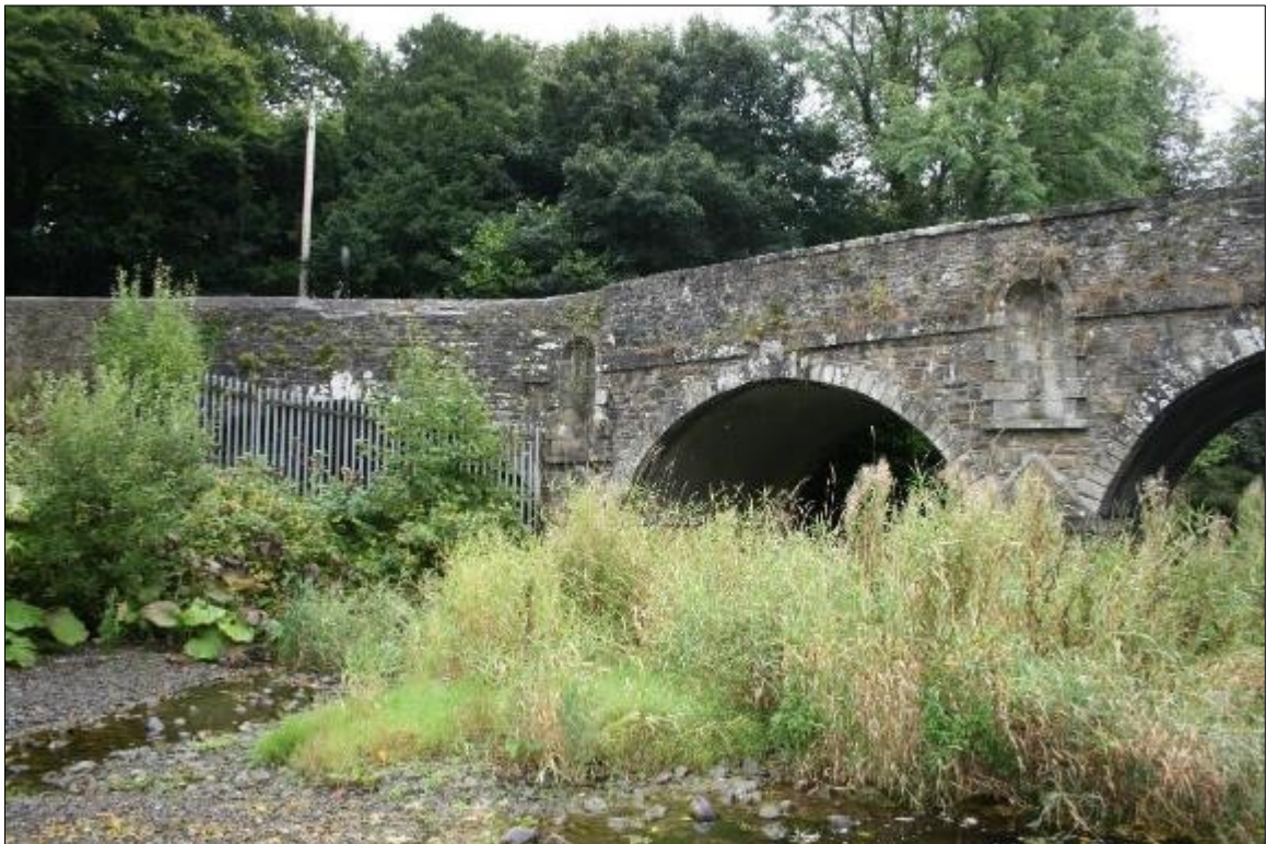
Plate 12: East half of north elevation
