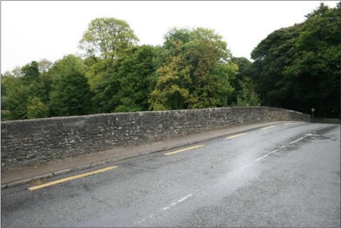
Plate 3: Detail of inner face of the north parapet wall
