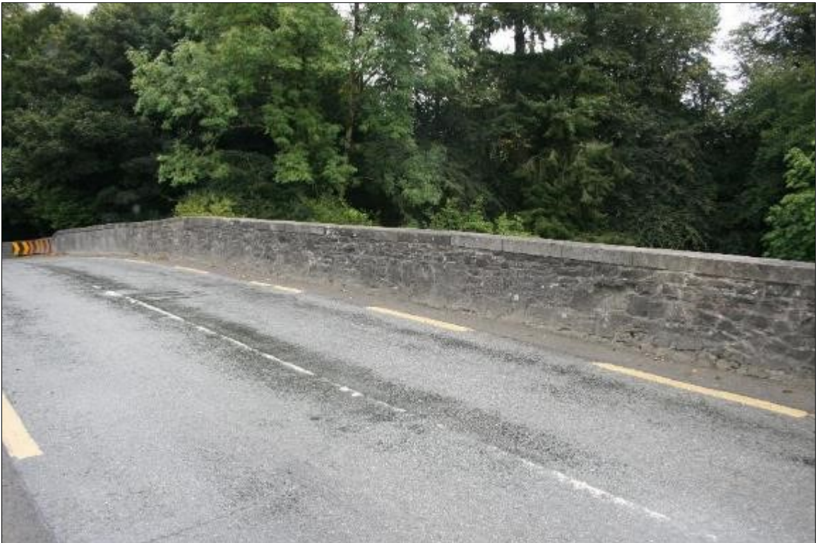
Plate 4: Detail of inner face of the south parapet wall
