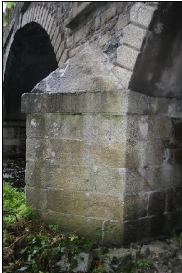
Plate 22: Detail of downstream cutwater on south elevation
