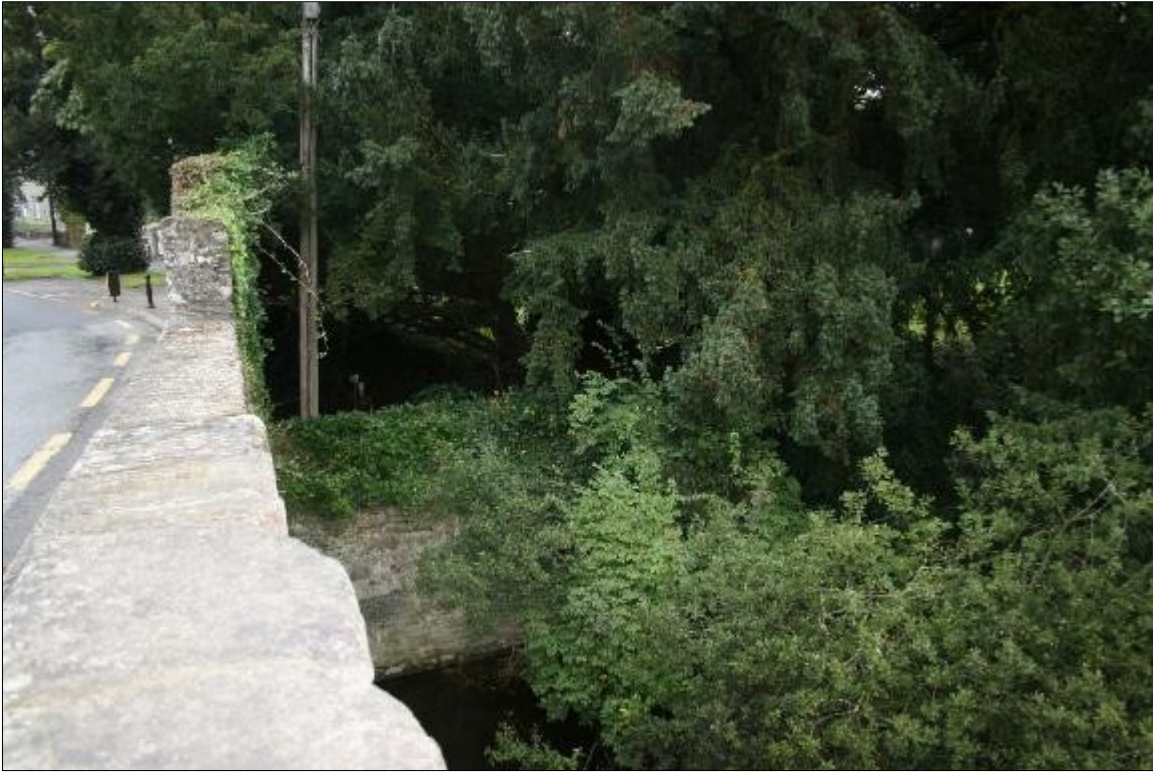
Plate 7: West abutment from north parapet of bridge; the garden area behind this riverside section is associated with La Rive, an end-of-terrace house and protected structure. The western landing area for the proposed pedestrian bridge will be accommodated in this location.
