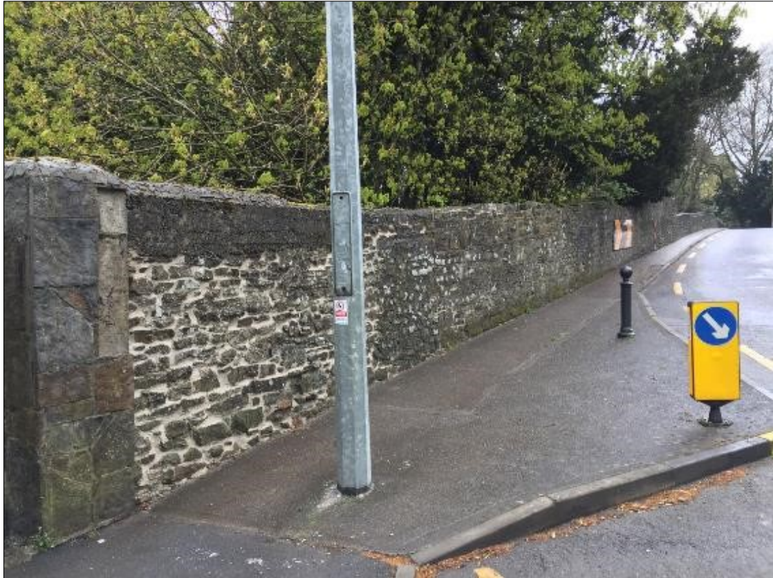
Plate 25: View from west of the roadside frontage of the garden area of La Rive – the closest wall section is clearly rebuilt and incorporates a portion of cast-concrete capping
