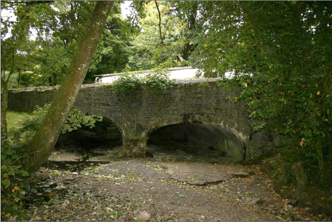
Plate 41: North-west openings of skewed archways carrying N78 over watercourse approximately 50m east of main bridge structure. The base of the new footbridge is to be positioned to the west
