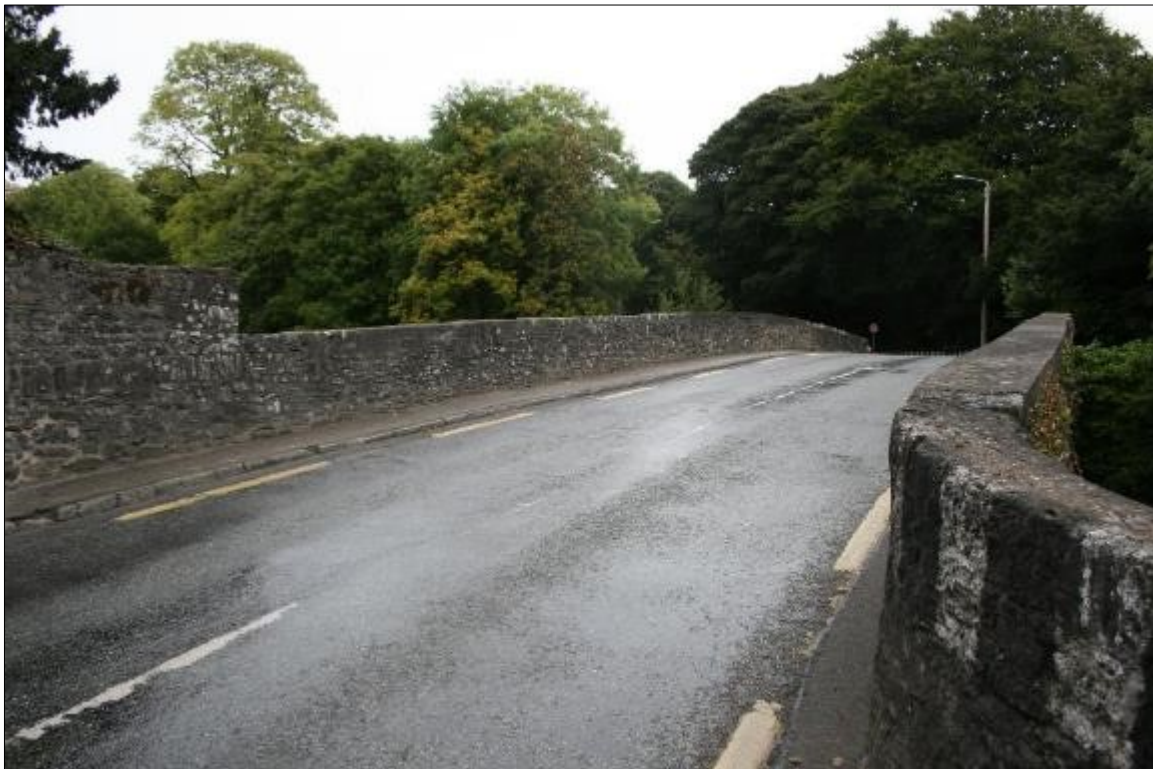
Plate 2: View over road deck from south-west corner
