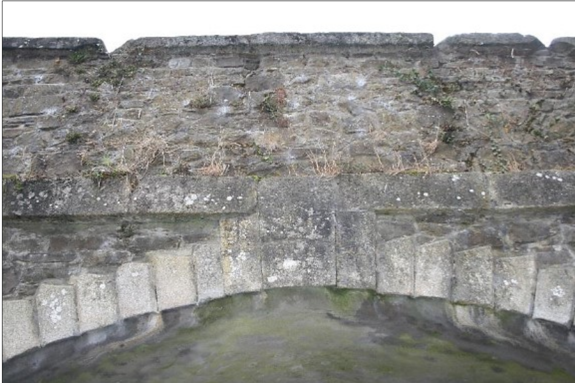
Plate 15: Keystone, voussoirs, string course and exterior parapet detail over 2 nd arch from west abutment
