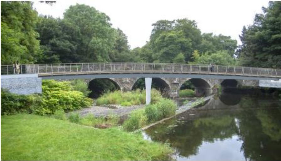
Figure 3-1: Two Span Steel Footbridge Elevation (North)
