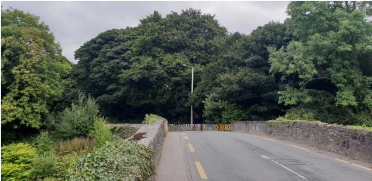
Figure 2-1: View Eastwards along existing N78 Carriageway crossing the Castlecomer Bridge
