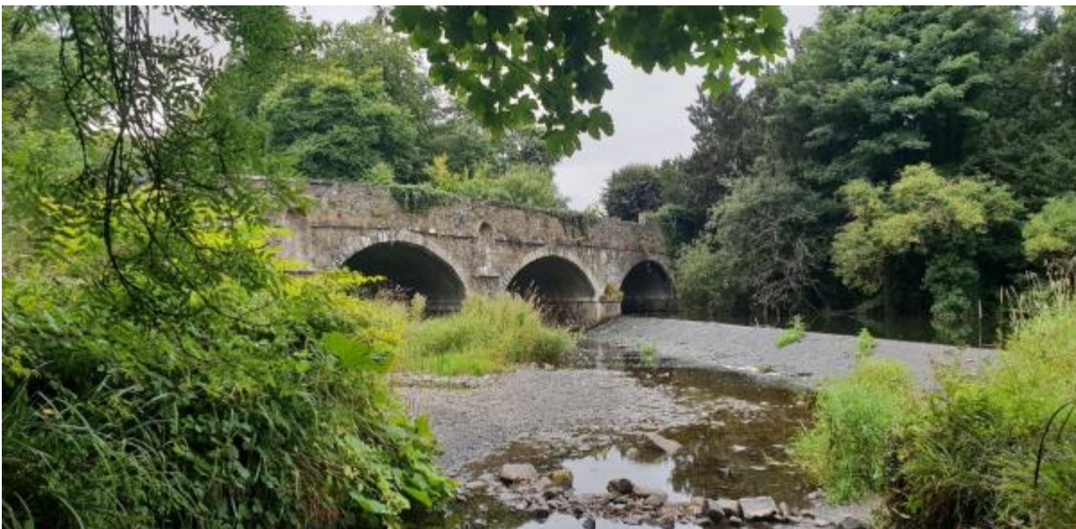
Figure 1-1: Elevation of North Side of existing N78 Castlecomer Bridge from Castlecomer Discovery Park
