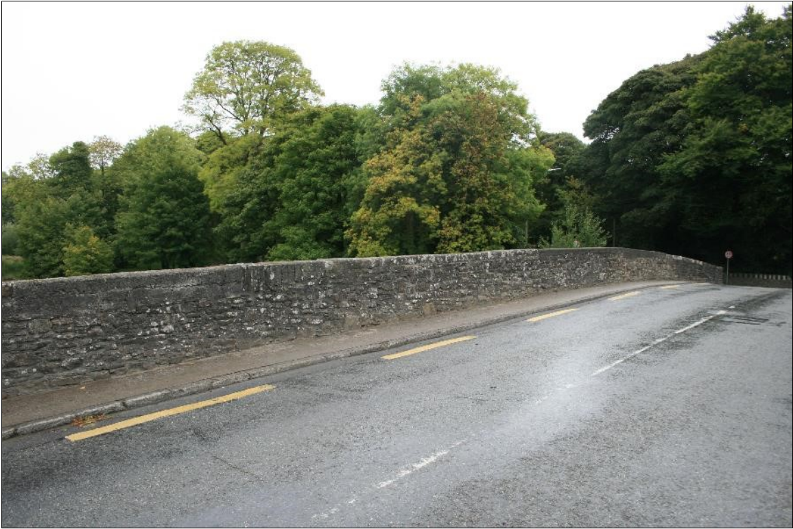
Plate 3: Detail of interior of north parapet wall
