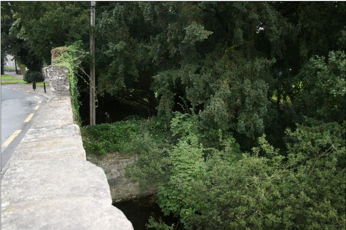
Plate 9: West abutment from north parapet.
