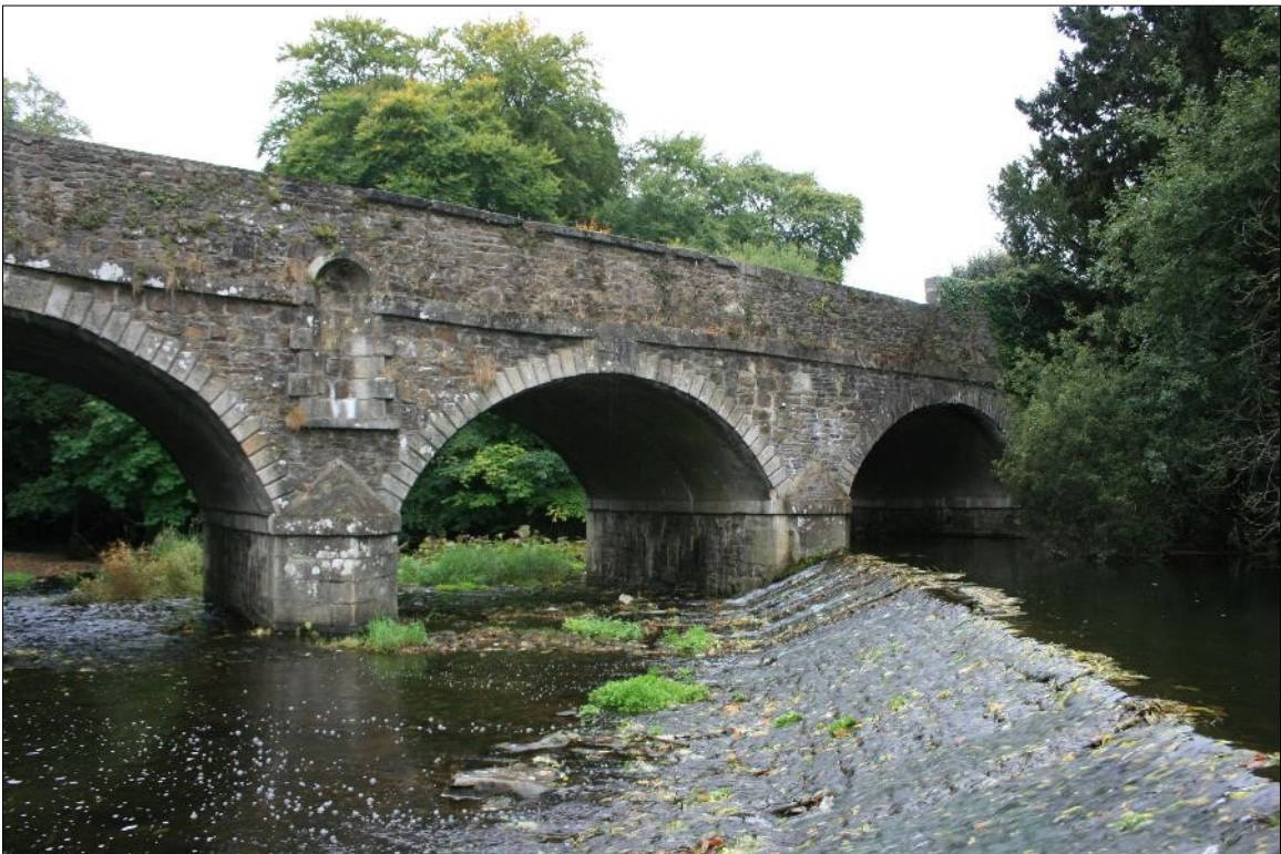
Plate 11: West half of north elevation with stone weir in foreground.
