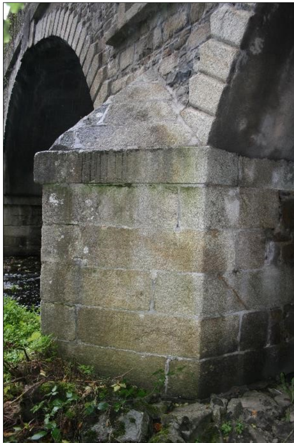
Plate 22: Detail of downstream cutwater on south elevation
