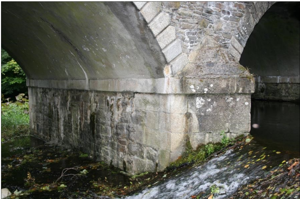
Plate 16: Pier closest to west abutment. Weir in foreground
