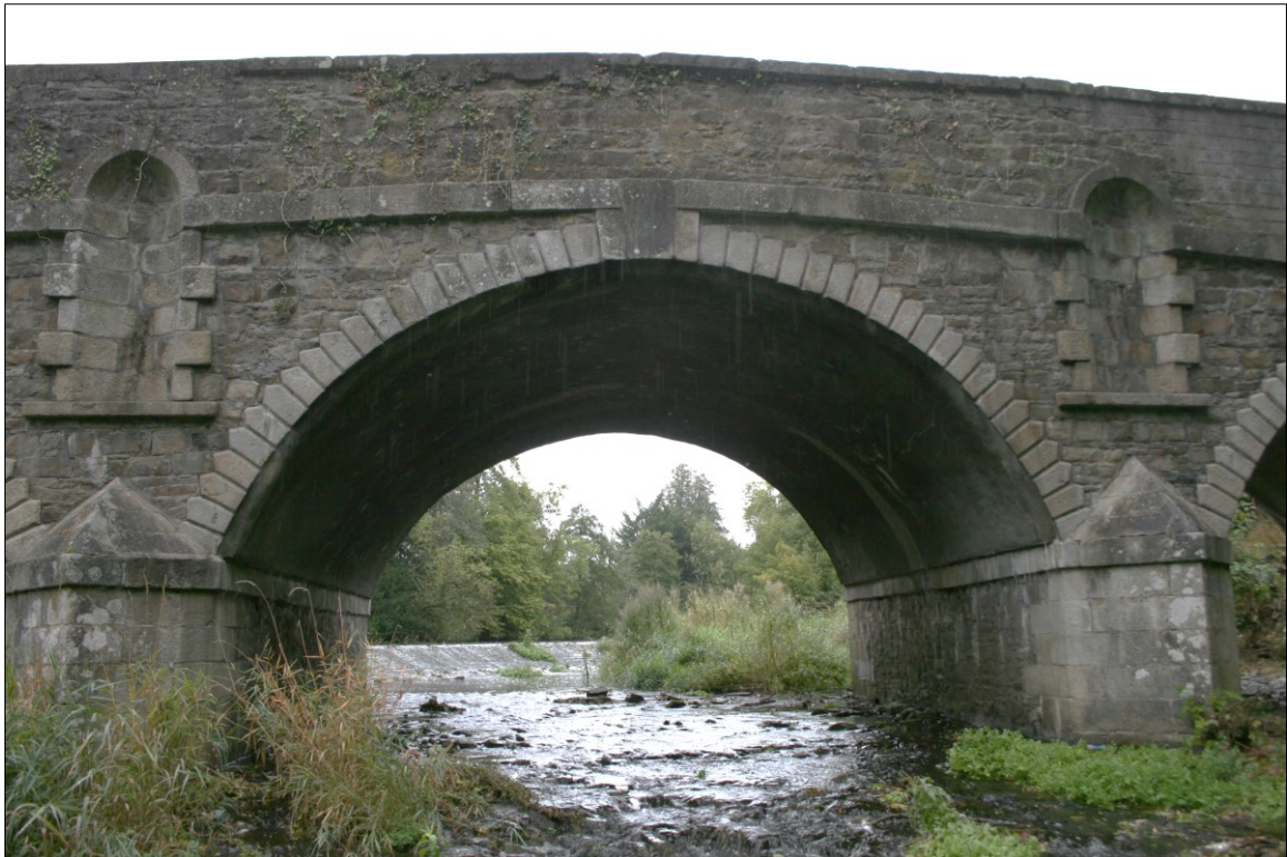
Plate 20: South elevation of central archway
