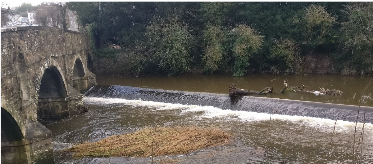
Figure 7-1: Debris located at the Weir from a Flood Event in December 2018
