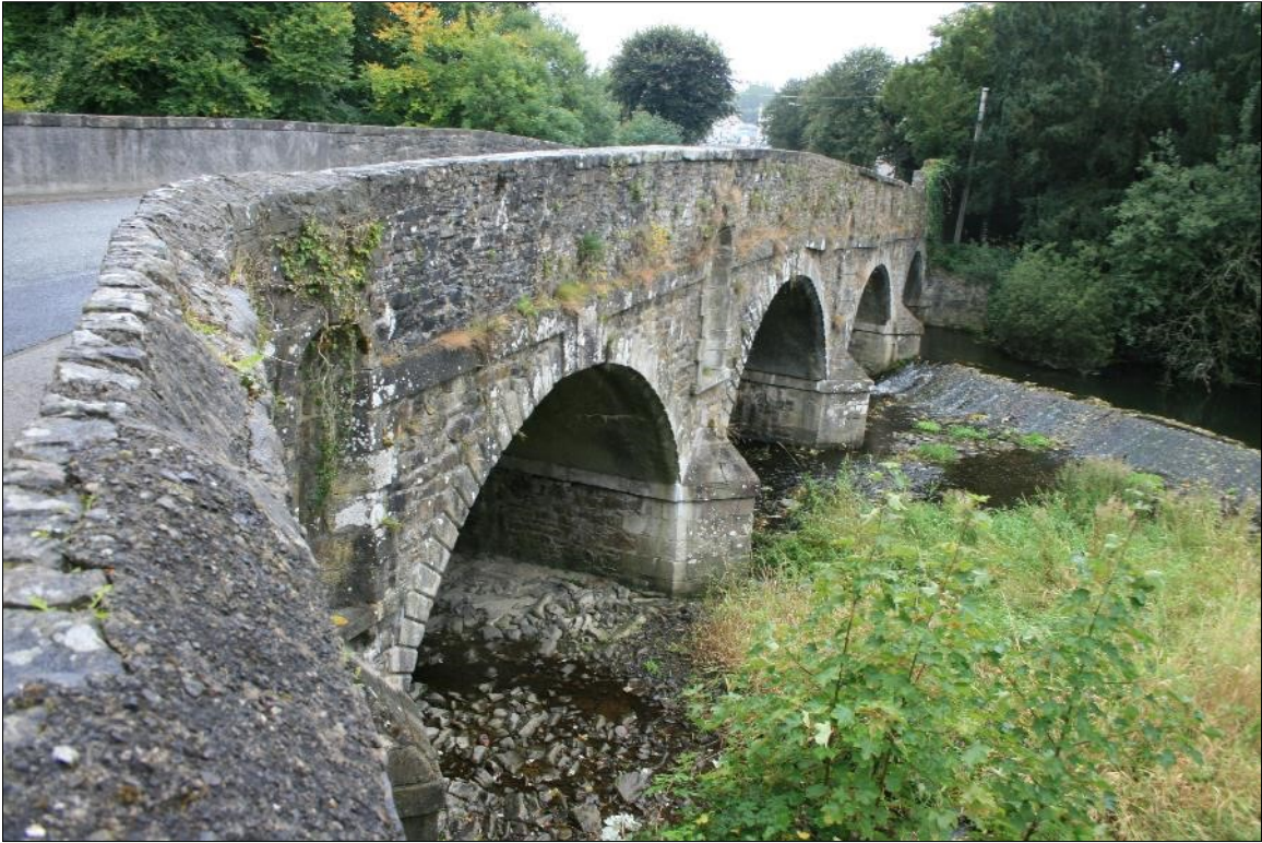
Plate 8: View along north elevation from north parapet at east end
