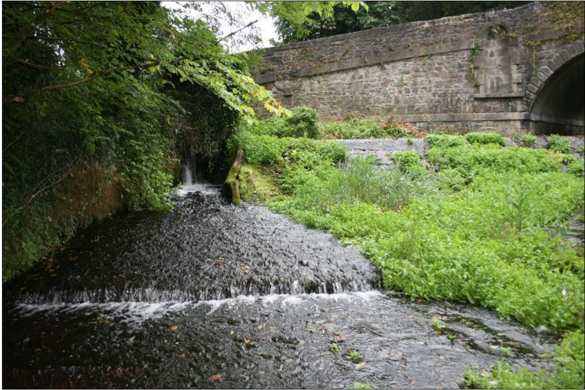
Plate 19: Sluice at west end of south downstream side of bridge.
