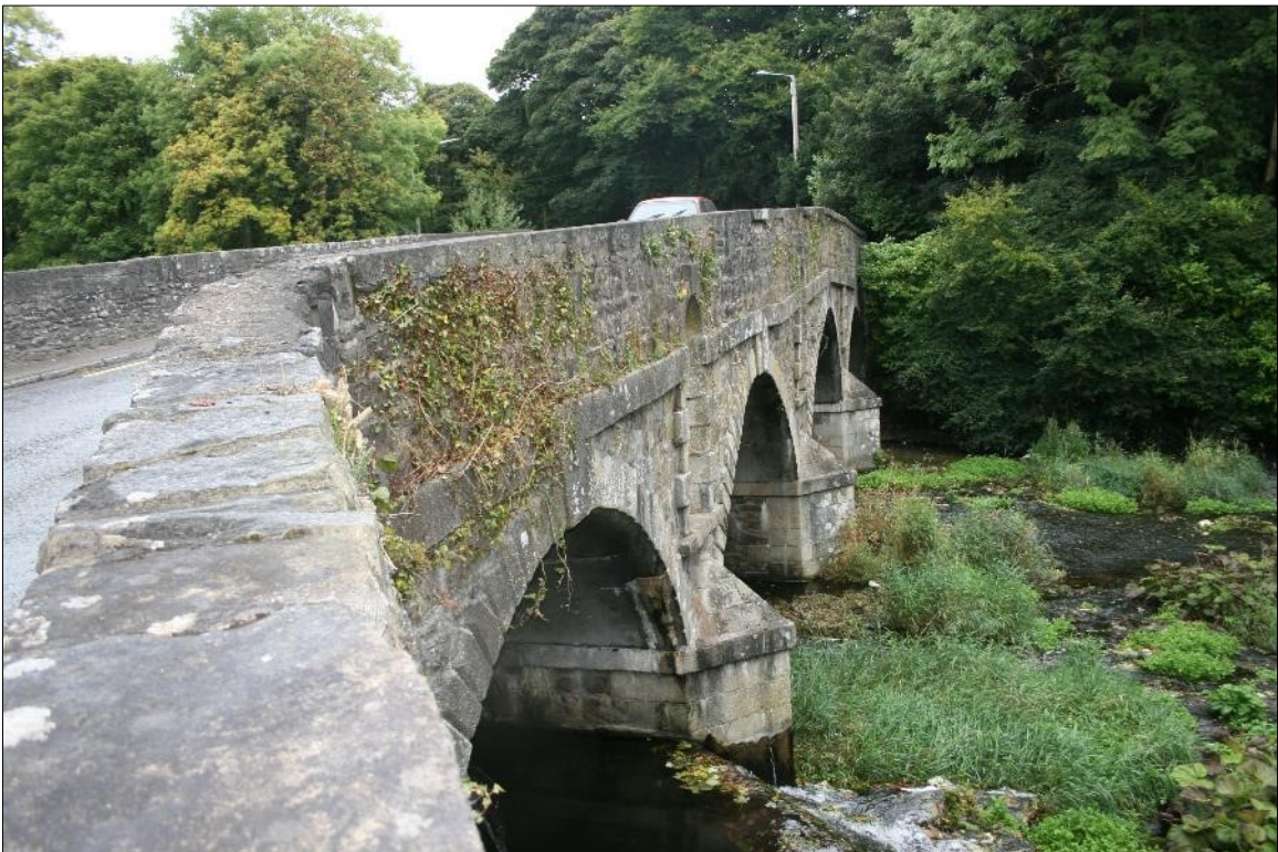
Plate 6: View along south elevation from south parapet at west end.
