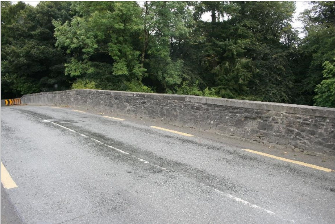
Plate 4: Detail of interior of south parapet wall
