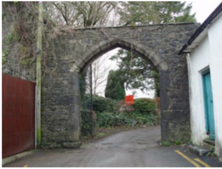
Plate 39. Gate arch at Barrack Lane, three phases of construction evident.
