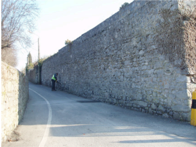
Plate 14. Western end of boundary wall to Evans Home,
