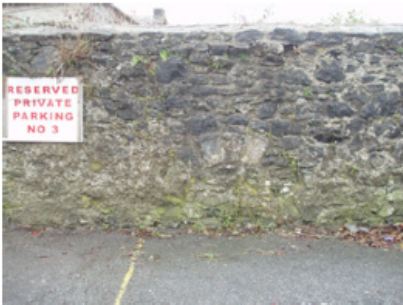
Plate 43. Blocked round headed arch in exterior of east boundary wall.
