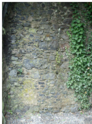
Plate 28. Detail of masonry, int north wall.
