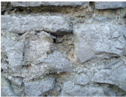
Plate 12. Render of 19th century wall F14 with distinctive pebbles, and later repointing. Many chipped faced stones used.
