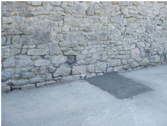
Plate 4. Location of trench at wall F12, note coursed rectangular blocks.
