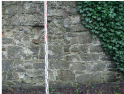
Plate 30. Red brick infill/ repair of boundary wall.
