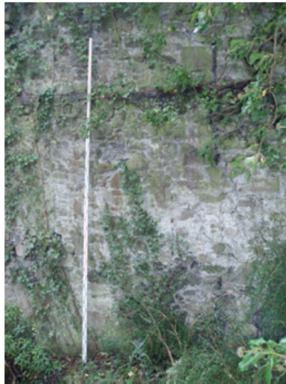
Plate 37. Internal end wall of building on Rocque, south west boundary. Scar of possible stairwell in wall.
