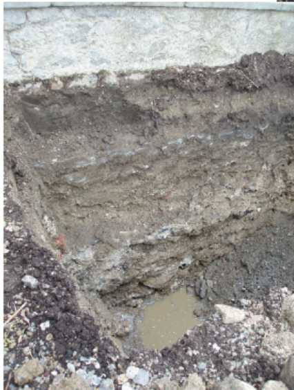
Plate 16. Trial pit 6, wall of Evans Home on 2 plinths.
