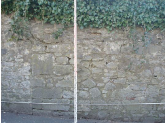
Plate 6. Large dressed quoins of Barracks, boundary wall abuts.
