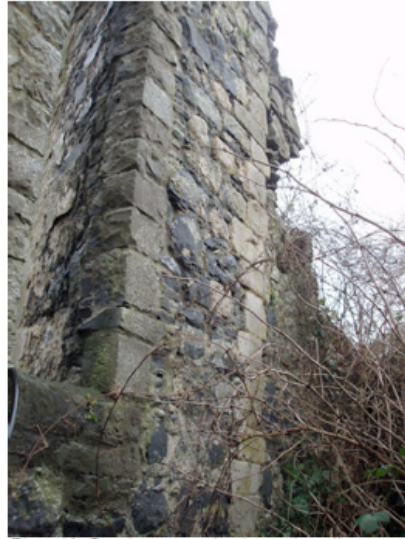
Plate 40. Sandstone quoins in north wall at south end of chancel.
