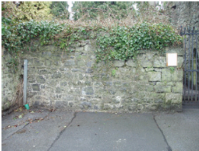
Plate 20. Wall at stepped entrance to site at west.
