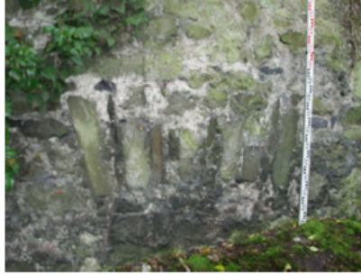
Plate 35. Voussoirs of arch over blocked opening 4.
