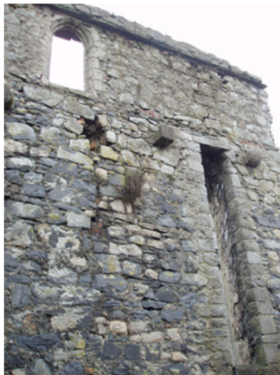
Plate 41. Patched wall of chancel, where it forms site boundary. Upper levels appear intact.
