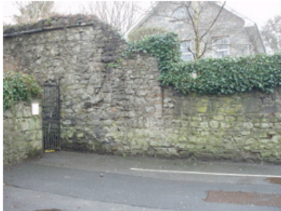
Plate 22. North wall claustral building, with added masonry to west, with brick dressed window.
