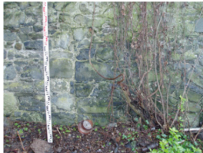
Plate 32. Join/ abutment of walls, west boundary wall.
