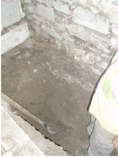
Plate 11. Trial pit 1, shovel at base of wall.
