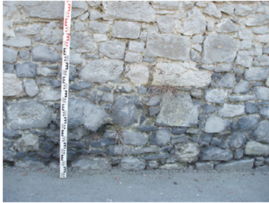
Plate 11. Lower courses of boundary wall, weathered black calciferous limestone with few trace of render extant.
