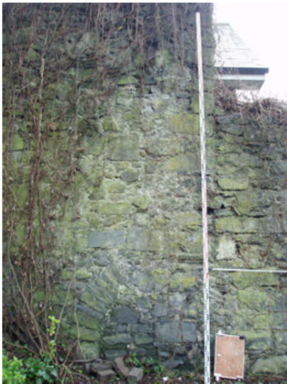
Plate 31. Blocked arch, cut /abuted by later wall.
