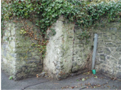
Plate 19. Untied walls at boundary at millrace.
