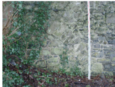
Plate 33. Blocked arch C, west boundary.
