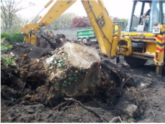
Plate 6. Removal of tree roots.
