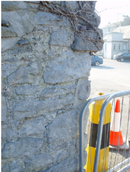
Plate 15. Projecting stones , possibly part of bridge parapet, with iron hinge pivot.
