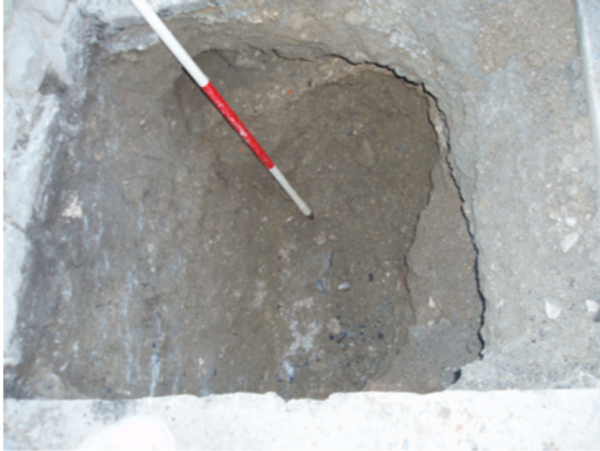
Plate 3. Wall F12 sits on earlier masonry which projects from the base of the wall. Depth 1.32m below street level. Red brick rubble abuts lower face of wall F12.
