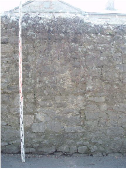
Plate 8. infilled ope in gable wall of barracks.
