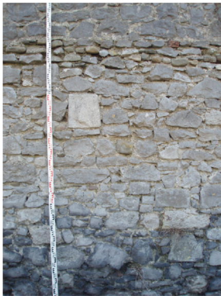
Plate 13. Levels of rebuilding, with reused stone from abbey.
