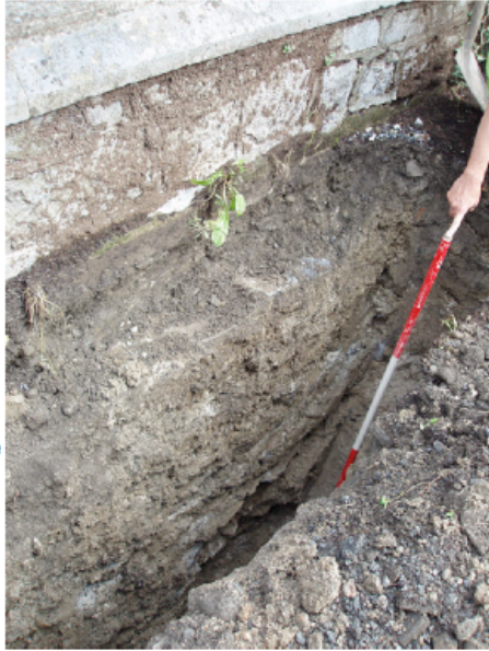
Plate 17. Trial pit 7, wall of Evans Home on plinth footing.
