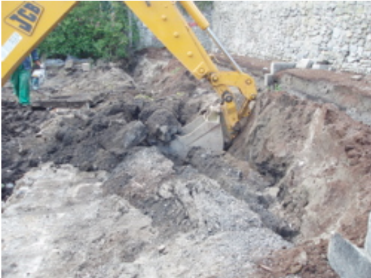
Plate 1. Removal of foundations.
