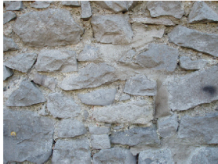
Plate 16. Chipped stone face of 19th century wall.
