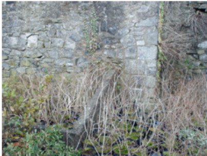
Plate 42. Round headed arch in late 18th or 19th century east site boundary wall.
