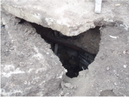
Plate 2. Well, covered by floorslab of greenhouse.
