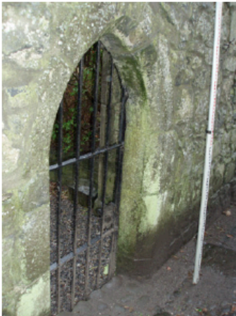
Plate 21. North door, ext, to claustral building.
