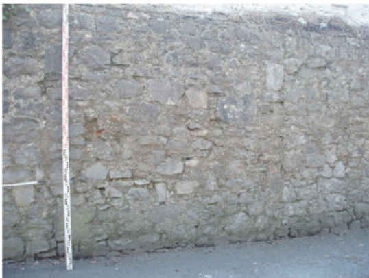
Plate 7. Barracks gable wall with infilled opes.
