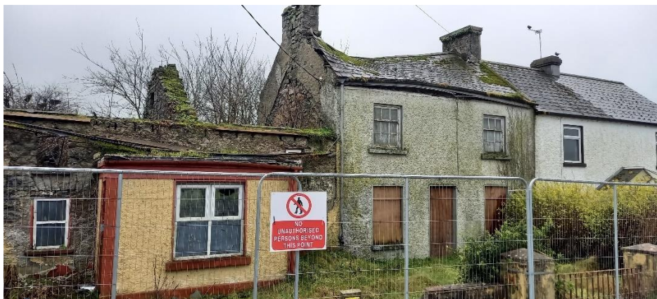
Pair of derelict houses to be demolished & replaced Site No.2
