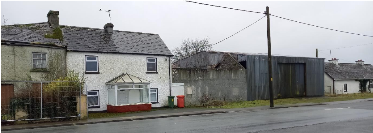
Existing buildings to be demolished and replaced Sites 1, 2 & 3
