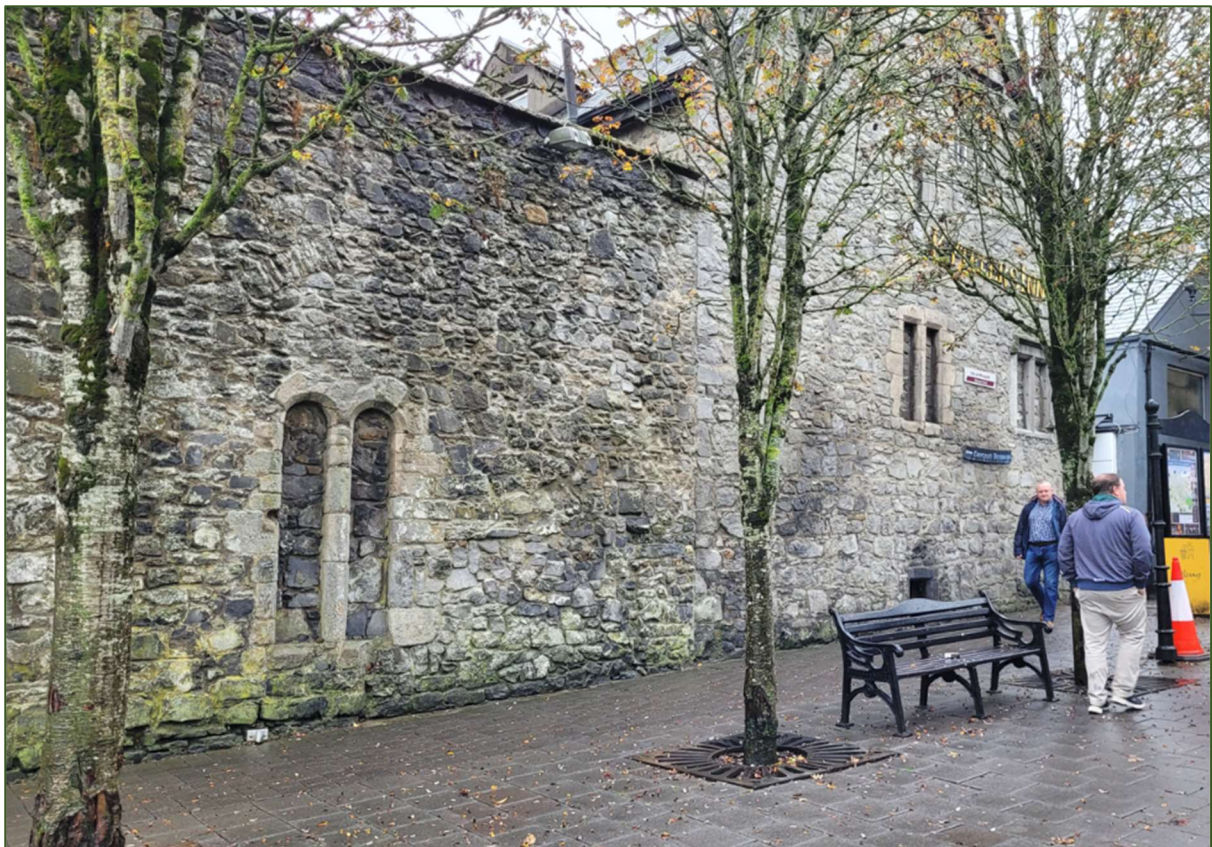
Plate 3 North facing gable elevation of Kyteler's Inn showing windows and opes.
