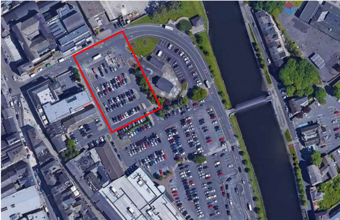
Figure 7 - Market Yard Car Park
